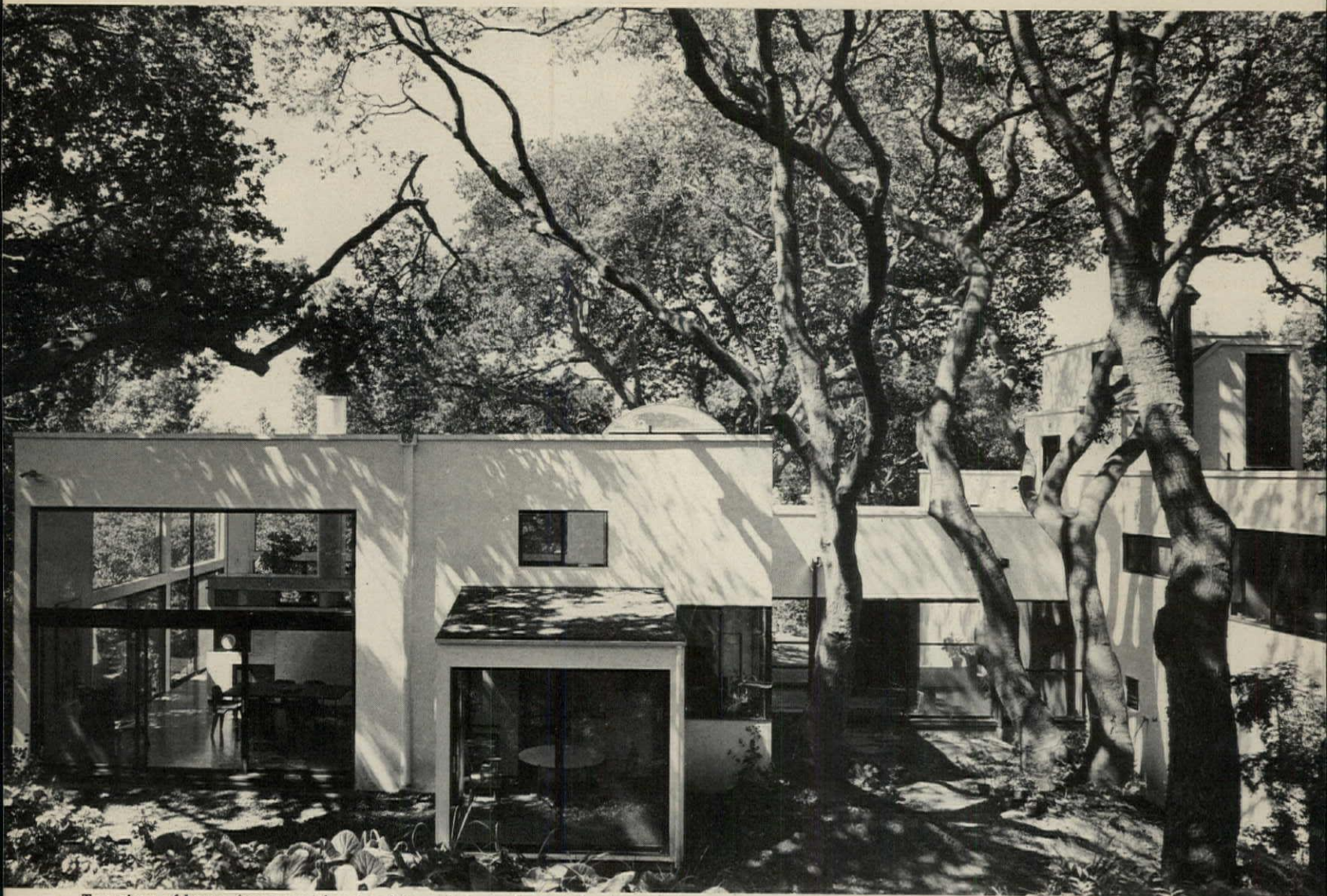
Two views of house—from rear ( above ) and front ( below )—show results of careful siting, planning, and engineering to save old oak trees. Shallow grade beams were used, for example, to avoid severing of tree roots.
