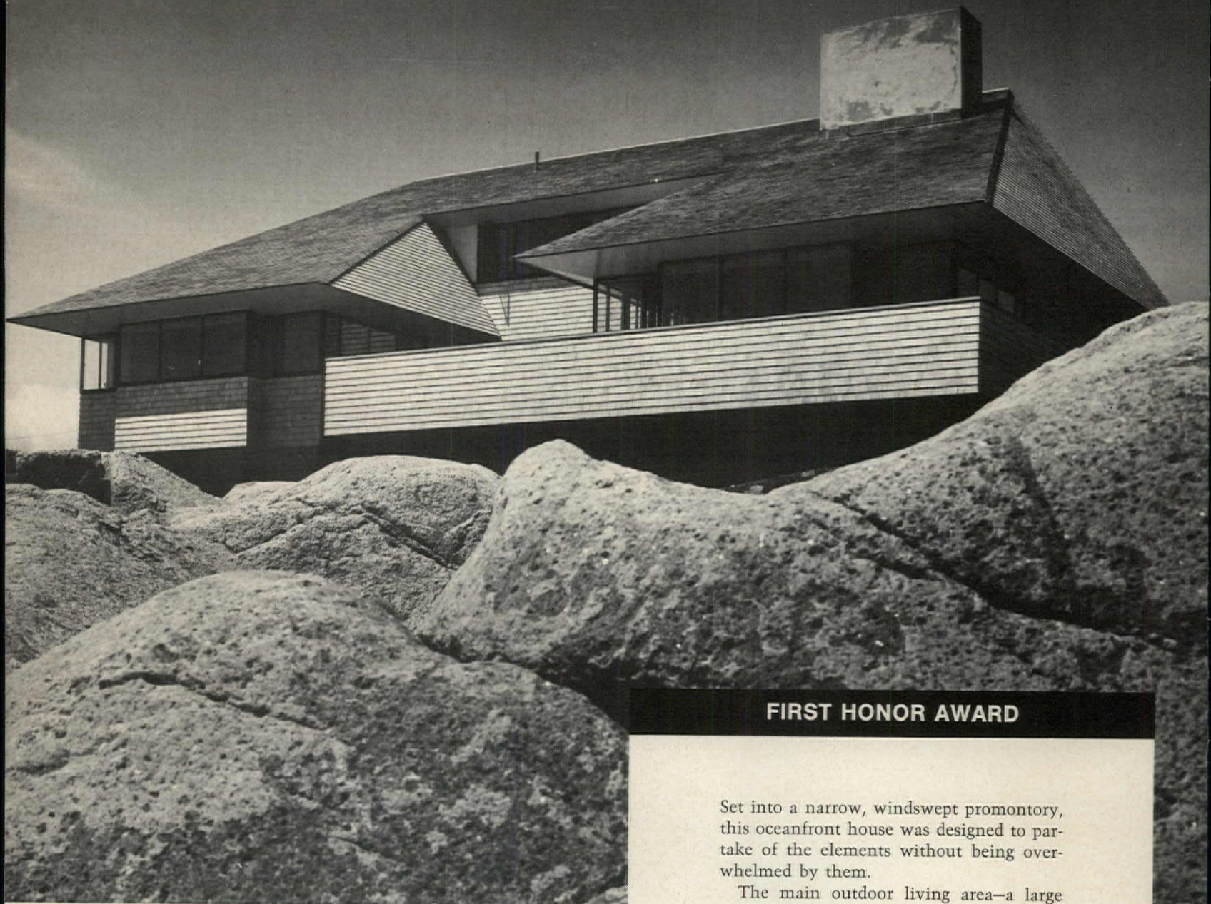
Rear of house cantilevers out toward ocean view, and front is dug into cliff (section, below). Master bedroom wing is at left, living room wing at right.
