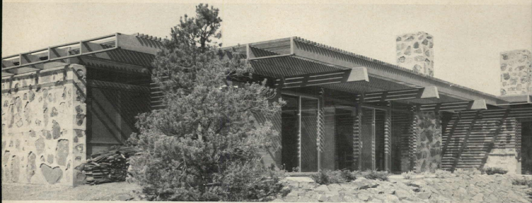
Roof framing is extended 8' and topped by latticework to create deep sunshade around house. Above: guest quarters at left and living room at right. Below:
