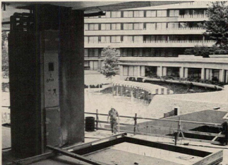
Vertical unit fits up next to column, allowing use of floor-to-ceiling glass walls. Units were designed for the Watergate in Washington, D.C., rear.
