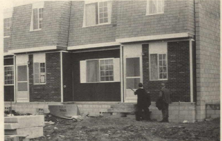
Stacked units are bolted together. The modules form mansarded townhouses.
