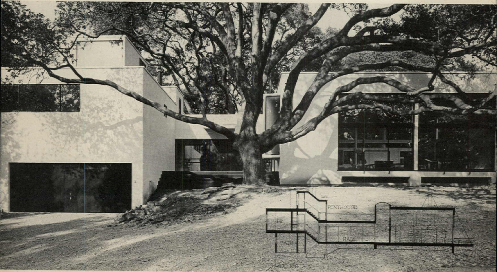
Two views of house—from rear ( above ) and front ( below )—show results of careful siting, planning, and engineering to save old oak trees. Shallow grade beams were used, for example, to avoid severing of tree roots.
