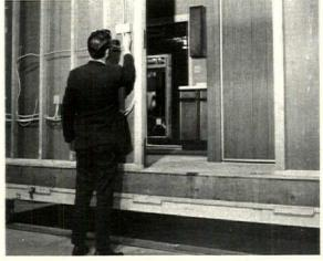
... and work is immediately checked on assembly line by an insurance company's inspector.
