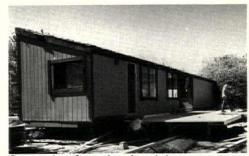
Construction photos show box sitting on temporary foundations of screw jacks (above). Running gear is permanent on these models, but on most houses it is removable. Unfinished interior (below) shows abutting ridges and posts ready to be bolted together and cased.
