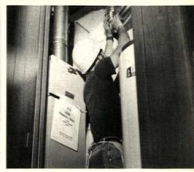
and hot water heater. The furnace and heater are placed behind a sliding panel to facilitate on-site inspection.
