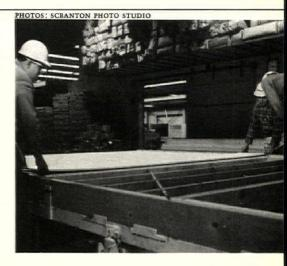
Ceiling panel is built on a jig . . .
