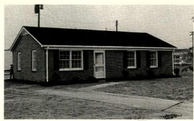
Alternate version (above and right) is slightly wider and has a full dining room, but lacks an entrance foyer and forces all traffic through the living room. Brick exteriors and durable materials are used to keep future maintenance costs to a minimum. Home has three bedrooms.
