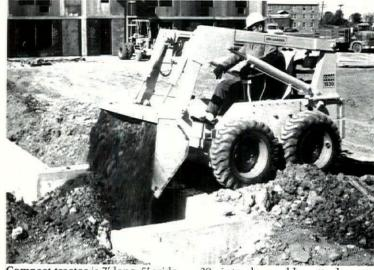
Compact tractor is 7' long, 5' wide, and 5' high. The four-wheel-drive unit can turn a tight circle in its own tracks. It lifts up to 1,500 lbs., weighs two tons. Three models-26hp, 30hp, and 37hp-have about
