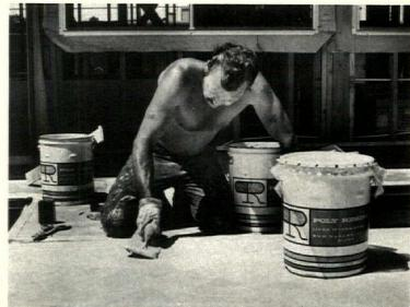
Polyurethane skin is both a seamless waterproof roof coating and a durable deck. It covers concrete (foreground) or plywood (background). Consistency for spraying, rolling, brushing, or spreading, varies with amount of silica thickener (by Cabot, Boston) added. Poly Resins, Sun Valley, Calif. CIRCLE 218 ON READER SERVICE CARD
