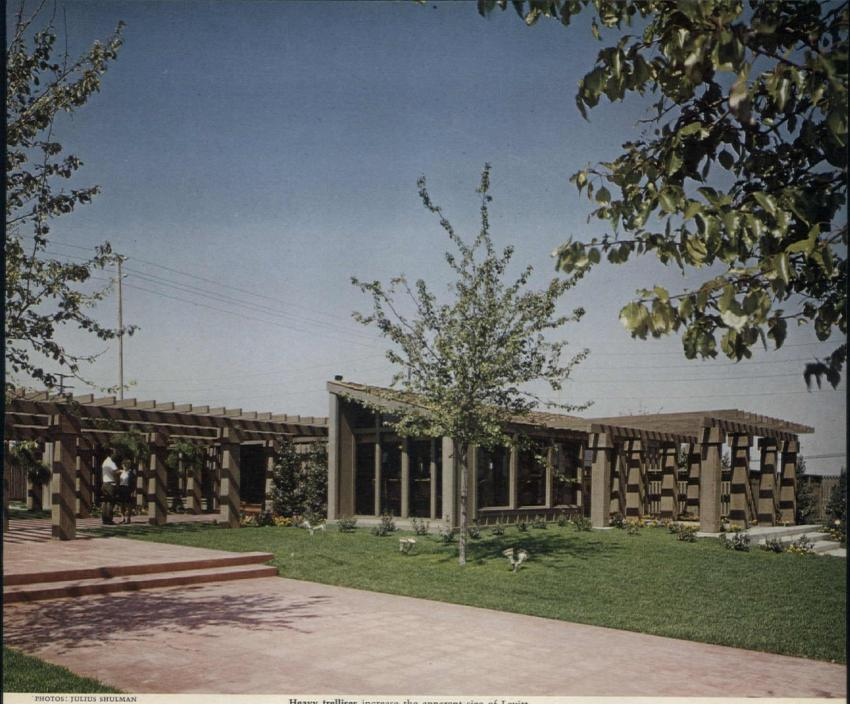
Heavy trellises increase the apparent size of Levitt & Son's sales office and help mask the boxiness of the modules. Buildings are made with shear panels and box beams to allow for large expanses of glass wall-unusual in a modular.
