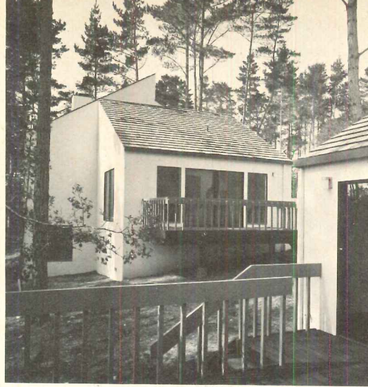
VIEW FROM DECK is of adjoining house. Deed restrictions require at least 20 feet between houses and limit density to four houses per acre.
