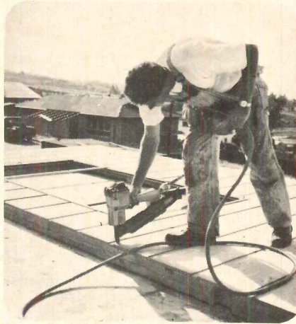
Fast on-site component construction with CN-137
