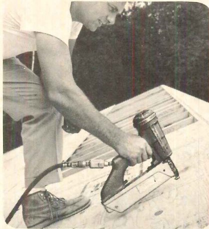
Staple Nailer anchors down plywood roof deck
