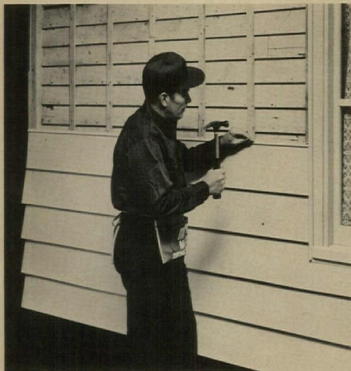
Solid vinyl clapboards , 4" or 8" (shown), can be applied over masonry or wood in remodeling. Color-impregnated material needs no paint, won't dent, peel or flake. Sample kit available. Mastic, South Bend, Ind. Circle 224 on Reader Service card
