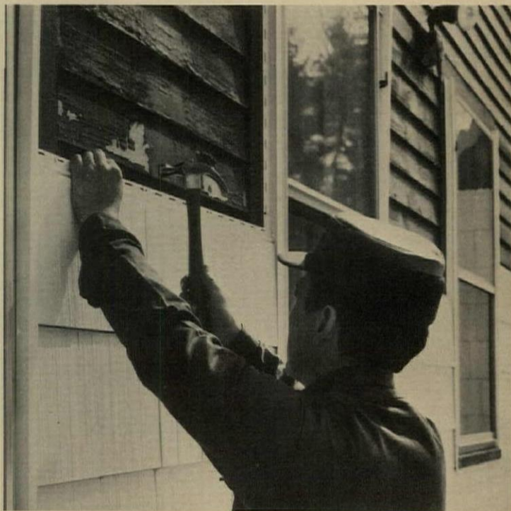
Shake-like siding resembles hand-split wood but is solid vinyl so it doesn't need paint, and it won't rot, chip, peel, blister or dent. Panels 11" x 38" lock together neatly and install easily with prepunched nailing holes. Bird & Son, East Walpole, Mass.
