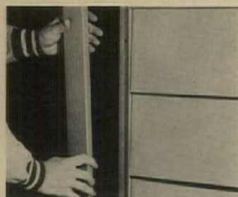
Snap-on corner comes in two pieces of formed aluminum. The first piece is nailed to corner and siding is installed. Then, the second piece snaps on over flanges of first piece to cover panel ends. No caulking is needed. Also, Akron, Ohio.
