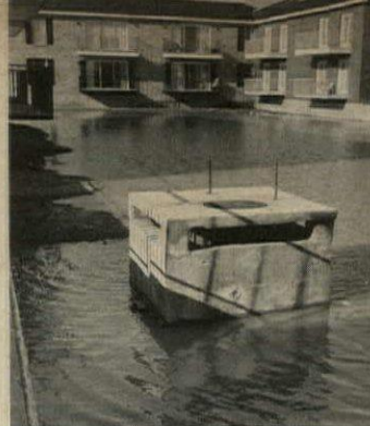
OVERFLOW BOX , designed to handle anticipated rainfall, also contains drain valve so lake level can be lowered for cleaning.
