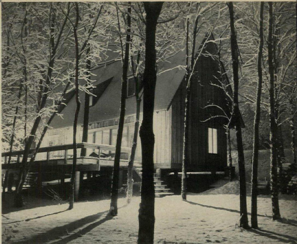
RAISED FOUNDATION (above and bottom) gives ample clearance against high spring-flood waters.
