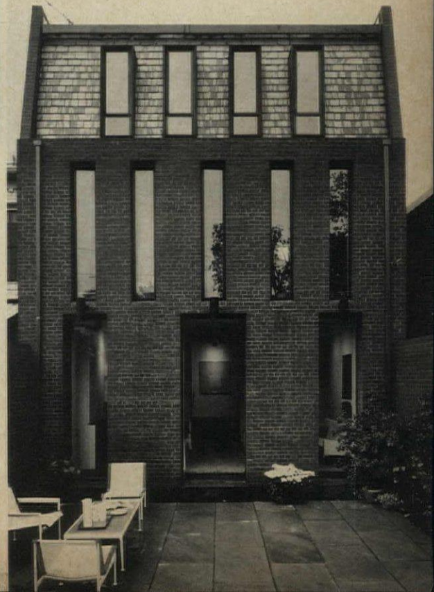
GARDEN ELEVATION ( below ) shows variety of fenestration on three levels. All windows are ceiling height and recessed in wall.
