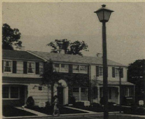
Hercules Light Riser ® laminated lighting standards used for street lighting, Town House Development, Willingboro, New Jersey. Public Service Electric and Gas Co.
