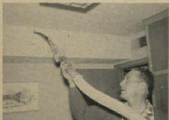
Acoustical insulation is a cellulose loose fill that controls noise as well as temperature. The lightweight material can be blown into wall and ceiling cavities through holes as small as 1" in diameter. Hagan Mfg., Delphos, Ohio.
