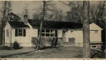
**Siding** is weatherproof insulation board surfaced with Tedlar film that requires no painting. Choice of clapboard or board-and-batten in a satinwhite finish. Clapboards are 12' long. Homasote, Trenton, N.J. Circle 228 on Reader Service card
