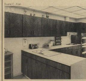
Soffits above the counters allow this kitchen to use a regular cabinet system under a very irregular, high roof. Working lights are set into the bottom of the soffit. The pie-shaped opening at the rear of the kitchen leads to an unusual type of side window (plan below). Architect: Ulrich Franzen.
