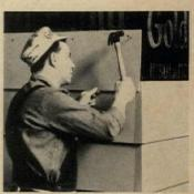
**Mineral-fiber siding** has a concealed nailing system that does away with adhesive, splines or slots. Nailing can be done  $1\frac{1}{2}$ " from the edge without splitting. Six colors: gold, green, red, gray, yellow and white. National Gypsum, Buffalo, N.Y. *Circle 230 on Reader Service card*
