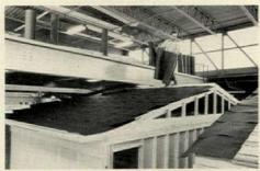
**ROOFING** is 240-lb. asphalt shingles over double layer of 15-lb. asphalt-impregnated felt. Overlapping felt provides for joining modules at site.
