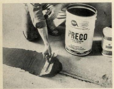
**Concrete resurfacing** bonds securely to worn floors, can be used to fill ruts, smooth rough surfaces, bed ceramic tile and serve as an underlayment for resilient flooring. Compound is self-curing and comes in grey and red. Preco, Plainview, N.Y. Circle 210 on Reader Service card
