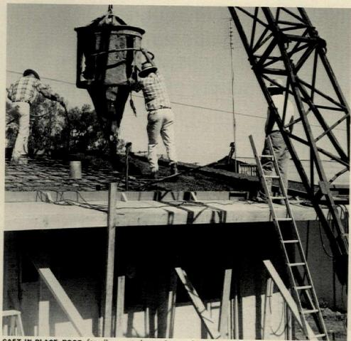
CAST-IN-PLACE ROOF for all-concrete house ties together tilt-up walls by means of overlapping reinforcing bars (see also drawing at upper right). Roof pour for 768-sq.ft. house takes three hours.
