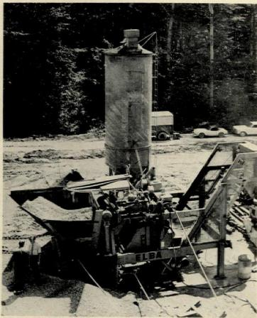
**SELF-CONTAINED PLANT** makes 45 cu. yds. of concrete per hour. Components include aggregates bin, left; cement silo, rear; concrete hopper, right.
