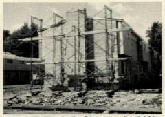
**BRICK VENEER** is the biggest on-site finishing job. It compensates for its extra cost by giving the appearance of conventional construction.
