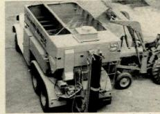
STORAGE COMPARTMENTS for sand and aggregates are loaded from top. Cement and water are kept in sealed tanks. Materials are proportioned, mixed and metered from central control panel (below) at rear of truck.
