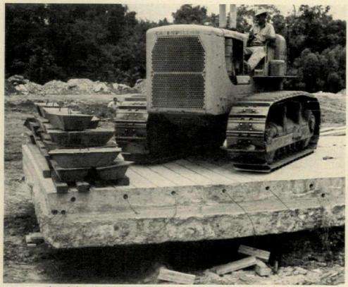
LOAD TEST showed that 15' of undercut house slab could support 123,000 lbs. after post-tensioning.
