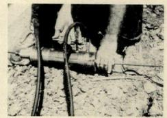
HYDRAULIC JACK pulls tendon to specified final tension by ramming anchor chuck into place.
