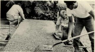
Colorful aggregate of uniform size (%- to %-inch on this job) is seeded from shovel. In background two finishers have already begun tamping in aggregate with wooden hand floats.
