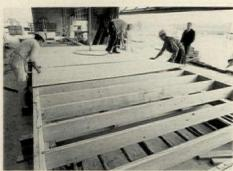
**FLOOR DECK** is sheathed after being assembled upside-down to assure precise joist alignment. Glue-nail fastening guarantees structural rigidity.
