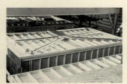
**DUCTWORK** for individual heating and cooling systems is fabricated in place from 5"-diameter tubing after first-floor ceiling has been attached.
