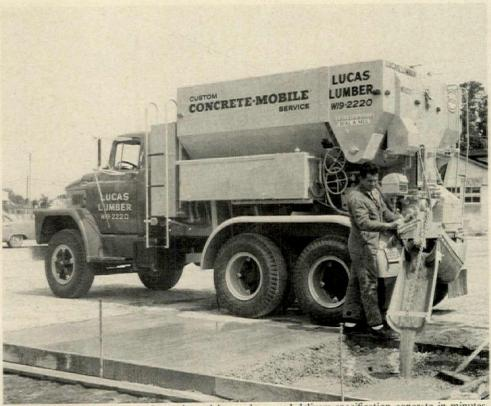
TRUCK-MOUNTED MIXER-a 6-cu.-yd. model-produces and delivers specification concrete in minutes
