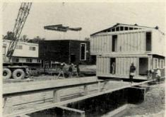
**FIRST-FLOOR MODULE** is lowered into place on masonry block foundation; longitudinal I-beam supports the 25'-long unit at its center.
