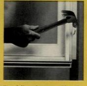
The full perimeter nailing fin on the double-hung Ultra Supreme Window (U.S.A.) reduces installation time by over an hour. Pop the U.S.A. in place, drive in the nails . . . it's in.
