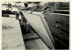
**CEILING UNIT** is turned over after being fabricated upside-down on platform above assembly line. Unit is then lowered onto module.
