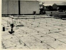
**SHEATHED TENDONS** are lightly tensioned and set on chair supports before slab is poured.
