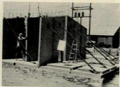
TILT-UP WALLS are braced (photo) before poured roof and apron anchor them (drawing).
