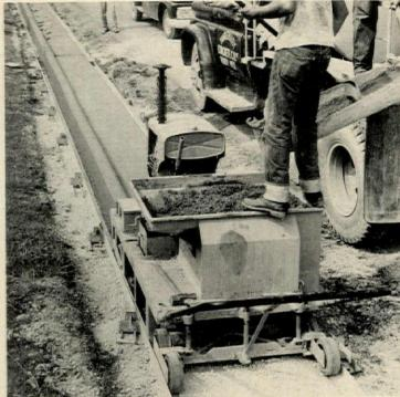
**CONCRETE EXTRUDERS** form curbs (*left*) and integral curb/gutters (*above*) at speeds of up to 35' per minute. Concrete mix should be free from slump.
