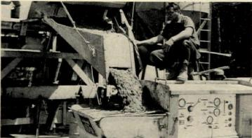
CONCRETE PUMP of 60-cu.-yd.-per-hr. capacity receives concrete from mixing-plant chute and conveys it directly to formwork a short distance away.
