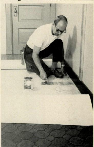
One-component adhesive allows perimeter bonding of sheet-vinyl flooring directly to existing resilient flooring. Quick setup time lets installer apply new flooring 15 to 20 minutes after adhesive is spread. Armstrong Cork, Lancaster, Pa. Circle 204 on Reader Service card
