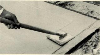
5. An edging tool is then used to secure the aggregate at the edges. This is final step before concrete sets up enough to begin the hosing and brushing operations.
