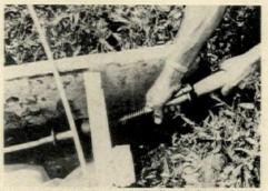
**CENTER-HOLE HAMMER** locks steel-strand tendon by compressing spring in tensioning anchor.
