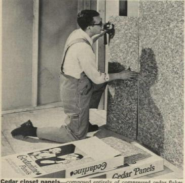
Cedar closet panels—composed entirely of compressed cedar flakes—are easy to install. Panels can be cut to fit, nail directly to studs or over existing walls, need no finishing. They are ½" thick. Giles & Kendall, Huntsville, Ala. Circle 221 on Reader Service card
