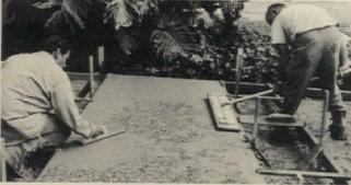
As aggregate embedment is completed along the edges one finisher uses a wood bull float to cover the center. Floating is continued until all aggregate is completely embedded.
