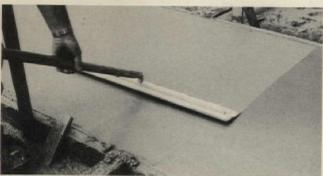
After screeding and tamping, the surface is smoothed with wooden floats. Final smoothing is done with this bull float. The surface is then ready for the aggregate to be seeded.
