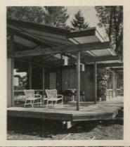
**REAR DECK** (below) is cantilevered. One end (right) is set into corner of house and carpeted to form outdoor extension of family room.
