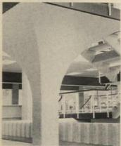
Exposed-aggregate matrix bonds with five times the strength of concrete, sets fast to prevent slumping and cures in less than 24 hours. It conforms to any shape and can be applied to interior or exterior walls or columns. Marbleloid, North Bergen, N.J.
