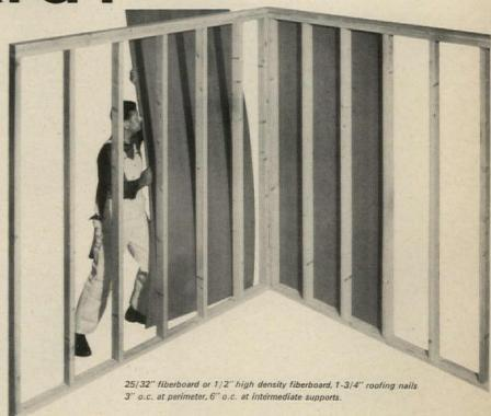
o.c. at perimeter, 8" o.c. at intermediate supports.
