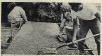
Colorful aggregate of uniform size (¼- to ½-inch on this job) is seeded from shovel. In background two finishers have already begun tamping in aggregate with wooden hand floats.
