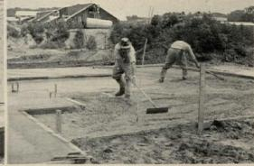
UNDER-SLAB TUBING is installed by two-man crew. First man unrolls a one-house supply—contained in a single coil, which eliminates joints—while
