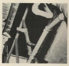
Maximum safety was achieved because torches were not required for installation; this was especially important in confined, "tinder-dry" construction.
