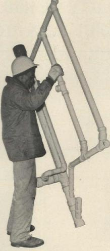
4. PVC pipe is lightweight and easy to install through and around the existing framing. It can readily be preassembled.
