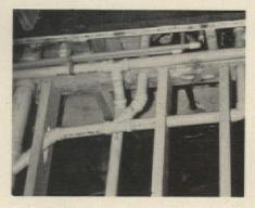
Installation was remarkably easy in tight, hard-to-get-at places because solvent cemented joints eliminated threading and soldering.
