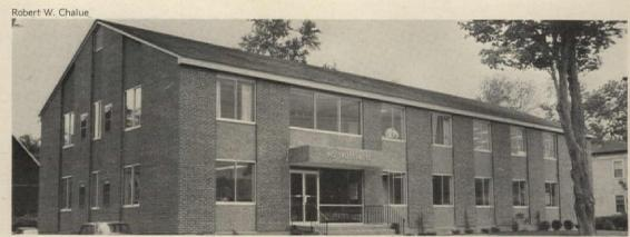
TRUSS-ROOF OFFICE BUILDING with precast floors, brick-veneered block walls and 12,000 rentable sq. ft.
