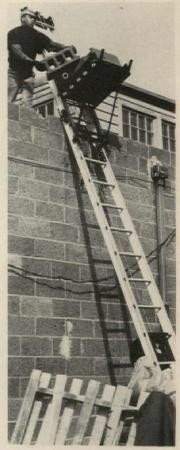
adder-platform hoist is designed to handle brick and block on a flat tray that fits onto the platform. The model shown also has a mortar hopper that can be used in place of the tray. Capacity: 400 lbs. Aeroil Products, South Hackensack, N.J.
