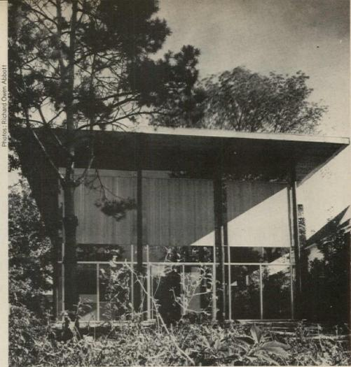
PINE POLES, 10' o.c. and 20' high, frame curtain-walled house. This is the rear elevation.
