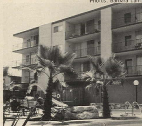
APARTMENT FIX-UP cost about $10,750 a unit.
