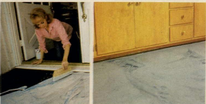
Marble-like seamless flooring can be applied in just one coat—inside or outside—for about 43 cents per sq. ft. Catalyst-activated colorant is lightly mixed into a white base to produce the streaking effect, then the liquid is poured onto subflooring and spread with a wallpaper brush. The surface is ready for use in four hours, requires no further finishing, and resists freezing or heat up to 600°F. Porous subfloors require preliminary sealing with a thin primer coat of the liquid; smooth concrete surfaces must first be etched. Liquid Marble of Luminall Paints, Los Angeles. Circle 295 on Reader Service card
