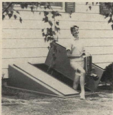
BUILDER: Willard Ryan, Custom Builder LOCATION: Madison, Wisconsin
