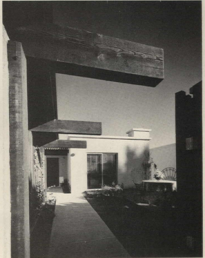
Heavy wood post-and-beam construction ( above, and facing page ) supports the carport roof, and adds to the feeling of early Spanish design. Front walls ( above, left ) are only 6' high to avoid a forbidding streetscape, but side walls are the full 9' height of the house.
