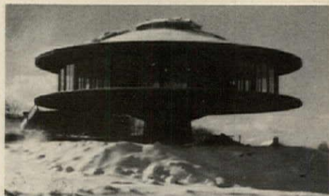
REVOLVING HOUSE is nearing completion on a scenic four-acre site in exurban Wilton, Conn.
