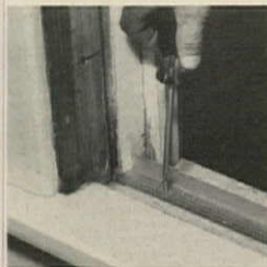
3. Install sill angle
