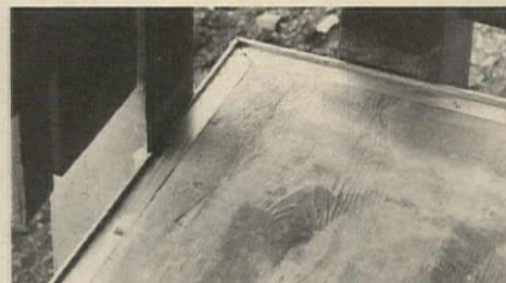
EDGING retains the 1/8" plastic deck topping.
