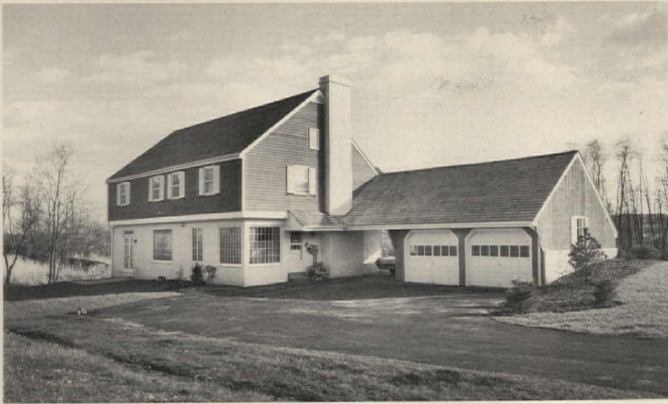
Driveway runs through the porte-cochere to the rear-facing, two-car garage. Normal side entry to garage (plan, bottom) would have required expensive grading of hill on that side of house. Rear-corner location and big windows make breakfast room unusually bright and cheerful.
