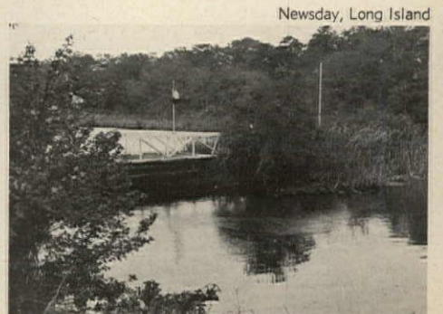
THE BRIDGE that led builder to the bench.
