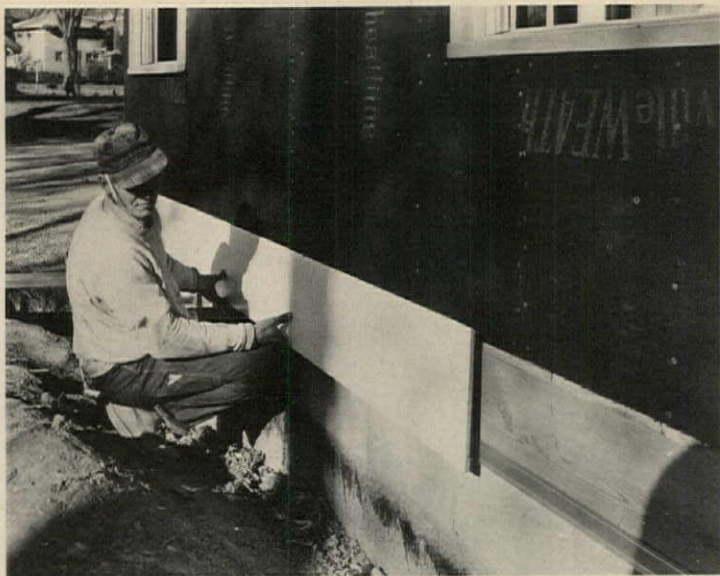
PLASTIC-COATED HARDBOARD —available from a few large producers like Masonite—comes with either vinyl film or thermosetting-plastic face.
