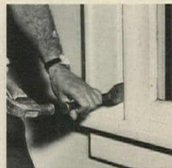
1. Remove sash stops
