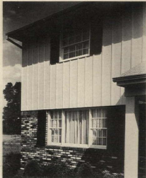
from painting. Above: DuPont's Tedlar on U.S. Plywood's 8" lap and board-and-batten sidings.
