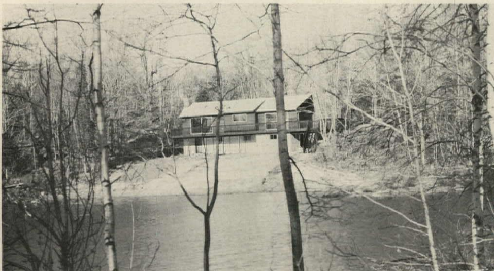
TWO-STORY CLUBHOUSE with locker room and social facilities was built after lake was reclaimed.
