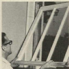
2. Remove old sashes
