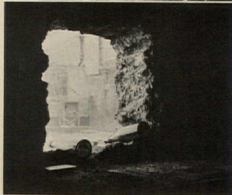
VERSATILE BURNER makes straight cuts and holes in heavy concrete. A 2½" hole ( top right ) can be pierced in 10" reinforced concrete in about two minutes, using up 6' of burning pipe. A 15" x 25" window-size hole ( bottom right ) takes about two hours to burn in 15" concrete.
