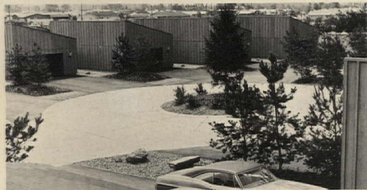
TWO-CAR GARAGES , unusual for Cleveland-area townhouses, face into turn-around. Completely private entrances are recessed at right of each garage.
