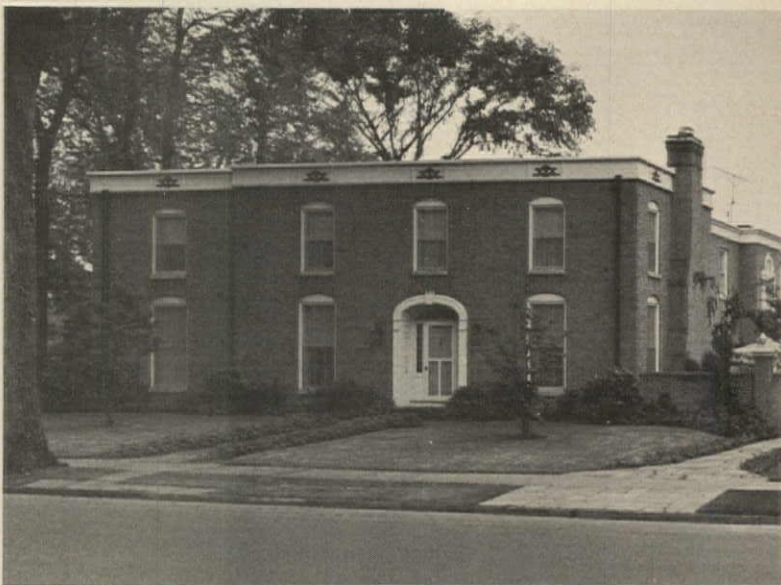
TOWNHOUSES on 190'-wide lot are Perry's most recent job. Units are
