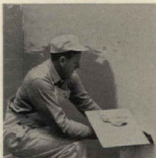
Trowel on Dens-Cote plaster.
