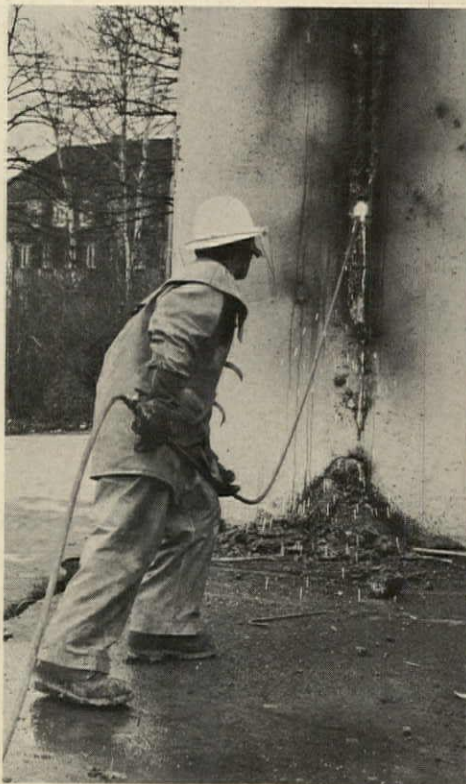
VERSATILE BURNER makes straight cuts and holes in heavy concrete. A 2½" hole ( top right ) can be pierced in 10" reinforced concrete in about two minutes, using up 6' of burning pipe. A 15" x 25" window-size hole ( bottom right ) takes about two hours to burn in 15" concrete.
