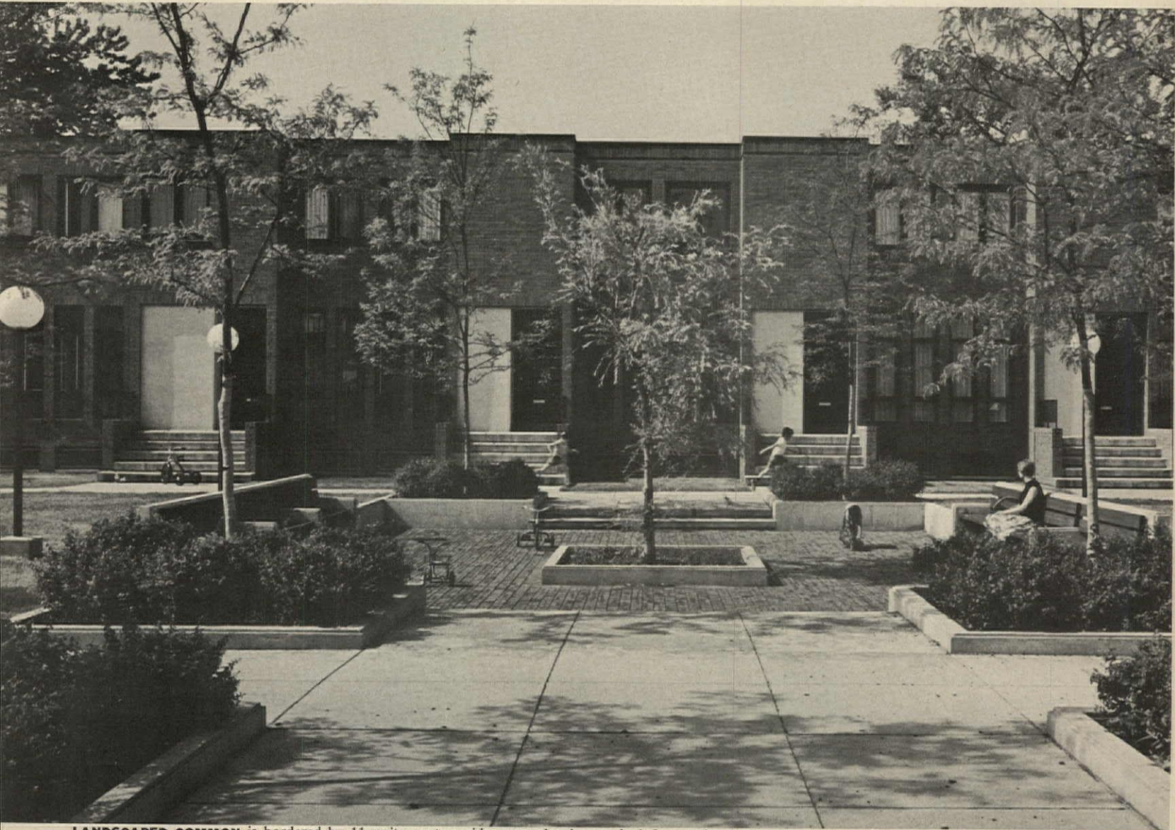
LANDSCAPED COMMON is bordered by 11 units on two sides, can also be reached from other units via private walks at rear of site ( plan, right ).
