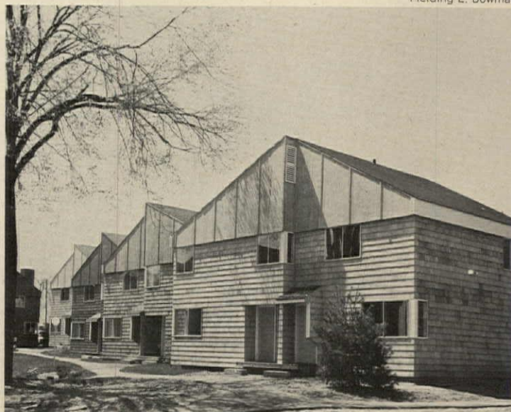
OFFSET FACADES , combined with recessed entries, give extra privacy at front door, add to the impression that each unit is a separate house.
