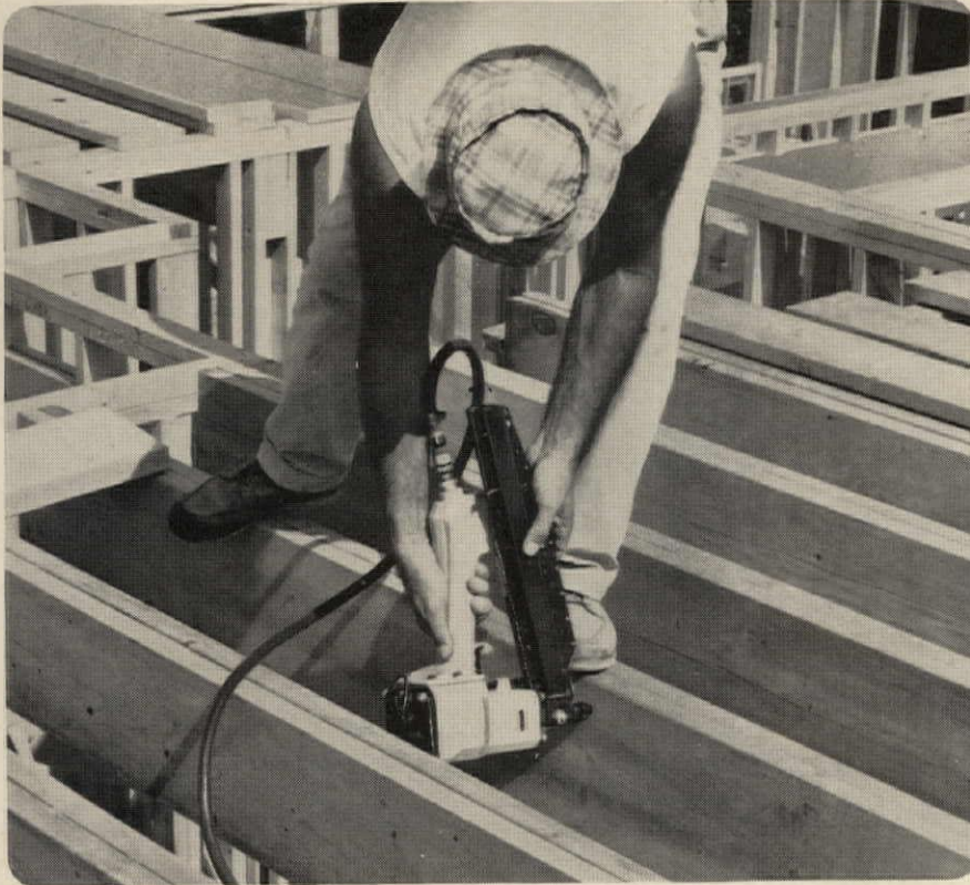
Nailing 1 x 4's to joists.
