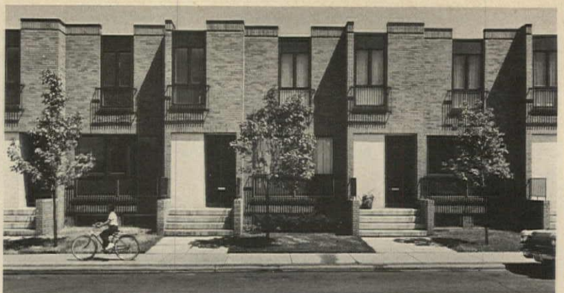
STREET UNITS have recessed windows on both levels for more privacy. Iron railings protect windows. Design retains character of old houses in the neighborhood.
