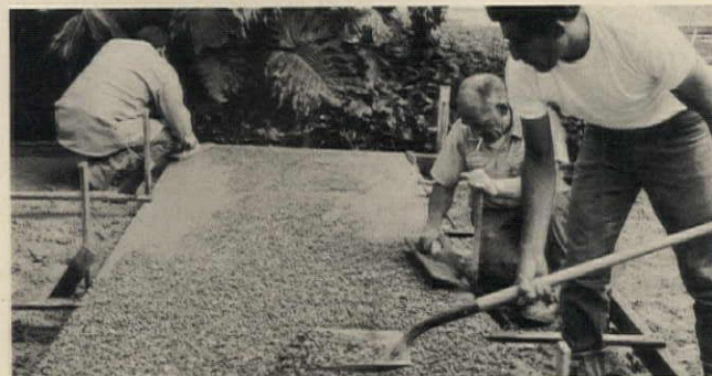
3. Colorful aggregate of uniform size ( \frac{1}{4} - to \frac{1}{2} -inch on this job) is seeded from shovel. In background two finishers have already begun tamping in aggregate with wooden hand floats.
