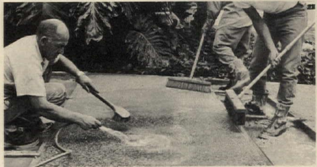
6. Medium-bristle push brooms are used for major brushing. The man with the hose touches up areas missed by the large brooms. This is the final step in producing the exposed aggregate finish.
