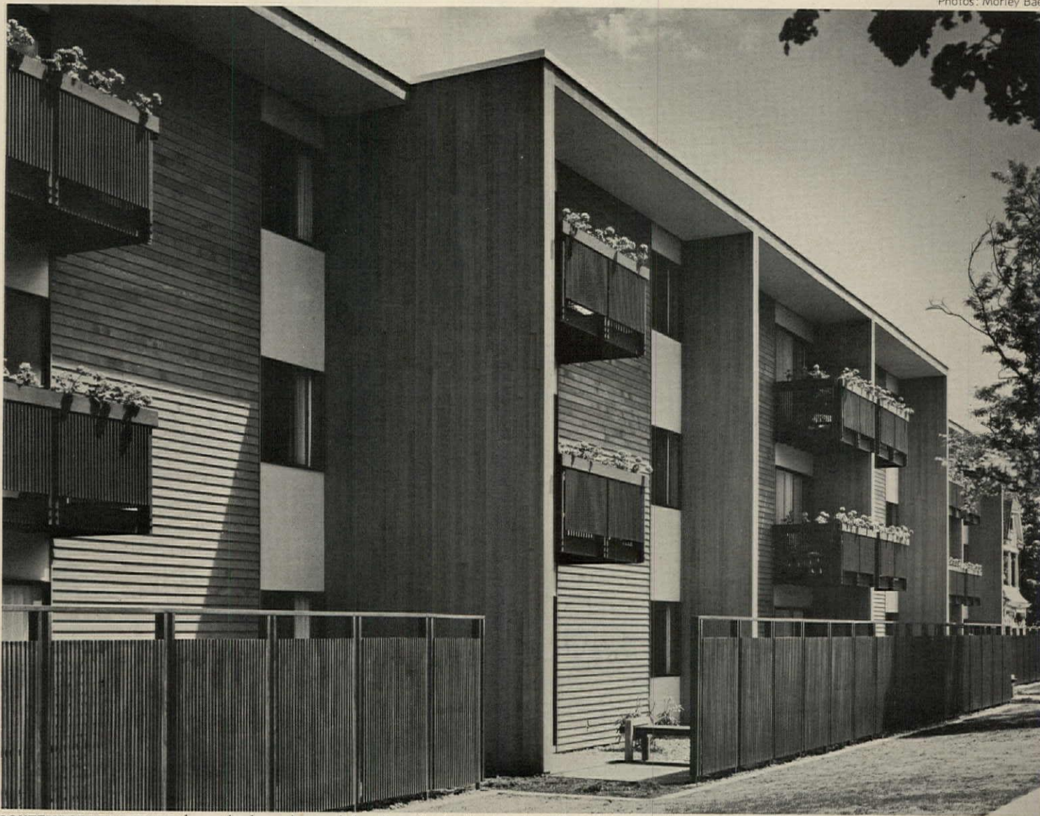
CONTEMPORARY DESIGN has setbacks and extended walls to lend privacy to individual units. Slatted railings screen upper balconies.
