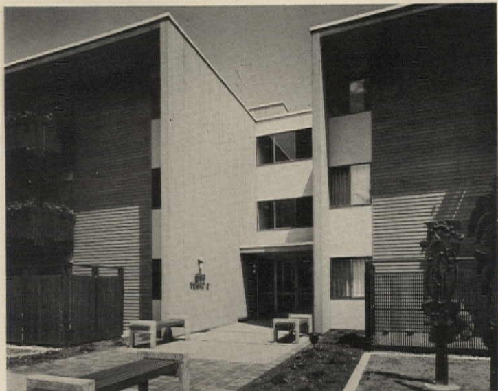
MAIN ENTRANCE on street side of project is set back between units. Doors lead to main lobby, windows above let light into upper lobbies.
