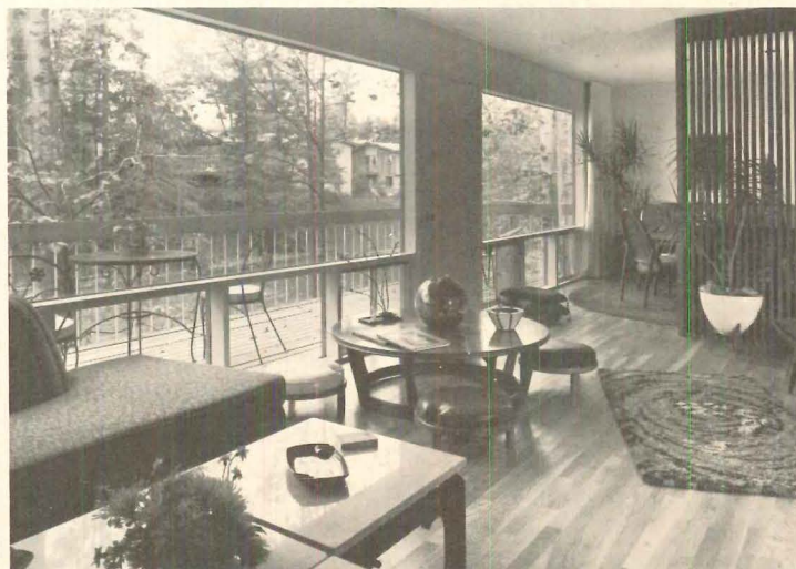
LIVING ROOM and dining area on upper level are partly separated by wood-slat screen. Window wall is fixed glass above sliding sash.
