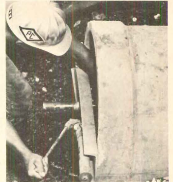
Pipe popper mates 24" to 36" gasketed concrete pipe sections up to 8' long. The hydraulic unit, operated by one man, is said to be especially time-saving in deep cuts in areas with unstable soil. Atlas Pipe Popper Corp., Farmingdale, N.Y. Circle 231 on Reader Service card
