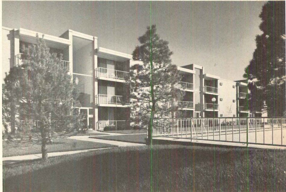
BUILDING ENTRANCES have three-story-high entry towers that bring daylight to all three landing levels. Community pool is in foreground at right.
