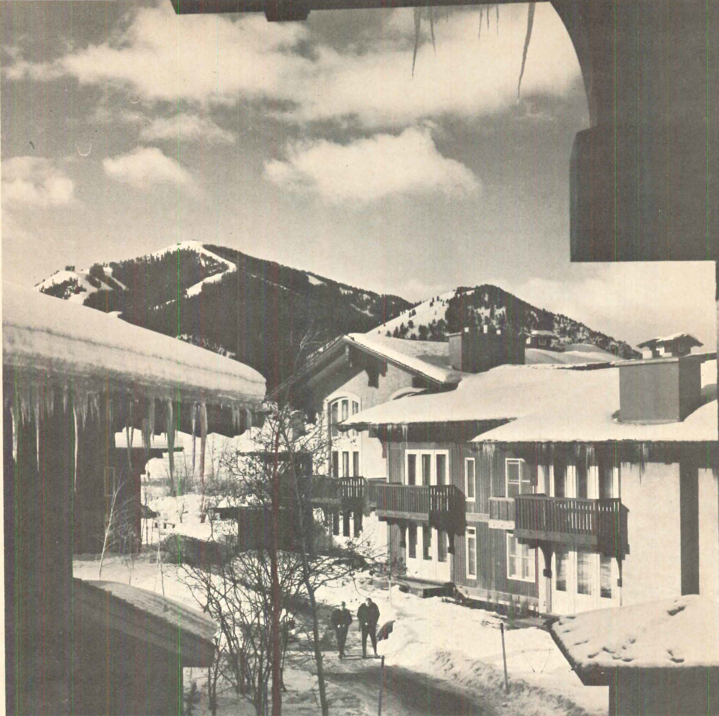
INFORMAL GROUPING of resort condominiums disguises fact that units are built to a strict module. Buildings are oriented to mountain view.
