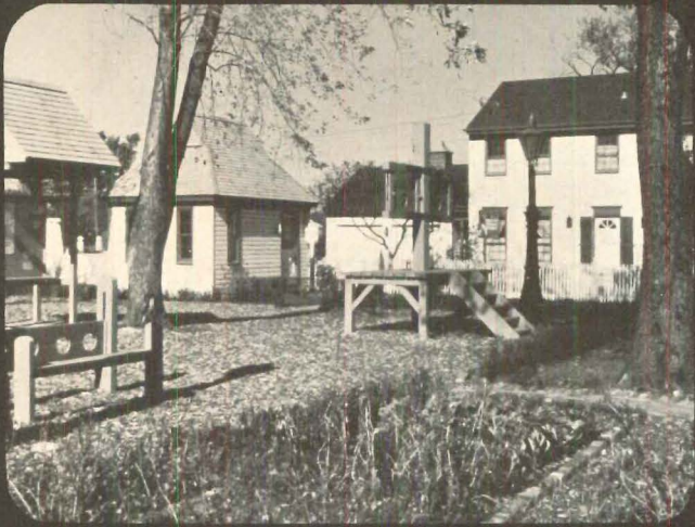
HISTORIC THEME IN A SALES AREA. John S. Clark, Northbrook, Ill., shows colonial models, like the one at right, around a replica of an old village common with public stocks and other historic touches. Small building is sales office.
