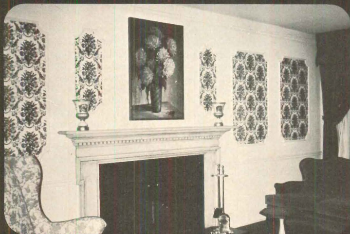
WALLPAPER PANELS. Colorful patterns are framed by stock molding applied over drywall. Other stock millwork forms the chair rail and the trim around the fireplace. Builder Alfred H. Mayer of St. Louis puts these decorative details in a house priced at $35,490.
