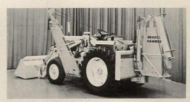
**Pipe-setter tractor** combines four tools to do the entire job: It breaks concrete (or other surface), digs a trench, lays pipe, backfills, and tamps. Hydraulic slide boom handles up to 4,500 lbs. International Harvester, Chicago. *Circle 267 on Reader Service card*
