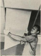
**Radiant heating panels** for use in suspended ceiling grids come in two models: 1) a 750watt unit with three to six heaters per control and a 2,560 Btuh rating; 2) a 500-watt model with four to eight heaters. Litecontrol, Watertown, Mass.
