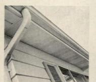
Aluminum soffit and fascia, coated with Tedlar, is guaranteed for the life of a house. Line includes two soffit styles—ventilated and solid—one fascia design, and a selection of runner channels and finish trim. Alsco, Akron, Ohio.
