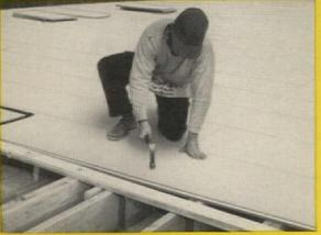
Structurally strong, weatherproof Homasote Floor Decking always gives you more value per dollar. In 4 ways: **sub-flooring, underlayment, sound control, and insulation!** Nailing the decking directly to floor joists and applying carpeting and pad complete the job. Insulation value is constant and sound-deadening characteristics can be measured by ISO R-140 and FHA 750 test results of INR +21 and STC 50. (Complete test data available on request.)
