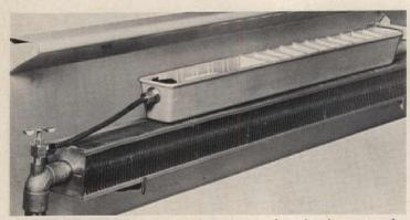
**Automatic humidifier** uses preheated water from heating system for faster evaporation. It is set on heating coil and connected to system at regular air vent. Two units will keep a 1,000-cu.-ft. room comfortable. Three S, Esterville, Iowa. *Circle 235 on Reader Service card*
