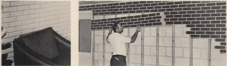
ALUMINUM PANELS interlock horizontally and vertically, are nailed to furring. Finished installation in white is shown above, at right.
