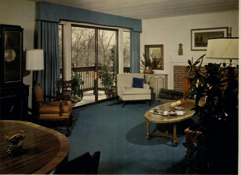
SLIDING GLASS DOORS open from living room to balcony of Ethan Allen model. Double-glazing and extra register in front of door minimize cold drafts.
