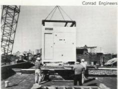
STACKING CORES inside pre-cut shaft in fivestory building is done through hole in roof.
