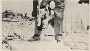
**Gasoline-driven rotating hammer** bores holes up to 2". An allattitude carburetor allows full-speed operation in any position, so it can work upside down for jobs on ceilings and horizontally for boring walls. Skil, Chicago. *Circle 261 on Reader Service card*
