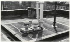
CAPPING core installation requires hooking up plumbing stack and heating vents atop shaft.
