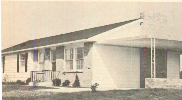
CUSTOM EXTERIOR shows three options—brick facade, fireplace, carport—a sectional builder can offer.
