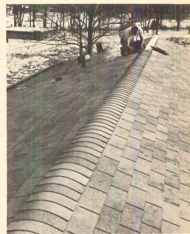
SHINGLES , plus felt and flashing, are added to cover up eave hinge and ridge. Capital also includes prefinished soffit system.
