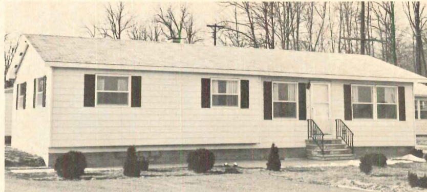
NEW MODEL —with higher roof pitch and conventional windows and siding—abandons all ties with mobile home, though Capital manufactures both on adjacent production lines.
