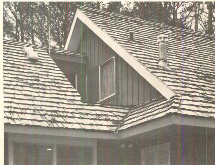
UPSTAIRS WINDOW for bedroom (5) was created by cutting out section of adjoining roof line. Cost was negligible.
