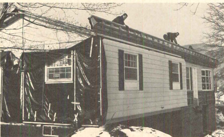
HINGED OVERHANG is lowered for exterior finishing after house sections have been drawn together at their perimeter beams (by hook and ratchet) and bolted.
