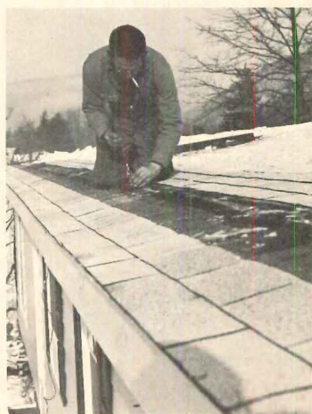
SHINGLES , plus felt and flashing, are added to cover up eave hinge and ridge. Capital also includes prefinished soffit system.
