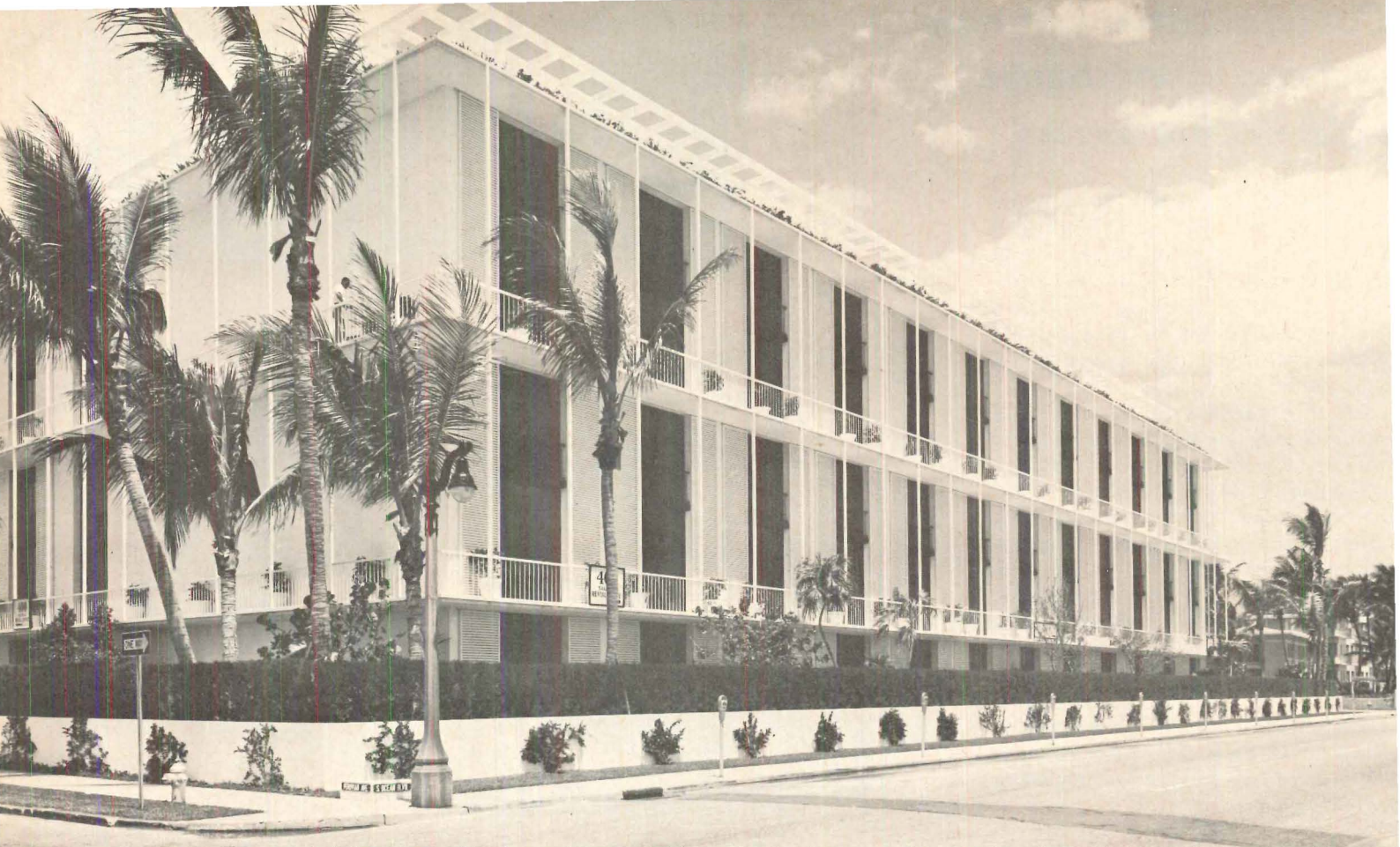
DISTINCTIVE DESIGN includes two-story-high louvered panels and long verandas that are reminiscent of southern colonial architecture.
