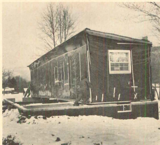
7. PUSHING a section is so easy that sometimes it takes only a stiff breeze and an anchor chain.
