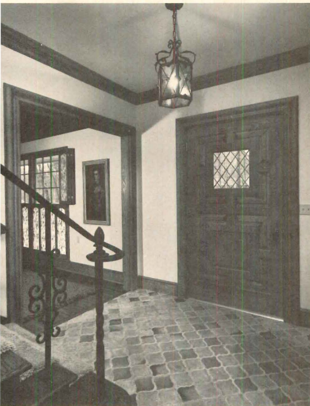
FRONT ENTRY (1 in plan, below) has oversized panel door that cost $70. Matching wooden trim (stock fireplace surround at 70¢ a foot) was used as crown and door molding. In all, $90 worth of extra trim was added throughout the house.
