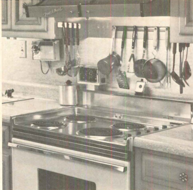
UTENSIL RACKS surround electric range. Plastic laminate covers walls as well as counter tops. Cost: $1 a sq. ft.
