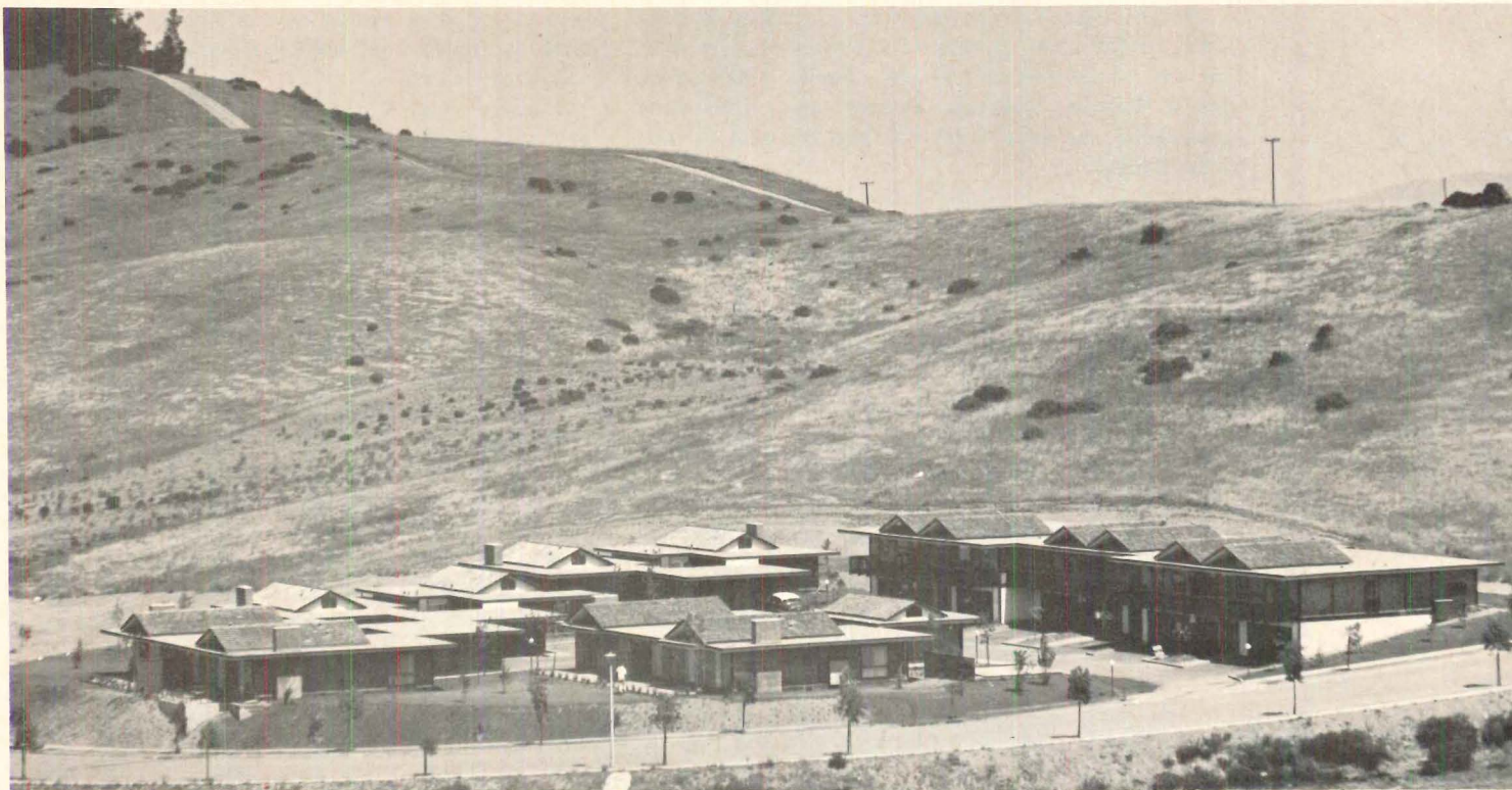
COMPACT PLAN places units along the perimeter of the pie-shaped, 1.3-acre site. All the private patios face outward; parking is in the center.
