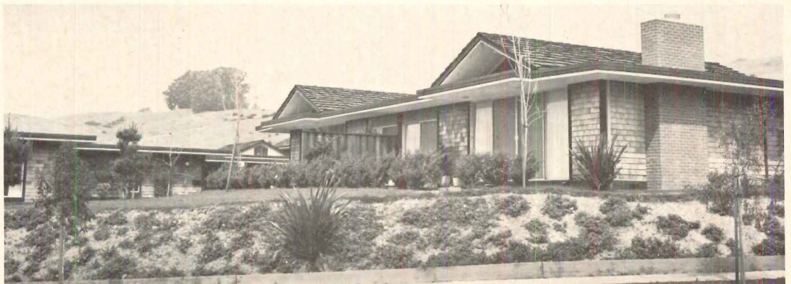
ON-GRADE UNITS have rear patios facing golf course, plus private courtyards behind garages.
