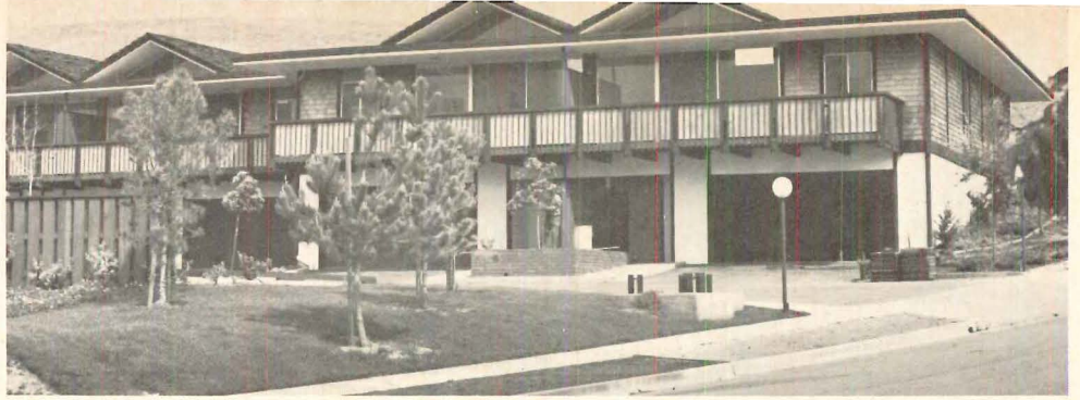
UPHILL UNITS have both balconies and on-grade patios. Living areas are above private garages.
