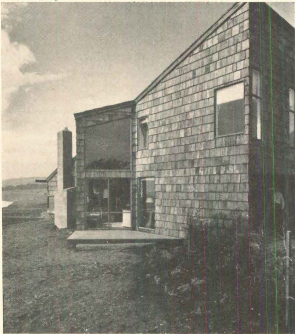
SHELTERED SIDE is high, opens to living-room deck, center, and dining terrace at far right.
