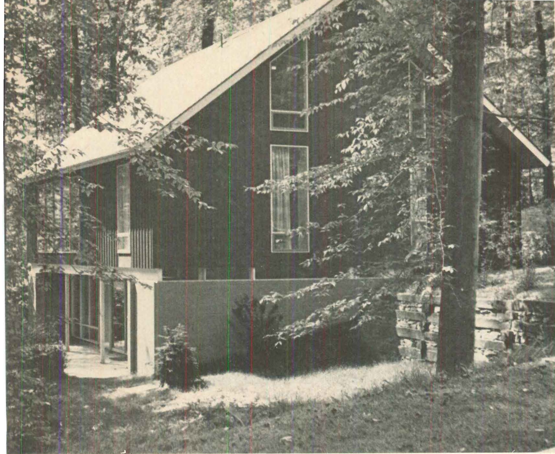
GABLE-END WALL has lower-level strip windows over which upper levels of house seem to float.
