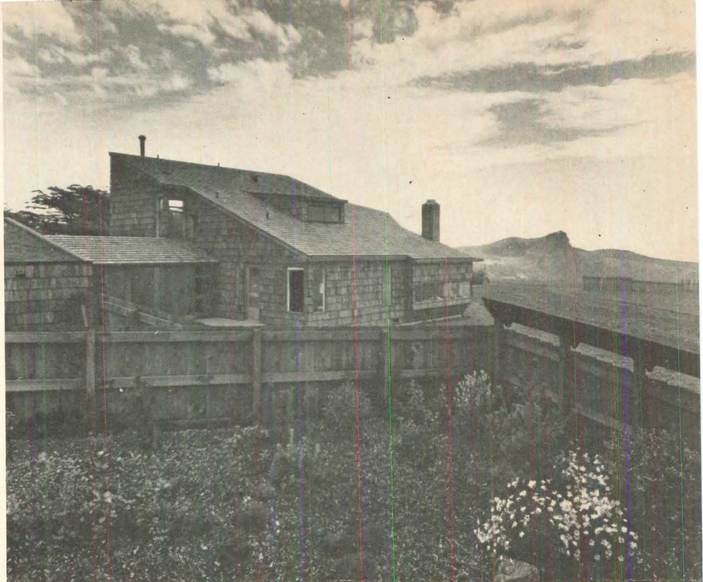
WINDWARD SIDE is low to reduce buffeting. Baffles on fence deflect wind from neighbor's yard.
