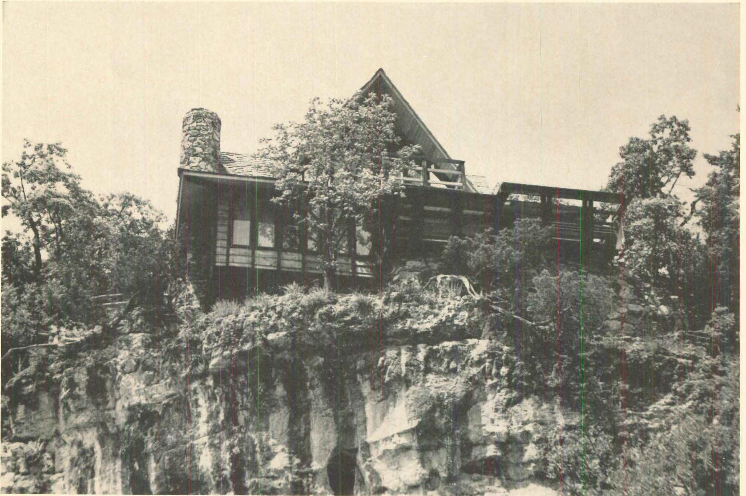
CLIFF-SITED HOUSE required hand-dug foundation to prevent damage to overhanging trees. Massive round chimney was built entirely of native stone.
