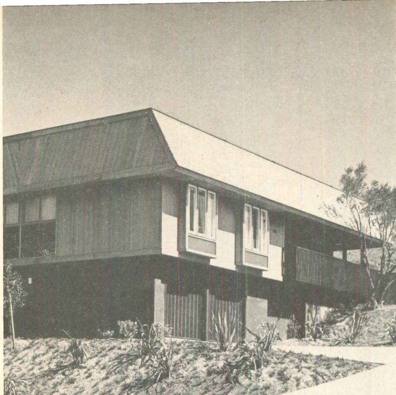
BROAD ENTRY DECK , right, is reached from uphill side of lot. Siding is stained redwood.
