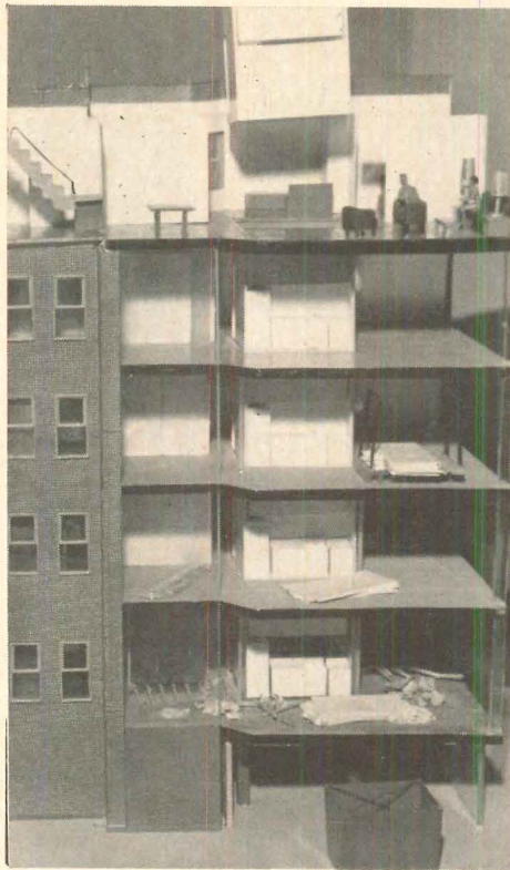
CAN-OPENER SYSTEM shown by model; drops materials through 8' x 8' hole in roof and floors, then closes shaft by stacking plumbing cores.
