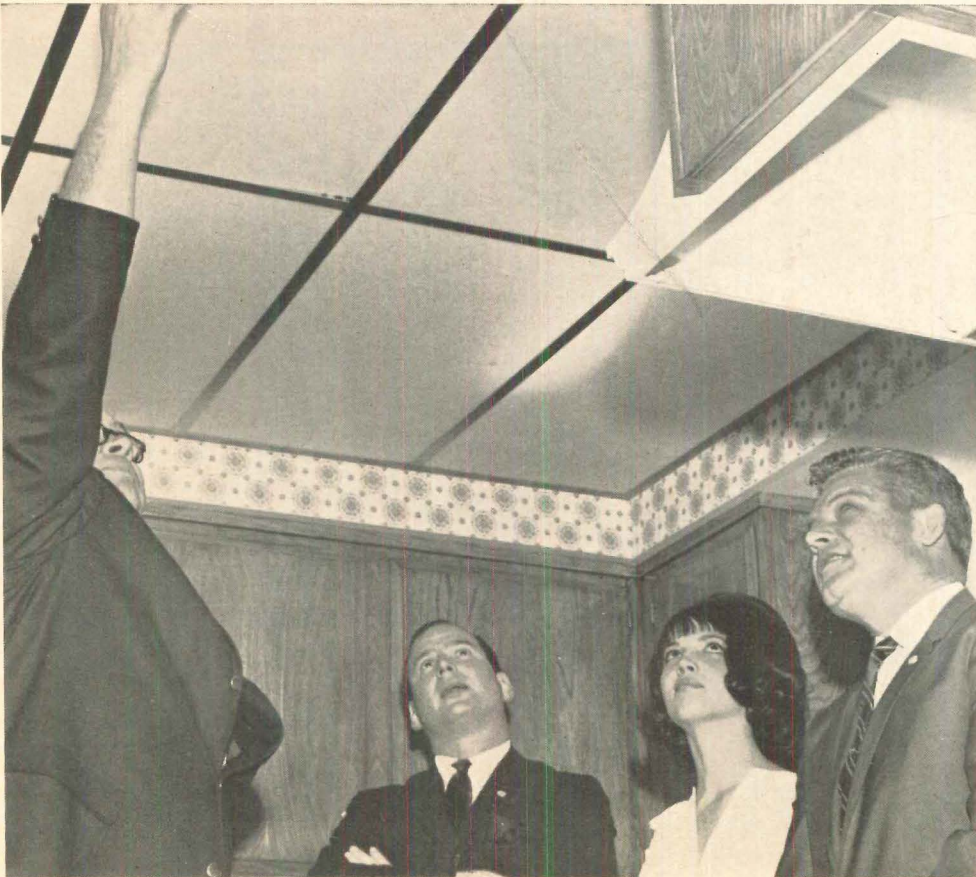
Still demonstrating in the kitchen, the salesman shows how the luminous-ceiling panels can be removed for easy cleaning and re-lamping. Other salesmen make notes on his performance.
