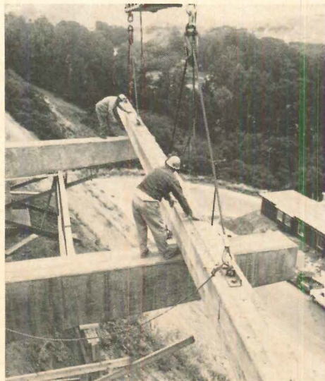
PRECAST BEAMS top off bents, providing support for deck. Wood beams can be substituted.
