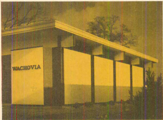
MDO plywood on a branch bank
