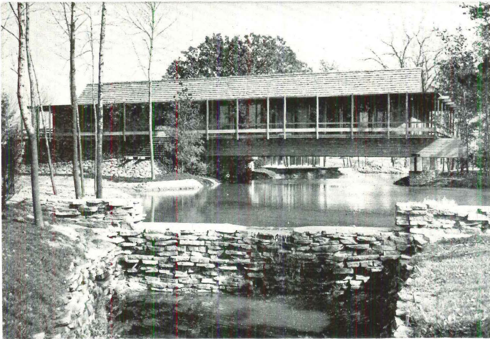
LONG SPAN over man-made pond is bridged by 1"x4" glue-lam beams on stone-faced concrete
