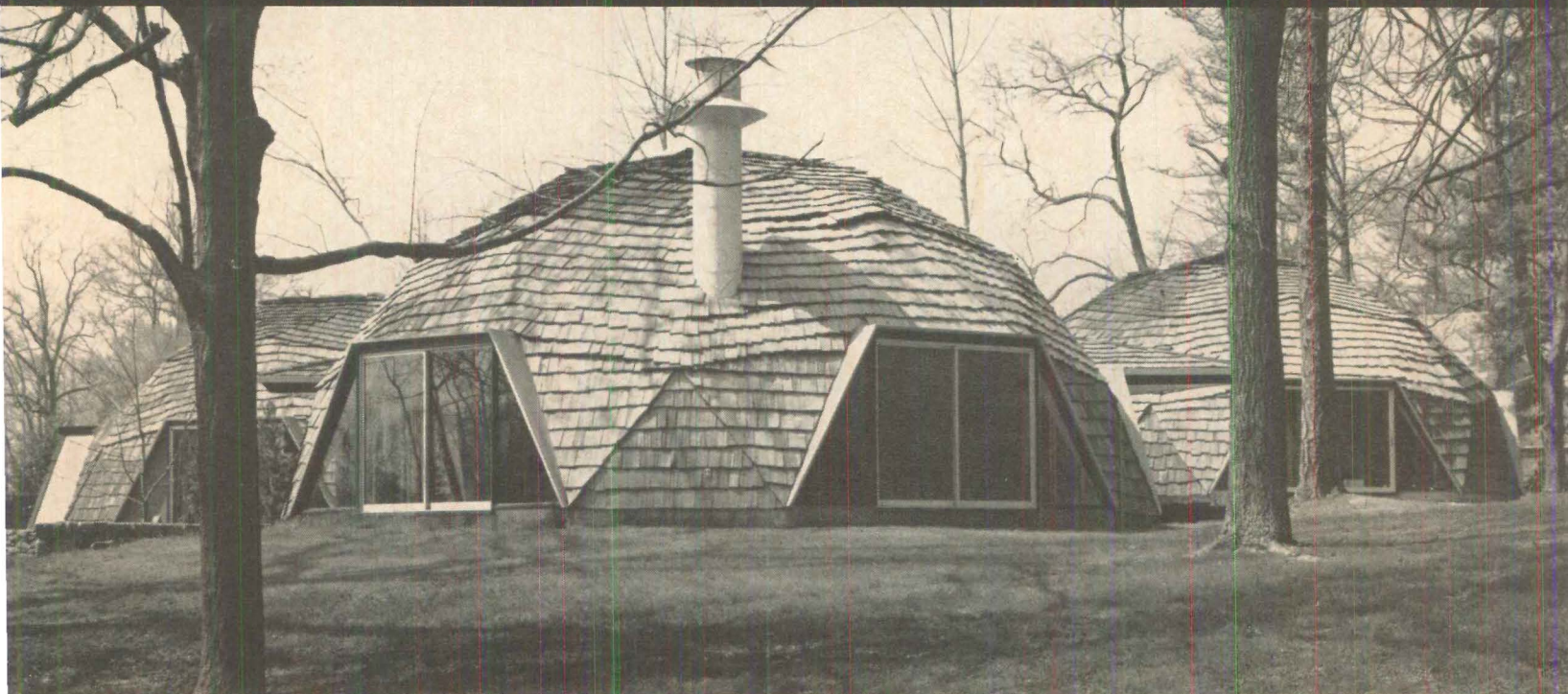
Residence, Narberth, Pennsylvania Architect: Stein and Rowland Associates Certi-Split Handsplit-Resawn Shakes, 24" x 1/2" to 3/4" with 8" to 10" to the weather.
