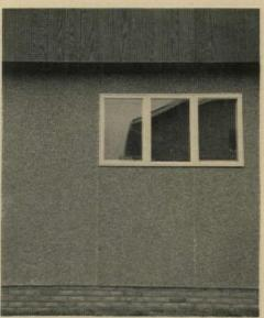
an exposed seam (above) between 4'-wide panels, but manufacturer supplies a touch-up kit of matching aggregate to avoid use of batten strips.
