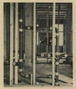
**PLASTIC-SEALED JOINT** in cast-iron pipe is enclosed by metal sleeve. System eliminates cumbersome hub joint, makes pipe more flexible.
