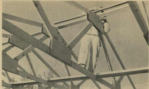
**ROOF SYSTEM** is framed by 2x4 trusses on 4' centers. Bottom chord of each truss spans 28', is spliced at the center by a factory-made finger
