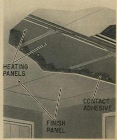
LAMINATED CEILING on second floor incorporates electrodes for electric resistance heating. Heat for first floor is by heat pump and ducts.
