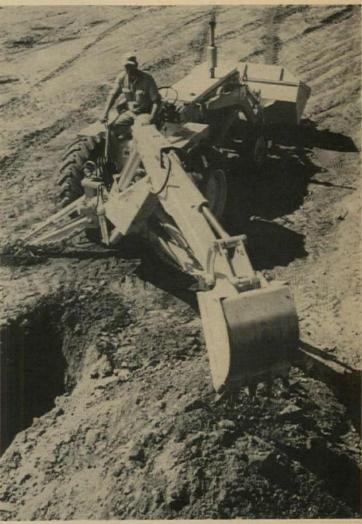
Hydraulic-cushioned backhoe digs to 121/2', operating at 2,100 psi. It has full feathering control and simultaneous crowd, lift and curl action. Two other models dig to 14' and 15'. Bucket widths: 12" to 36". Int'l Harvester, Chicago. (Circle 218 on Reader Service card)
