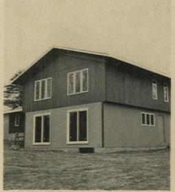
PLASTIC-CLAD WALLS and windows practically eliminate outside maintenance. Factory-applied aggregate-on-epoxy finish on lower walls leaves
