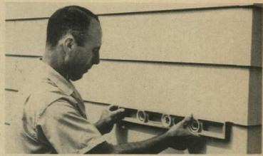
**Aluminum siding** has a weave pattern surface. The siding is finished with a nonchalking acrylic enamel paint available in six colors. Panels have a self-aligning snap lock to reduce installation time. U.S. Aluminum, Franklin Park, Ill. (Circle 236 on Reader Service card)
