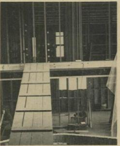
WALL SYSTEM differs at each level. First-floor studs are 4' apart, but second-floor studs are on conventional 16" centers because 4' stud spacing
