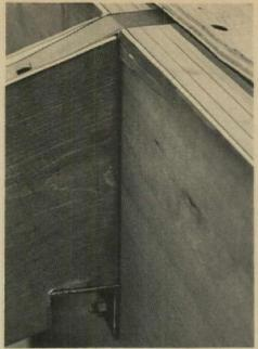
**LAMINATED BEAM** over carport is three 34"-thick boards and two thin veneers bonded together. Detail shows rafter strapped to ridge beam,
