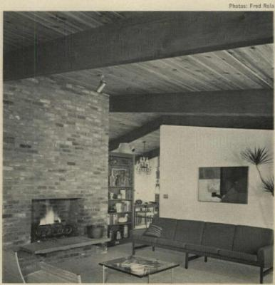
PLANK-AND-BEAM CEILING, shown here in the living room, is uncluttered because wiring for overhead fixtures runs through chases routed in the roof.
