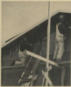
**BUILT-IN VENTS** open up roof continuously on all four sides. Sheathing-siding is cut short to leave a 6" gap under eaves. Gap is covered with
