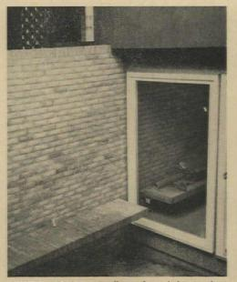
BUILT-IN LEDGES cantilever from below-grade brick cavity wall. Horizontal rods are tied to vertical reinforcing rods in wall, and brick ledge
