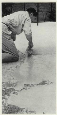
THIN COAT of silicone topping—usually 1/8" thick—is troweled on for \$1.00-\$1.75 per sq. ft.
