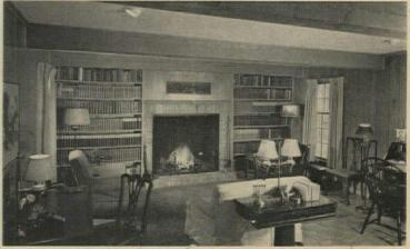
FAMILY ROOM has rough-sawn 8 x 10 ceiling beams which are structural as well as decorative, permit use of light 2 x 8s as second-floor joists.
