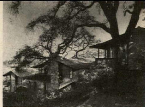
LOW SILHOUETTE gives stepped-down buildings the look of three separate hillside houses.
