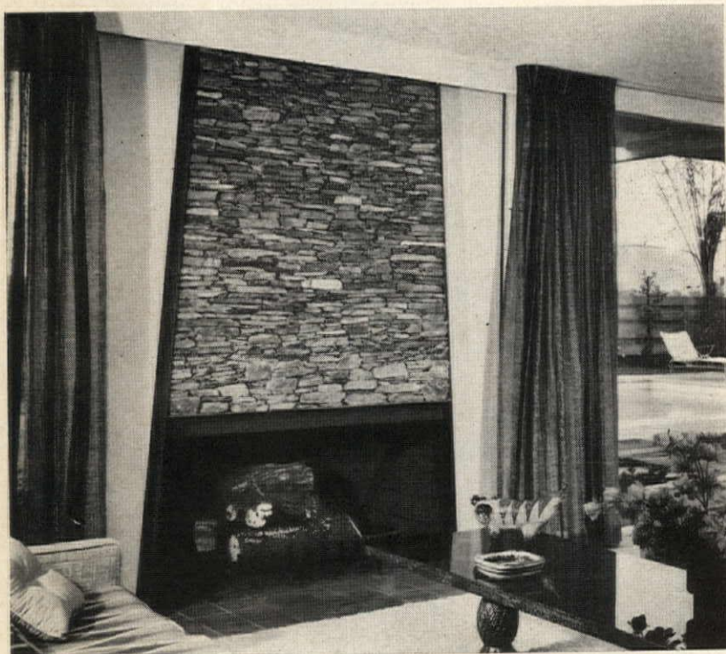
CHINK-LAID STONE FRAMED IN STEEL
