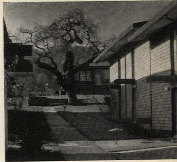
EXTERIOR MATERIALS include cedar shingles and redwood trim. Low fixtures illuminate walks.
