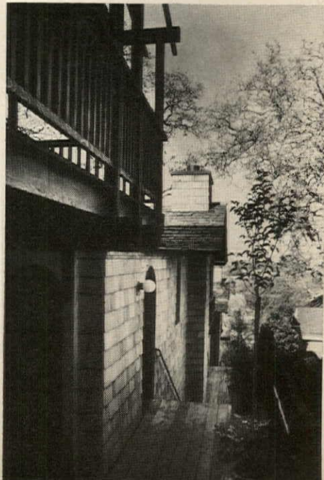
WOODEN WALKWAYS go down both sides of buildings. Arched door, left, leads to entry court.
