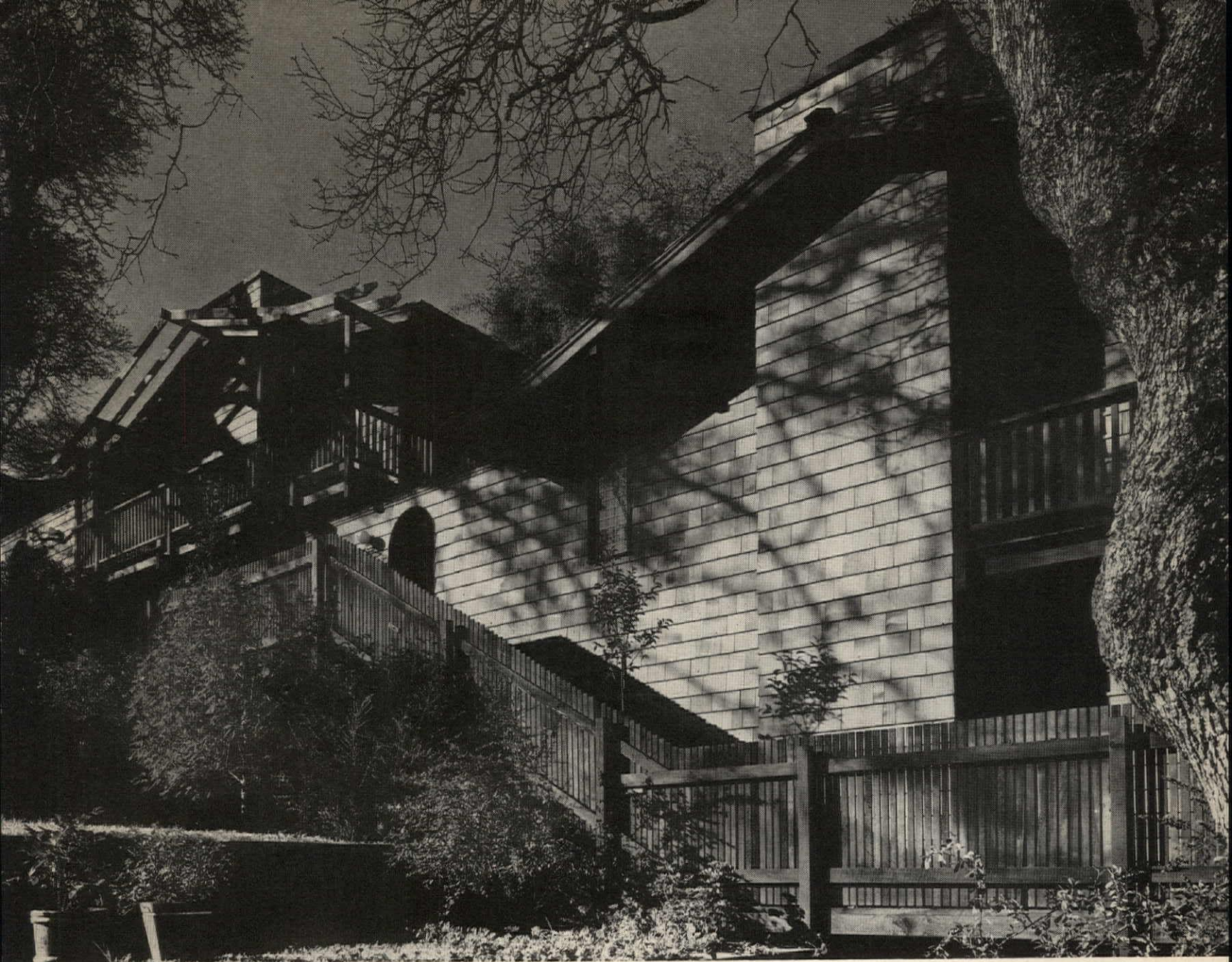
WOOD-SHINGLE SIDING and wood-slat fencing harmonize with the site's big trees and planting. Note terraced lawns.
