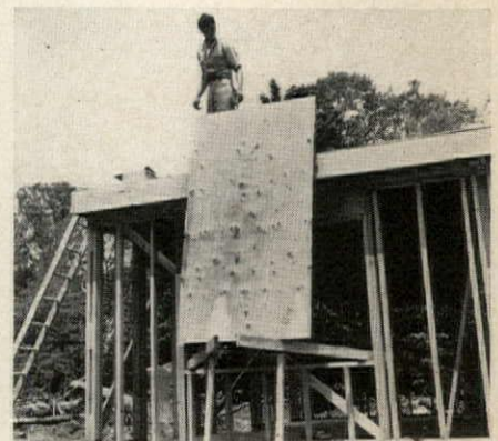
LOW-COST AIDS like this scrap-lumber sheathing holder help keep down overhead.
