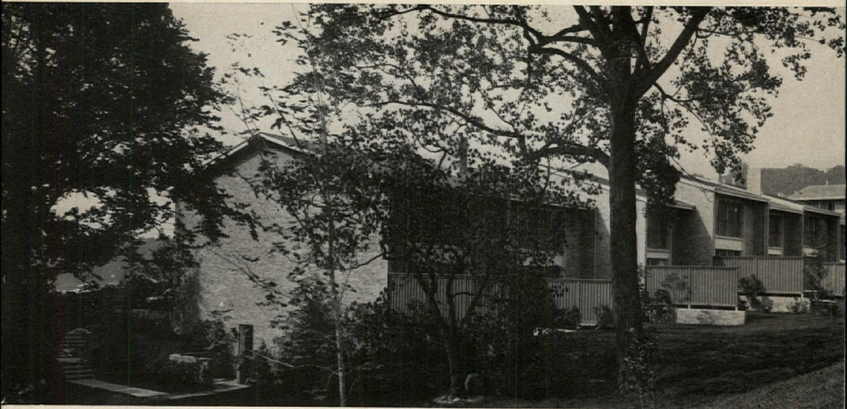
STAGGERED SETBACKS AND ELEVATIONS let rows of townhouses follow the natural topography of the rolling 68-acre site.
