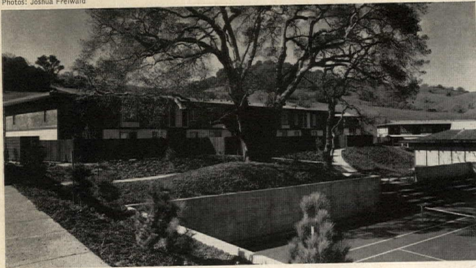
TENNIS COURTS are part of recreation center. Slatted fences shelter patios of nearby apartments.
