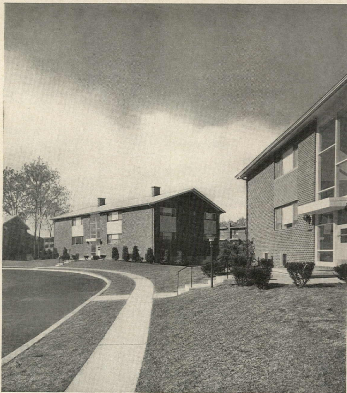
HILLTOP APARTMENTS , Baltimore, Maryland, use York air conditioning systems, including Borg-Warner furnaces, to assure year-round comfort. Builders, Gorn Brothers.
