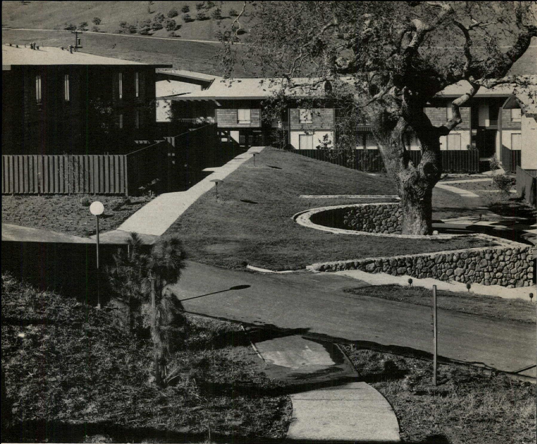
LAVISH LANDSCAPING includes stone retaining walls to preserve large existing trees. Land contours were left undisturbed, and all utilities are underground.
