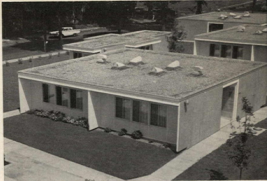
FOUR-UNIT BUILDING has reinforced concrete walls. Two units open off entry door at right.
