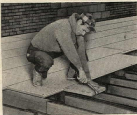
Weatherproof, all wood-fibre Homasote Floor Decking eliminates separate cutting, fitting and nailing. Carpet and pad can be installed right over "4-Way"—resilient floor covers need only an additional layer of hardboard or plywood. Write for Bulletin 4-212.
