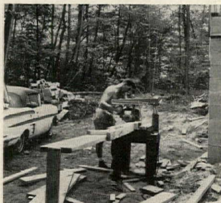
PRECISE CUTS —for tight fits and true alignment—are made by radial-arm saw.
