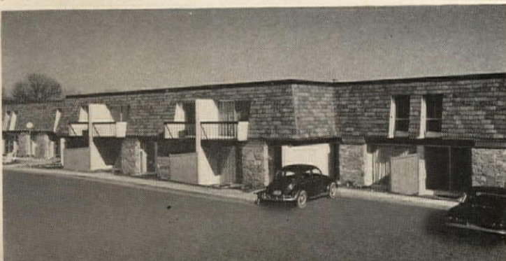
FRONT ELEVATIONS are broken up by setbacks, party walls and deep second-floor windows.
