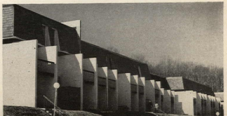
REAR ELEVATIONS of downhill models have extended masonry walls that create private patios.
