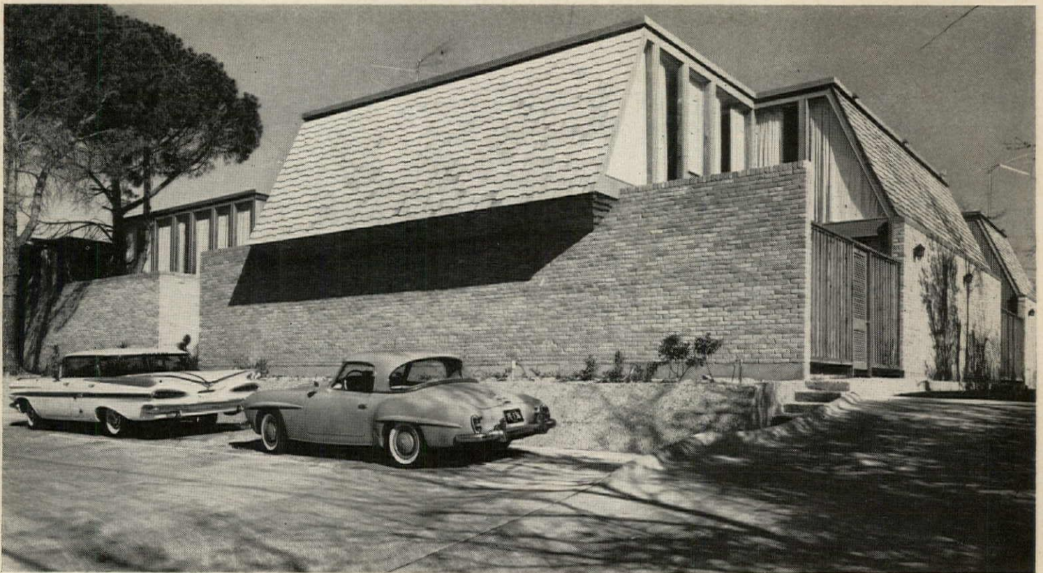
MANSARD ROOF , broken by glass gable ends, helps reduce scale of six-unit building. Mexican adobe brick was used for walls, cedar shakes for roof.
