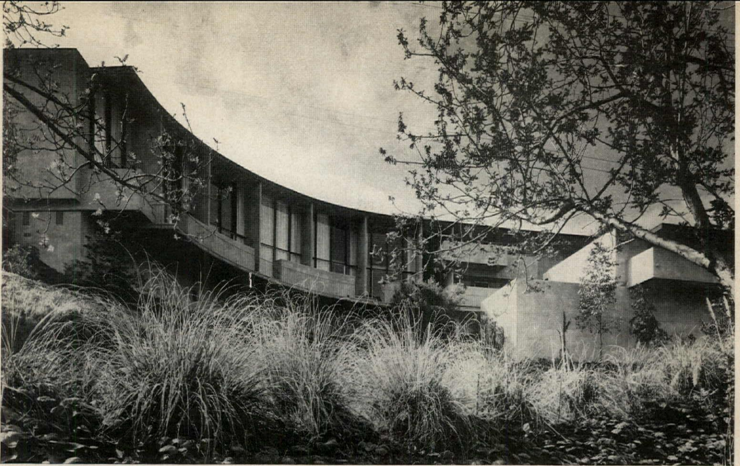
CURVED FACADE has cantilevered balconies, overhanging roof and fin walls for privacy between units. Building at right has indoor parking on lower level.
