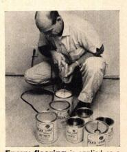
Epoxy flooring is applied as a liquid over almost any surface. Flooring is tack-free in several hours and can withstand traffic in a day. A textured effect with plastic confetti (right) is one special effect possible. Flex-Coat, Paramount, Calif.
