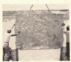
**SLAB** is slipped between piles until notches in bottom corners lock into matching notches in piles.
