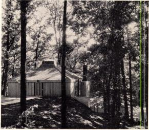
**SIMPLE FACADE**, with windowless walls of 1x3 t&g cypress, gives no hint of glass walls facing views at side and rear.
