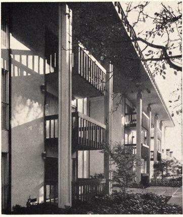
**REGULAR SPACING** of decorative roof columns, plus vertical detailing on balcony railings and fascia, increases facade's apparent height.
