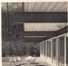
**STEEL ROOF** is carried out in an 8' overhang. Sliding doors and windows are steel framed.
