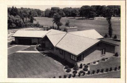
You be the judge. First off, note that Fire-Chex Shingles contain more asbestos than any shingle of equivalent weight. Probably why Fire-Chex was first to earn the U/L Class "A" Fire-Safety Rating. And to protect against high winds, Fire-Chex gives you exclusive Sta-Seal® Tabs that bond one shingle course to the next on light pressure contact. Also, Fire-Chex has been proved in 15 years of field use with millions of
