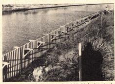
**BRACES** are bolted to the ½"-thick interlocking asbestos sheets to carry concrete cap form.
