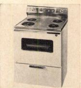
Electric range in white or shaded copper has a brushed chrome tilt top and backsplash. Infinite heat controls, an automatic timer and an appliance outlet are included in the 30" unit. Suggested retail price: \$179.95. Philco, Philadelphia.
