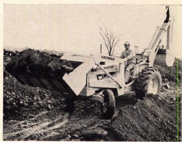
**Industrial wheel tractor** is equipped with loader and backhoe. The backhoe has a 30"-wide bucket with a 9.9-cu.-ft. capacity and can dig 15' deep. The loader has a 3,200-lb. capacity. Allis-Chalmers, Milwaukee. (Circle 230 on Reader Service card)
