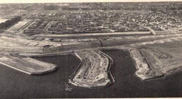
OCTOBER: DREDGING ENDS and bulkheading is nearly done, followed closely by backfilling.
