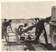
**PRECASTING** of 6'x8' seawall slabs is done at site. Forms are steel angles on level ground.
