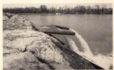
RUNOFF WATER flows over dike from filled section, left, into excavated lake, right.
