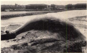
WATER BOUND FILL is self-compacting and leveling. Dike, left, is at final fill height.
