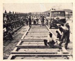
PARTITION FORMS of glass fiber are wired before pour. Panels cure on wood racks at left.
