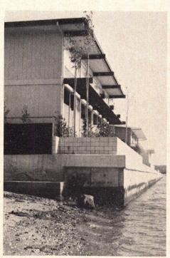
**CONCRETE BULKHEAD** capped by reinforced bond beam permits homebuilding at water's edge.
