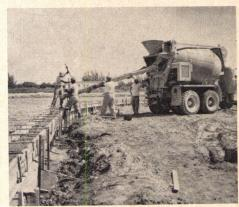
CAP of reinforced 3,000-lb. concrete, 18" wide and 6" deep, finishes and ties seawall.
