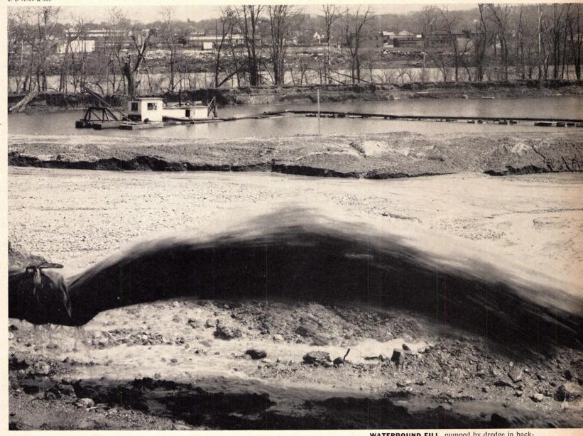
**WATERBOUND FILL**, pumped by dredge in background, gushes into settling basin (see p. 94).
