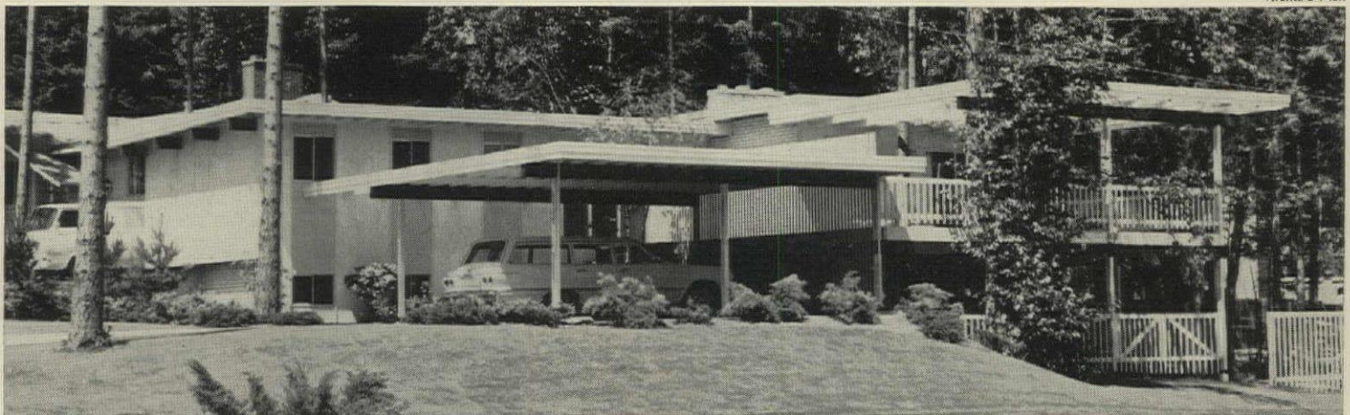
CARPORT GRADE can be adjusted to site variations in this $24,000 (plus lot) Seattle house.
