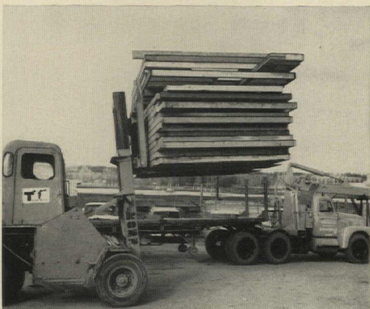
FORKLIFT loads panels on boom truck which delivers two houseloads on each trip. All houses, including odd-lot units, are supplied this way.
