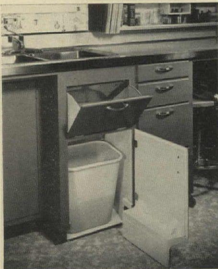
Garbage unit has top hopper that feeds can.
