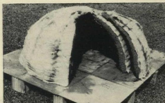
INSTANT IGLOO is a plastic sheet ignited to form a foam shell.
