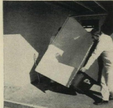
BATHTUB of glass-fiber-reinforced plastic has integrally molded walls.
