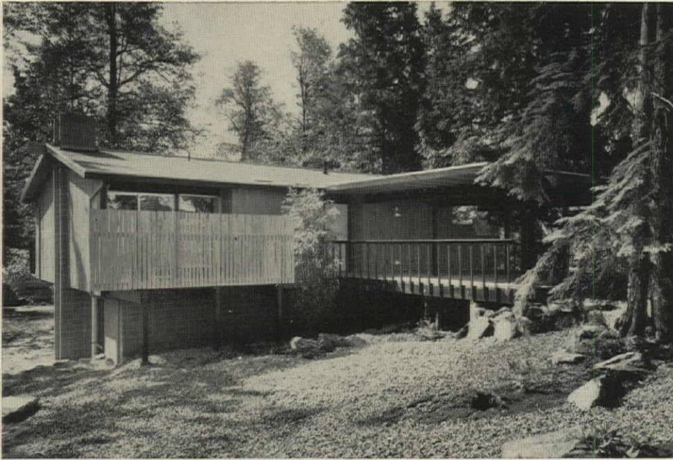
CARPORT-BRIDGE leads from street to upper level of $24,500, two-story hillside house.
