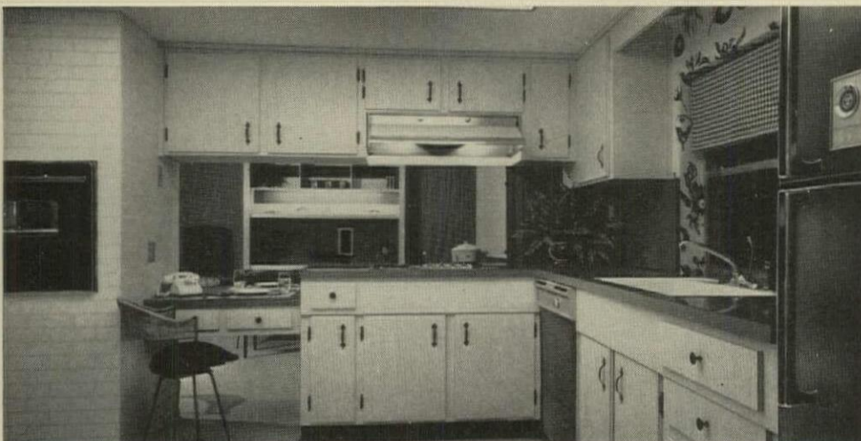
Bridge desk , left in photo, is simply a short counter section, with drawers underneath, hung between the base cabinets and the oven wall. The low counter continues
