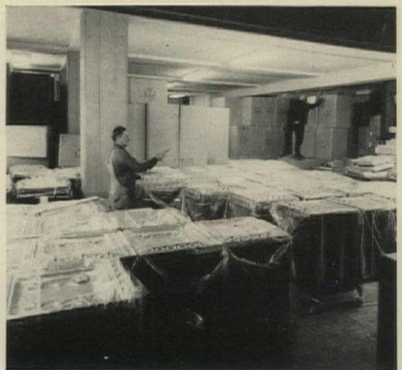
2. ON-SITE WAREHOUSE insures continuity of supply and no job delays. Located in Hillside Apartments' auditorium, it lets Olshin keep at least 50 complete kitchens on hand.
