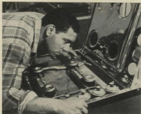
3. APPLIANCE SHOP is set up in the auditorium to test new equipment prior to installation and make minor adjustments and repairs. Workman above checks gas flow on range.
