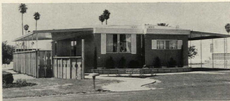
$8,000 MODEL , combining two 10'x55' sections, is extended at sides by patio and carport roofs.
