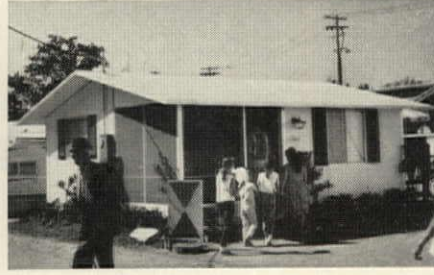
ROOF PANELS bear on, and are riveted to horizontal wall angles. Fascia is riveted on.
