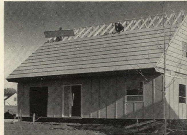
High-speed roof system uses 2 x 10-ft. Bermuda shingles made of Hypalon-surfaced plywood. It took four men six hours to install, starting at eaves with concealed nailing and folding up successive courses of the shingles. Hypalon film acts as a continuous hinge at interlocking horizontal joints.
