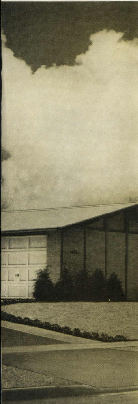
To make the 28-ft. tilt-up wall sections, 1/2" Exterior plywood, presurfaced with Tedlar, was fastened to studs on 24" centers, then battens were blind-nailed to cover stud nails. Battens, window casings, trim and plywood soffits are also Tedlar-surfaced.
