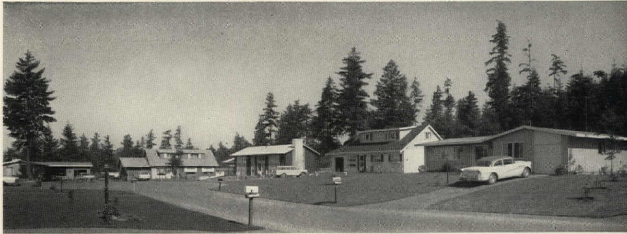
Most Mayer/Peterson houses are between $10,000 and $17,000 and are in medium-sized developments like this, a group of 17 near Lakewood, Washington. Most of these were sold before completion. All houses use plywood component systems, but vary widely in siding and architectural styles ranging from ranch to colonial (below).
