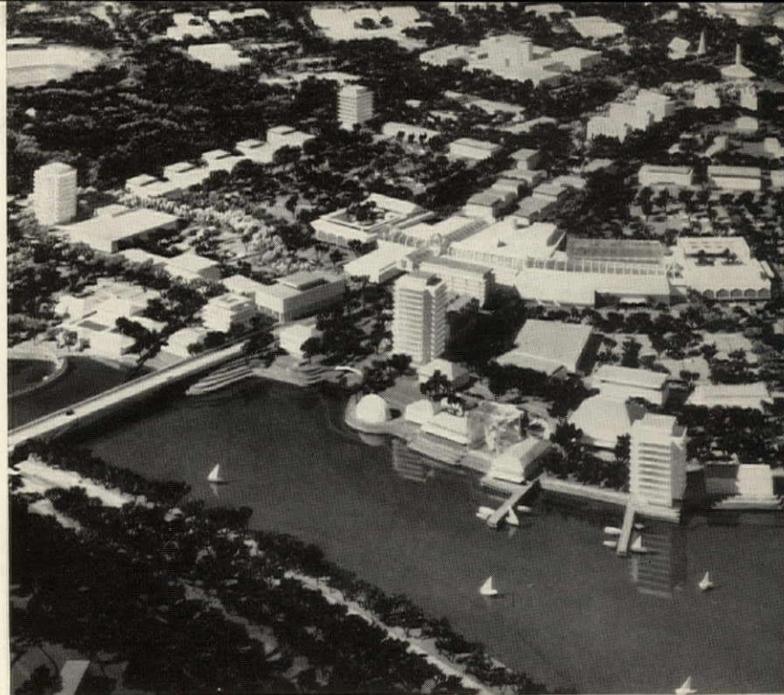
TOWN CENTER , as shown in model, will hug lake formed by damming of Little Patuxent River. Route 29, at left, is crossed by bus-route bridge.
