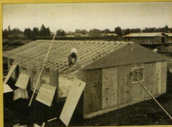
5. PlyScord roof sheathing is stacked alongside the house so the crew can reach it easily. Mayer/Peterson have never used anything but plywood for roof decking on their houses.
