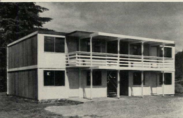
FINISHED FOURPLEX built of sections shown above required less than a week of site work.
