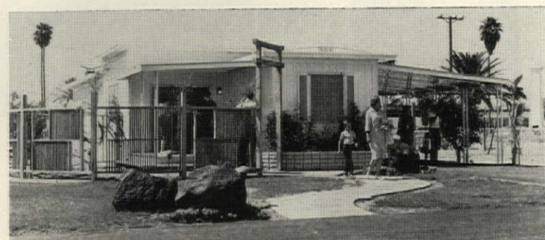
$10,000 MODEL combines 10'-wide sections of different lengths to create setback for entry.
