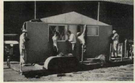
WALLS AND GABLE ENDS , finished on both sides and wired, are shipped partly assembled.
