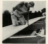
**Roof framing system** includes laminated beams and laminated roof decking. Beams are 4' x 10', 6' x 10' or 6' x 12' and from 12' to 60' long. Deck planks are 6" wide and 3",  $3\frac{1}{2}$ " or 4" thick. Edges are beveled. Weyerhaeuser, Tacoma, Wash.
