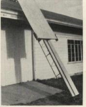
**Electric conveyor** can deliver six pieces of sheathing per minute to upper levels of a building. Lightweight unit has <sup>1</sup>/<sub>4</sub> hp electric motor that operates on regular 115-volt current. Can also lift roofing or nails. Easy-Way Prods., Ponca City, Okla. *Circle 92 on Reader Service card*
