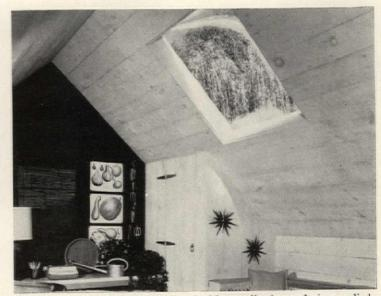
**Plastic skylight** has insulating double acrylic dome. It is supplied with framing and flashing pre-installed, can be set in place simply by nailing through a 3" aluminum perimeter flange. American Cyanamid, Cambridge, Mass. (*Circle 50 on Reader Service card*)
