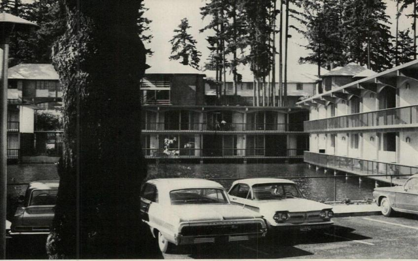
**TWO-STORY BUILDINGS** (seen from 2 in site plan) project over water on reinforced slabs.
