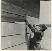
**Mineral-fiber siding** looks like wood, resists fire, warping, blistering, peeling and termites. Dura-shakes have a plastic finish that comes in five colors. They can be applied over existing siding as well as on new construction. Ruberoid, New York City. *Circle 46 on Reader Service card*
