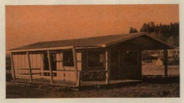
Osborne says only plywood will stand this rugged treatment without racking. His floors are  $\frac{5}{8}$ " plywood, glue-nailed to 2 x 4's. Walls are one layer of rough-sawn plywood with battens. Roofs are stressed skin panels. By using plywood to keep costs down, Osborne can give second-home buyers more house for the money.
