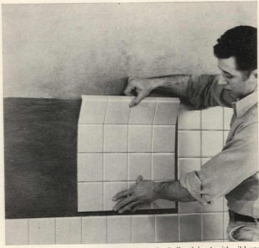
Large tile sheets are made of 16 standard tiles joined with ribbons for fast installation. Master-Set sheets also include cove or cap trim, can be set with conventional mortar, thin-set mortar or adhesive. American Olean, Lansdale, Pa. (*Circle 8 on Reader Service card*)
