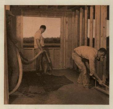
H. A. Briggs Company used a plywood and concrete system for soundproof floors in their Four Fountains apartments, Tacoma, Wash. (above and left).
