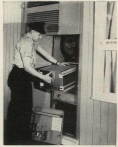
SLIDING RACKS make components easy to maintain or replace. Here air filter is removed.
