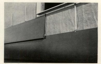
**Clear redwood siding** is treated with a transparent finish that is guaranteed against blistering, peeling, cracking or flaking for five years. Metal fastening system requires no nailing. Union Lumber, San Francisco, Calif. (*Circle 47 on Reader Service card*)
