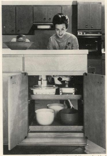
**Two-way access cabinets** can be used as dividers or for island or peninsula installations. Both base and wall cabinets are made with doors on front and back. Available in contemporary and provincial styles. Long-Bell, Longview, Wash. (*Circle 66 on Reader Service card*)
