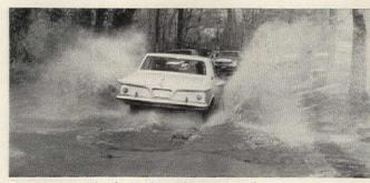
**FLOODING** results from clay soil, poor grading and paucity of storm sewers.
