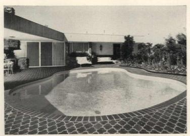
**Quarry tile** comes in a variety of shapes. Made of hard-burned shale, it is nonfading, stain resistant and can be installed indoors or out. Available with brushed or smooth surfaces. Ludowici-Celadon, Chicago. (Circle 32 on Reader Service card)
