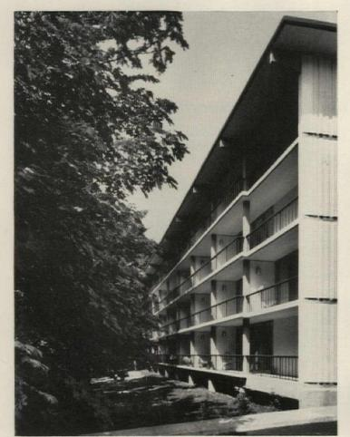
FOUR-STORY BUILDING (seen from 3 in site plan) has deep balconies with stub-wall dividers.
