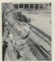
Adjustable wall ties permit mason contractors to erect cavity walls in two steps: 1) female ties are installed in interior wythe with eyelets protruding 2"; 2) exterior wythe is tied in with male ties. Dur-O-WaL, Cedar Rapids, Iowa.
