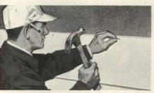
NAIL ALONG TOP EDGE. Siding won't split; vinyl color-coat won't chip. Nails easily, firmly. When complete siding job is done, nails won't show.
