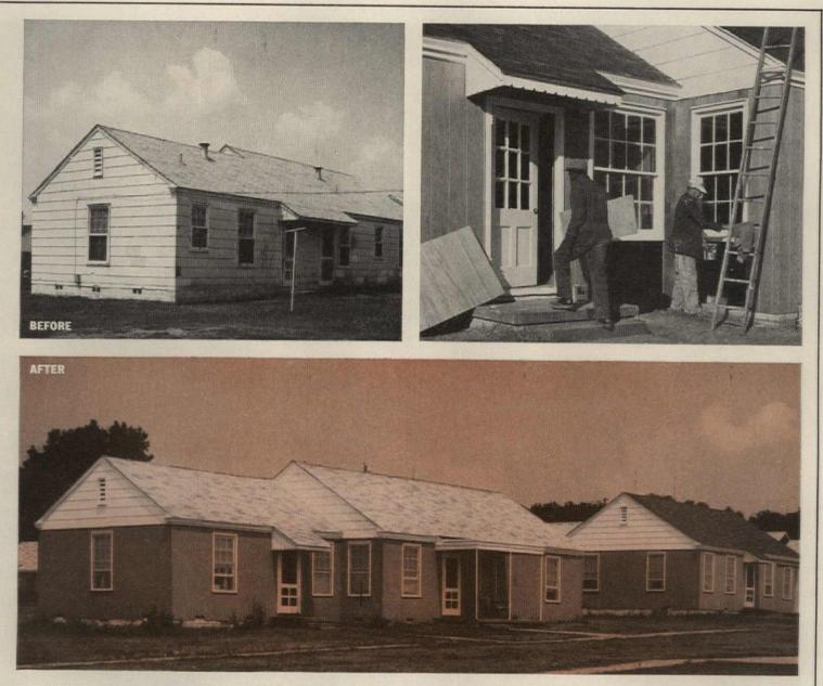
In Little Rock, Ark., this 56-unit housing project needed a face-lifting. Plywood did the job fastest, at lowest cost. Housing Administrator Robert Coxon specified grooved plywood siding to replace stained, broken asbestos shingles.
