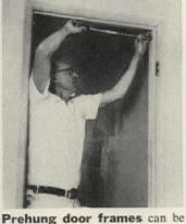
installed by one man in ten minutes. Presto frames have onepiece T&G construction with interlocking mitered joints. Casings, stop and hinges are factoryinstalled. Dexter Inds., Grand Rapids, Mich. Circle 135 on Reader Service card
