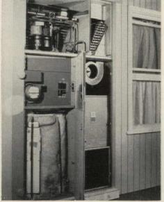
**COMPARTMENTED CABINET** houses heat pump and coils, circuit box, water heater, fan, filter.
