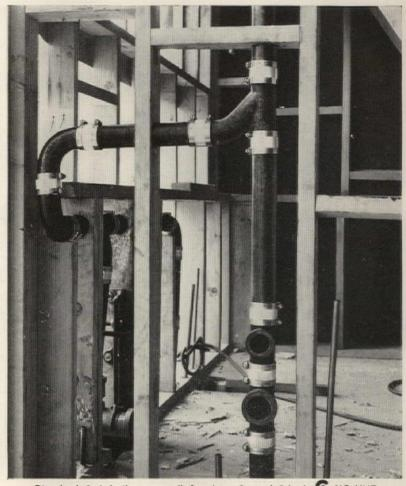
Standard 2x4 bathroom wall framing. 2- and 3-inch **G** NO-HUB pipe and pipe joints fit easily inside of partition and through drilled plates. Ideal for compact installations. Economical, too—all short pipe lengths are usable.
