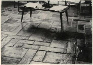
**Cast-stone flooring** has texture of natural stone, comes in lightweight, modular units ranging in size up to  $12" \times 18" \times 5\%"$  thick. Travertine marble and Spanish tile patterns are also available. Emco Mfg., Lorane (Reading), Pa. (*Circle 31 on Reader Service card*)
