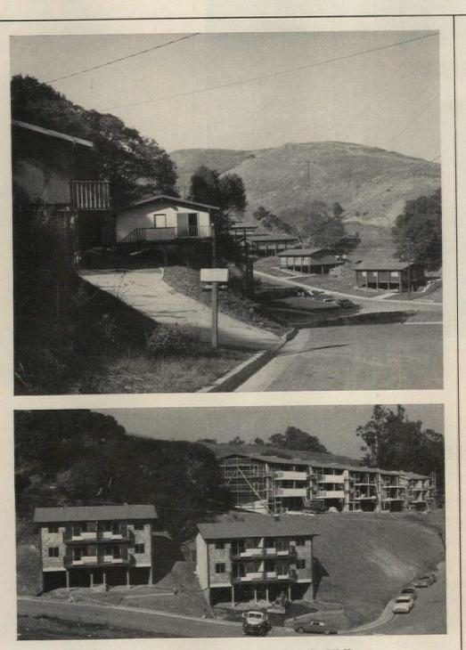
serves as both subfloor and underlayment for tile. Walls are plywood sheathing under stucco or shakes. Roof sheathing is plywood. Foreman Irwin Smith sums it up: "Plywood gives stronger structures with less waste and hardly any lost motions. It's easy to handle and makes neater jobs. I'm in favor of using plywood on all frame construction projects."
