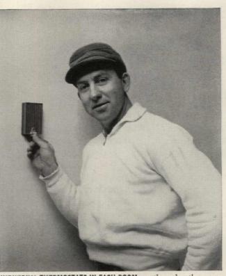
**INDIVIDUAL THERMOSTATS IN EACH ROOM** are the only other components needed to complete an electric ceiling cable system. A strong selling point with prospects, they allow homeowners to adjust the temperature in any part of the house separately.
