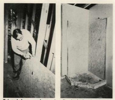
**Tub and shower enclosures** have Formica laminated to a styrenefoam inner core. Aqua-Wall is installed in precision channels, which are first attached to new or old walls. No adhesive is needed. Glass Shower Door Co., Chicago. (*Circle 57 on Reader Service card*)
