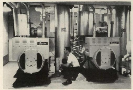
POWER PACKAGE uses generators run by natural gas engines, which in turn are connected to
