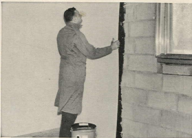
Bonding polystyrene foams—does not collapse foam.
