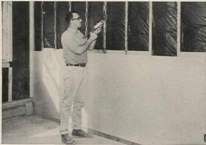
Stud adhesive—bonds to wood and metal.
