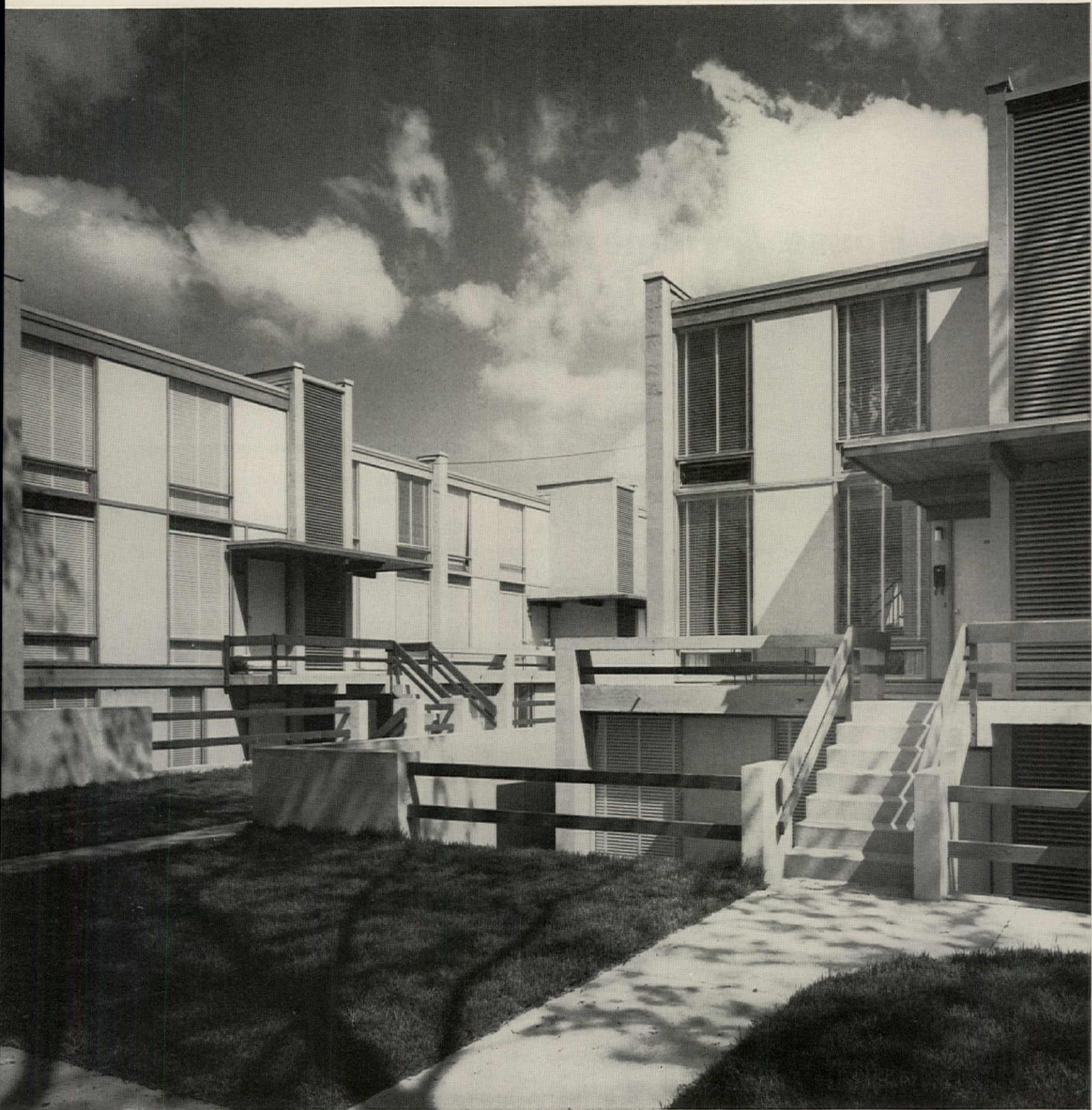
Vest-pocket project in New Haven, Conn., renewal area is an Honor winner (p. 52). Its ground floor is a half-story below grade, so no apartment is more than seven steps up or down.
