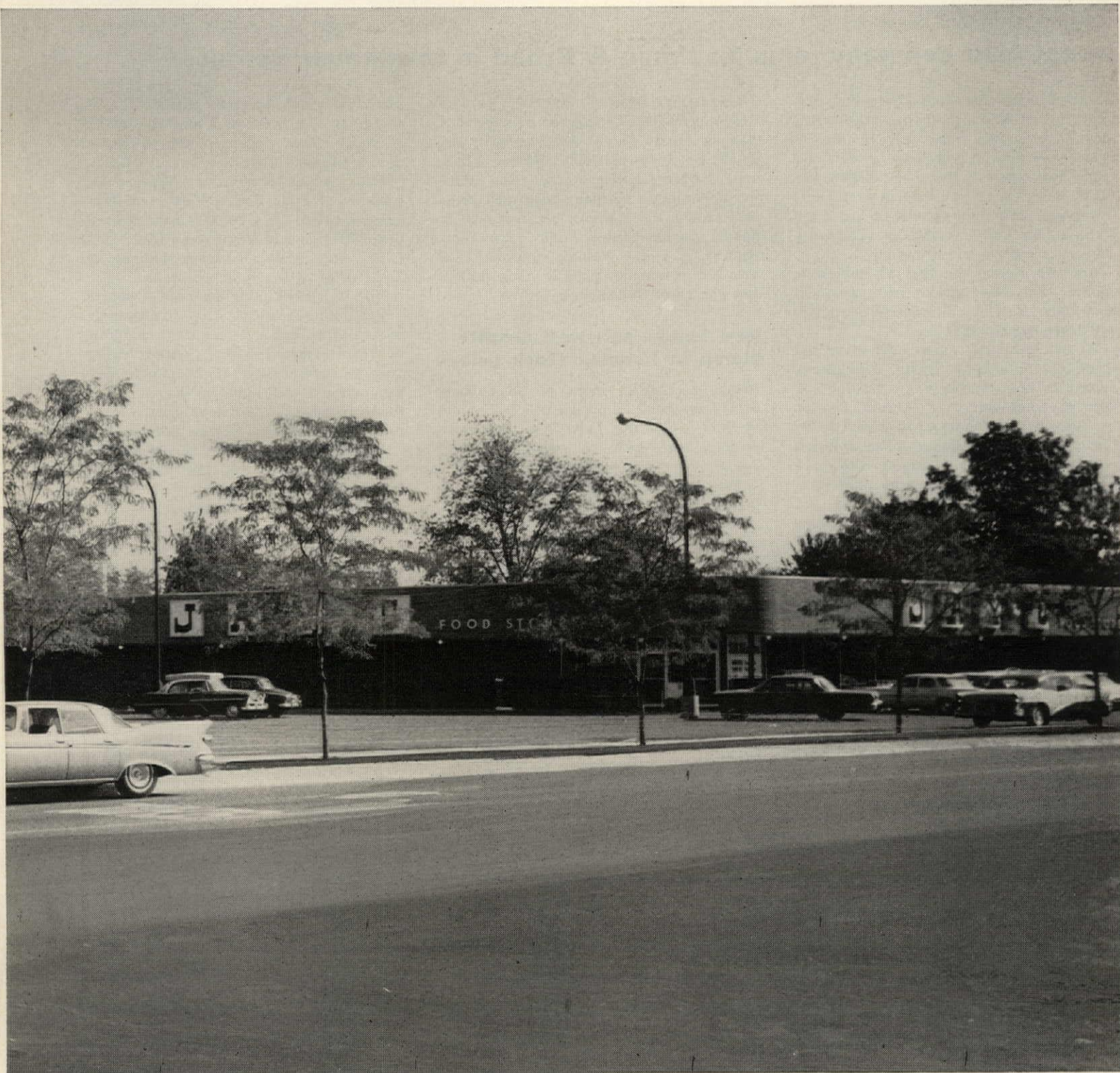
Architects: Harry Weese & Associates. Owner & General Contractor: Repp & Mundt. Bryant Dealer: W. A. Thomas
