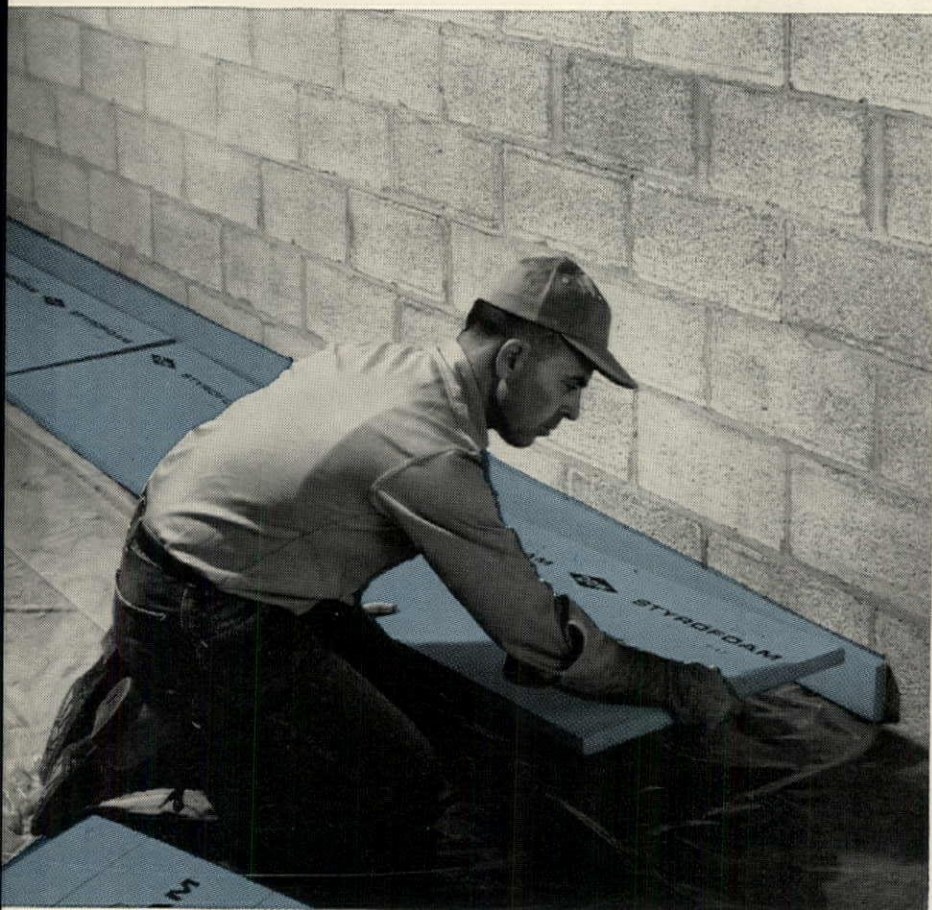
Remember Styrofoam for slabs and foundations.
