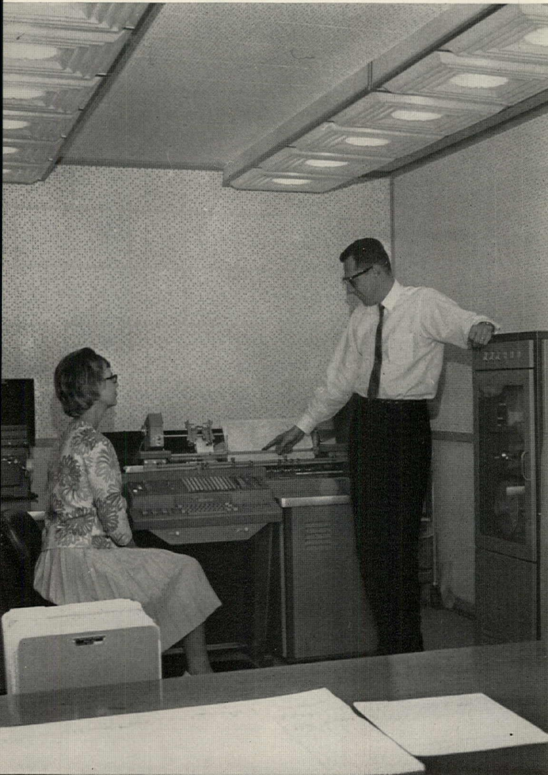
Computer at center is fed data from tape reader at right.
