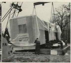
2. STEEL CRADLE, suspended from lifting yoke by cables, lets crane unload house from trailer and position it on prebuilt foundation.
