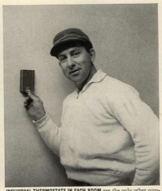
INDIVIDUAL THERMOSTATS IN EACH ROOM are the only other components needed to complete an electric ceiling cable system. A strong selling point with prospects, they allow homeowners to adjust the temperature in any part of the house separately.
