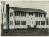
The under-6" pitch on the roof of the house above lacks mass, and the roof overhang is both non-authentic and too small to offer any protection. The 9"-pitch on the Thompson-designed house at the right is in scale and the gutter cornice is both more colonial and less expensive.
