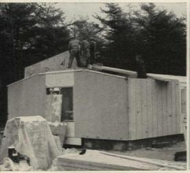
**4. ROOF PANELS** (4' x 15'), stored in attic during transport, are set in place by hand. Shingles or roll roofing finish the job.
