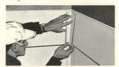
INSTALL METAL CORNERS. Both inside and outside corners slip under siding at bottom, nail at top. Lengths to match siding width. Vinyl color-coated.
