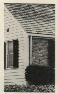
Corner boards should also be used on colonial houses with brick facades (above and drawing, lower left). They hide the narrow end of the brick wall, and do away with the need for careful pointing on the end.
