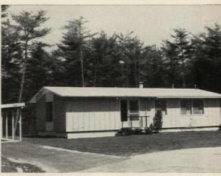
FINISHED HOUSE has trim contemporary lines. Vertical siding can be painted lumber or plywood with polyvinyl fluoride finish.
