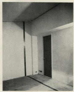
FOLD-OUT HINGES in end wall and floor are continuous, but not in line because floor was folded behind wall. Battens will cover hinges.
