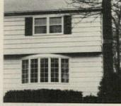
The 12" clapboard exposure above is too wide and out of scale; the 4" exposure at left is —and looks—in scale.
