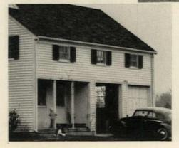
"Shutters must be sized so they would actually fit the window if closed," says Thompson. The drawing at right shows two other basic points: louvers should be slanted so they carry water away from the window when closed; and shutters should be mounted—either by hinges, or by blocking if they are screwed to the house—so there is a drainage gap of at least 1/8" between the shutter and the house.
