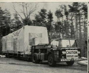
1. TRUCK TRAILER delivers folded but complete house to site. Temporary strapping, under polyethylene, strengthens unit during hauling.
