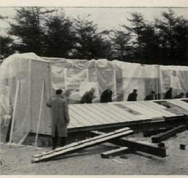
SIDE WALL, hinged to floor, is raised by workers after they have first swung out end-wall sections and then unfolded floor sections.
