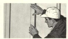
SNAP-ON METAL BATTENS. Fit firmly on clip strips that nail to siding. Available in 8' and 9' lengths, are vinyl coated in colors to match siding.
