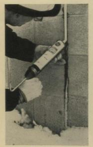
Silicone sealant for expansion joints, glazing and caulking costs about two thirds as much as similar industrial products. It can be used at sub-zero temperatures, cures to form a durable seal that remains flexible. G. E., Waterford, N. Y. For details, check No. 22 on p. 203
