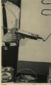
**All purpose mastic** is used for laminating wallboard, paneling, bonding foam insulation and as a stud adhesive. Black Stuff forms an immediate and lasting bond. It comes in cartridges, quarts, gallons and 5-gallon pails. H. B. Fuller Co., St. Paul. For details, check No. 25 on p. 203
