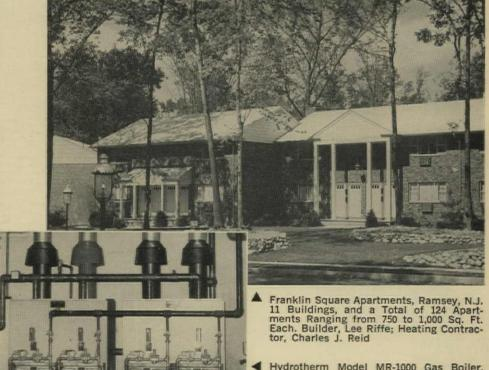
Hydrotherm Model MR-1000 Gas Boiler, 1,000,000 BTU/hr Input is Used to Heat a 24-Unit Apartment Building Totaling 21,000 Sq. Ft.
