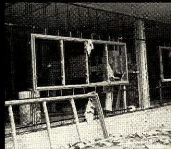
Then Keymesh Paperbacked lath is applied.
