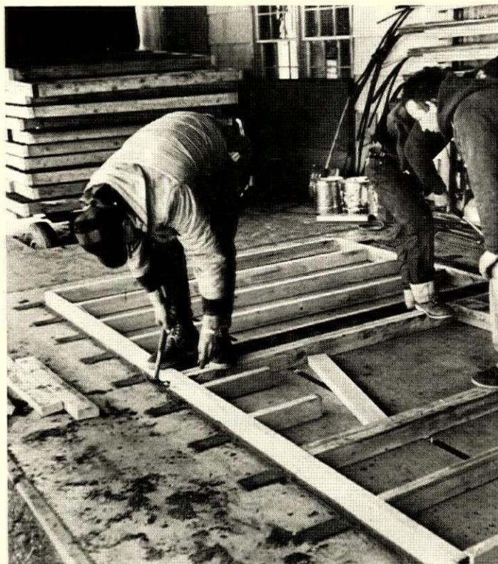
$105 PANEL JIG is made of angle irons that are gunned into the slab ( below ). Marked steel straps are panel templates; laid in the jig, they mark positions for each stud and for the window and door openings.
