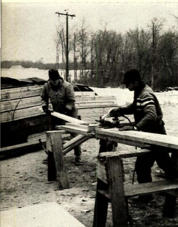
$9 CUTTING JIG has wooden guides ( below ) which hold a standard power saw. Guides are bolted to a long plywood table ( above ) which has a 2x4 side guide. Adjustable stop is held with a C-clamp. Cost does not include saw horses.
