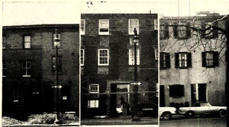
FIRST JOB (shown before, during and after remodeling) is a good example of remodeling mistakes that lose money. Roof was raised, fenestration revamped, floor levels changed—all too expensive. Arcade through building leads to interior court onto which ten houses open.
