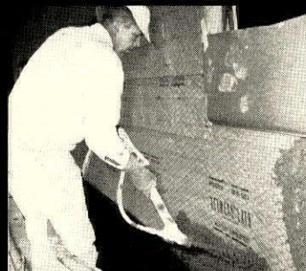
Cement trowelled prior to application of finish coat.
