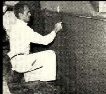
Cement trowelled prior to application of finish coat.
