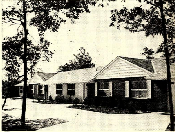
NEW JERSEY CONDOMINIUM project of attached one- and two-story units priced at $12,500 to $18,500 is first big retirement community in the East. Robilt Inc. plans 5,000 units.
