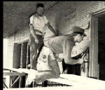
Portland Cement is sprayed on.
