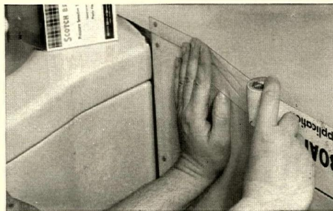
4. After nailing, cover joints with vinyl tape.
