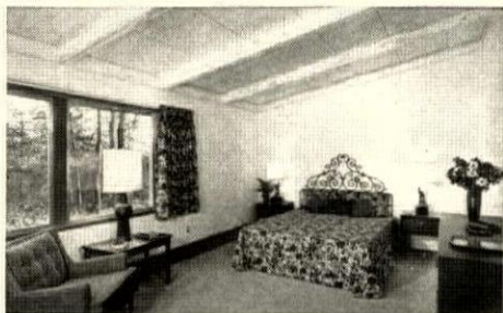
BEDROOM CEILING is underside of roof deck.
