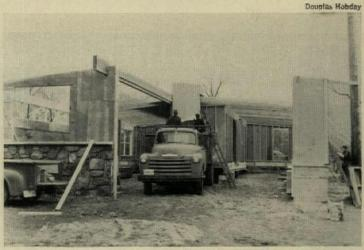
HOUSE is built after core is set on foundation (see below). If rafters rest on core, a roof box beam spanning the end posts is included in core.
