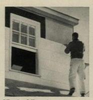
Vinyl siding has a ten-year, maintenance-free guarantee. IVBS is applied without special tools (package includes all accessories). Styles: horizontal lap 12" wide and 16" long, vertical panels 4'x8' and 4'x9'. Four colors. Insulite, Minneapolis.
