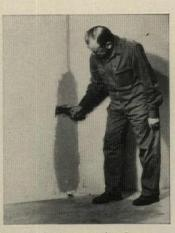
Movable drywall system without exposed seams unzips for room layout changes. A high-tensile, self-adhesive, waterproof tape is the zipper. Joint is easily retaped in its new position. Penn Metal, Parkersburg, W. Va. (For details, check coupon No. 24 on p. 198)
