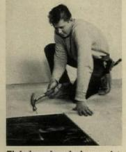
Flakeboard underlayment is available in  $\frac{3}{8}$ ",  $\frac{1}{2}$ ",  $\frac{5}{8}$ " and  $\frac{3}{4}$ " thicknesses, can be used under tile, sheet goods and carpets. It complies with FHA UM-28 floor underlayment specs and with CS236-61. Collins Pine Co., Chester, Calif. For details, check No. 31 on p. 198
