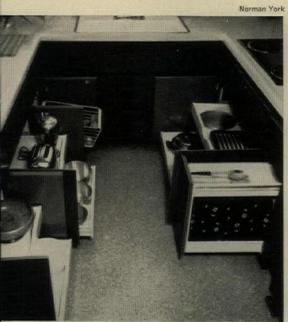
**12** Sliding drawers in kitchens, like these in John Long's Phoenix houses, are featured by 10% of the builders. The extra cost over shelf-bracketed cabinets is less than \$15. Heavy-duty sliding drawer hardware costs \$4 per base cabinet, or \$20 for the five in this kitchen. The hardware will support as much as 100 lbs. when the drawer is fully extended. It is installed simply with screws at the sides.
