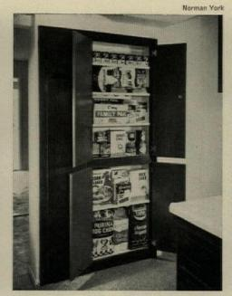
**13** Kitchen pantries are making a strong comeback: 42% of the builders sampled now offer them. The one shown above in a John Long model is framed easily—shelves are built into a partition thickened for this purpose. Doors are prefinished plywood, shelves are pine, and the total cost is about \$25—low for this much shelf space compared with square-foot costs of other kitchen storage.
