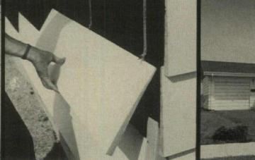
Siding clips are nailed into the wall sheathing with a rubber-headed hammer. Sheathing is butt-joined for a snug fit—a constant feature of UNICOM construction. From the foundation to the finished home, the UNICOM house is solidly built, easily constructed, made to assure fewer callbacks and better business for you.
