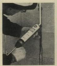
Silicone sealant for curtainwalls, precast concrete, expansion joints, and window glazing is applied from a caulking gun without mixing. It resists temperatures to 250F, can be applied in below-zero weather. \$26 a gal. in bulk. G. E. Waterford, N.Y For details, check No. 32 on p. 165
