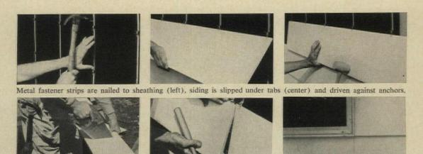
At joints, siding is sawn (left), set into extra fastener strip (center) after edges are painted. Joint is wiped with paint.
