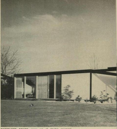
**DISCIPLINED DESIGN** grows out of Alside's structural system. Steel frame, painted black, supports wall panels.
