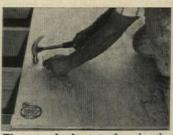
Floor underlayment, a sheathing-grade plywood, has a solid veneer sheet under the face veneer. Since there are no voids under the face veneer, damage from spike heels and heavy furniture is eliminated. Vancouver Plywood, Vancouver, Wash. For details, check No. 9 on p. 165
