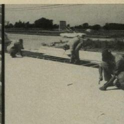
UNICOM board subflooring, delivered pre-cut to standard uniform modular length, is quickly and accurately laid down to provide you with a sturdy, lasting deck.
