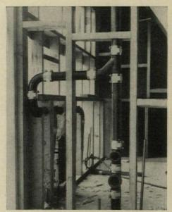
Hubless cast iron sanitary systems are covered in two reports. The first describes the new no-hub system of joining cast-iron pipe and fittings in drain, waste, vent, and sewer systems. It allows 2" and 3" pipe to be run in a wall with 2x4 studs. This 44-pager includes complete specs and shows typical installations. The other booklet is a 36-page report by the Pittsburgh Test Laboratory on results of its investigation of the system. Cast Iron Soil Pipe Institute, Chicago.
