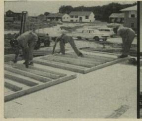
Carpenters use the open deck area as a convenient and uncluttered table to assemble wall components from pre-cut UNICOM parts delivered to the site.
