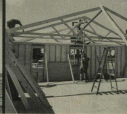
A notched gin pole moves a truss into position for the UNICOM house. W trusses provide free-span area below, obviate load-bearing interior partitions.
