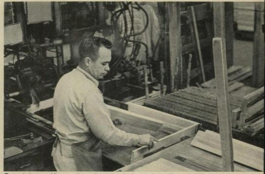
6 precisely assembling complete units-automatically squaring, nailing and drilling holes for ...
