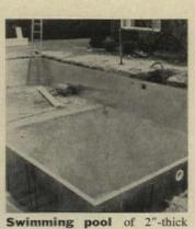
aluminum sandwich panels is assembled in an excavation. Package includes steel channel, vinyl liner, aluminum coping, plumbing and filter system. A 16' x 32' pool costs \$995 as a kit, \$1,995 installed. Trojan Pools, Troy, N.Y. For details, check No. 23 on p. 165
