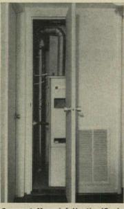
Compact Moncrief Heating/Cooling Components require as little as 2 square feet of floor space.
