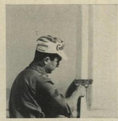
**TAPE BEDDING** is done with hand knife: fast drying material may clog automatic equipment.
