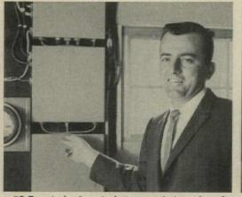
"G-E motorized controls turn a whole series of preselected circuits ON or OFF when you press one of the entranceway switches. Lights can also be controlled locally. Low-voltage wiring lowers the cost of extra switches.
