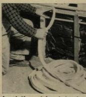
Insulation strip, designed to cut labor cost of caulking around doors and windows, is simply pushed between studs or sills and door or window frame. Bonded cellulose fiber strip is 3/4"x11/4", comes in 50' rolls. Wood Conversion Co., St. Louis.
