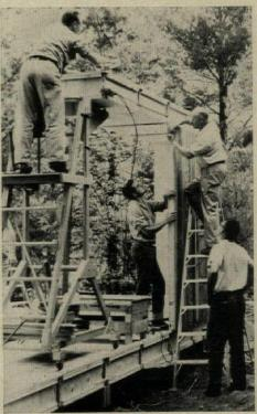
WALL AND ROOF PANELS go up together. Clamps align panels for stapling and lag bolting.
