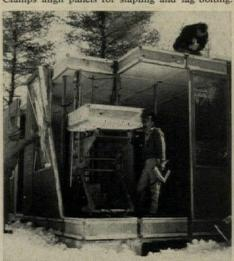
LIFT raises roof panels into position, Fascia panels finish roof and floor.
