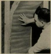
Mineral-wool insulation is made slightly oversize for fast fitting between studs. When blanket is pressed in place, the spring-back of the mineral fiber holds it without stapling. Sizes: 15" wide, 4' and 8' long, 2", 3", and 35%" thick. Celotex, Chicago.
