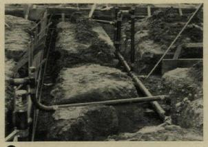
NO HUB piping goes underground! We recommend the new "Hubless Cast Iron Sanitary System" unqualifiedly for under-floor drains. The neoprene sleeve joint resists abrasion, is flexible and leakproof. Roots can't penetrate it. Heat and acidy soils don't affect it. The stainless steel shield and clamps are highly corrosion resistant to outlast the ordinary life of residential structure.
