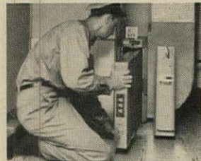
Easily installed in new or existing homes, with little interruption of heating or cooling.
