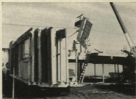
MOTEL WALL SECTIONS , loaded on truck in erection sequence, are placed by crane.
