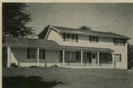
IN NEBRASKA: "Builds our reputation for quality." Lippold Construction Co., Omaha
