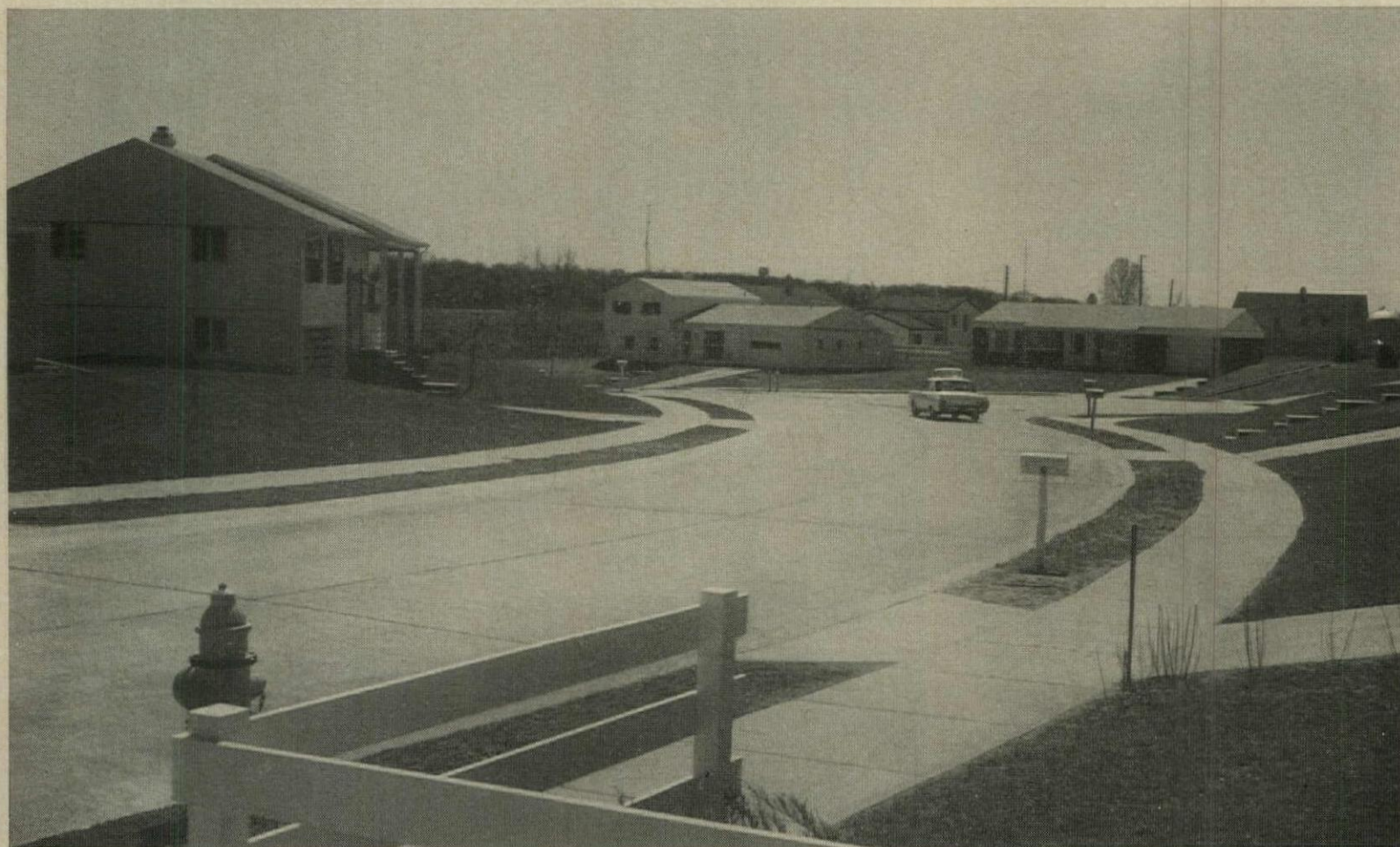
A new concrete street with integral curb and gutter in Riverside Manor, South Bend, Indiana
