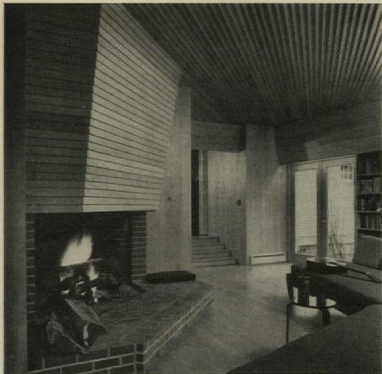
Wood achieves a distinctive pattern effect in this living area, where the entire ceiling and much of the paneling are installed like bevel siding. A clear finish is used throughout the room to expose the natural variations of tone and grain.
