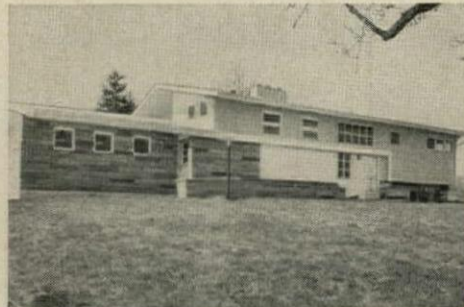
IN OHIO: "Our carpenters like to work with it." Sims Bros. Inc., Marietta
