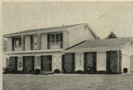
IN OHIO: "Reversible edges help us eliminate waste on gable ends." Smith-Kettler Bldrs., Inc., Cincinnati
