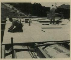
Flooring is 2-4-1 plywood, nailed to create a monolithic diaphragm floor that acts as a rigid brace for the entire support system.
