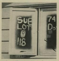
oped a masking agent that can be sprayed, brushed, or rolled on. It peels off glass (above) or metal, taking slop-over spray with it, but it sinks into wood or gypsum and acts as a sealer. Another big builder now dips all his hardware in the material before mounting it, paints right over the hardware, and then peels off the coating.
