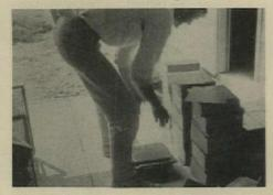
able on the floor, most installers mix tiles from various boxes (above). Asked the TAMAP engineers: Couldn't some way be developed to prevent sticking? And couldn't tiles of the same color from various production runs be mixed in the plant?
