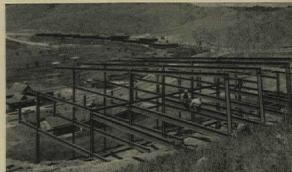
Skeleton view shows four sloping bents that form carport roof, then sweep down house to add ceiling height in the living area.
