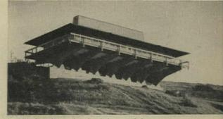
Uphill view shows the visual drama of the structural system. Underside of the floor is finished with curved plywood hiding utilities and insulation. *continued*
