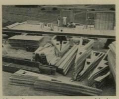
After walls were up, trusses were erected in three sections: outriggers (shown stacked), W-trusses, and vertical trusses (see section drawing, right).
