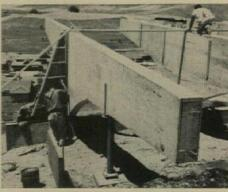
Triangular lateral braces, over wall, and pipe columns, foreground, carry no load. They resist horizontal forces, unequal loading, and rotation.
