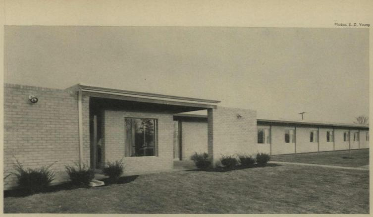
ONE-STORY BUILDING is slab-on-grade construction, perfectly familiar to builder's regular subcontractors. Windows are stock aluminum units.
