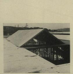
Roof panels on both flat and peaked areas are stressed-skin plywood, with decorative wood inner faces. Wall framing is conventional post-&-beam.
