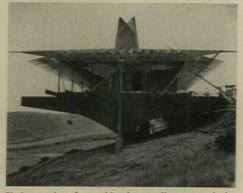
Skeleton view from side shows all structural elements from concrete foundation wall to the vertical trusses that form the rooftop plenum.
