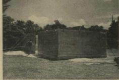
**SIDEWALLS** of paper honeycomb with aluminum skins are fastened to sill (detail lower right).
