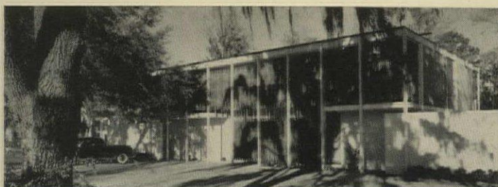
Street facade (above) presents the same interesting, but closed, appearance to the street as the rear elevation (left) does to the view side. Steel H columns are on 6' centers, exposed and painted white throughout. Solid second-floor sidewalls are weathered redwood paneling.
