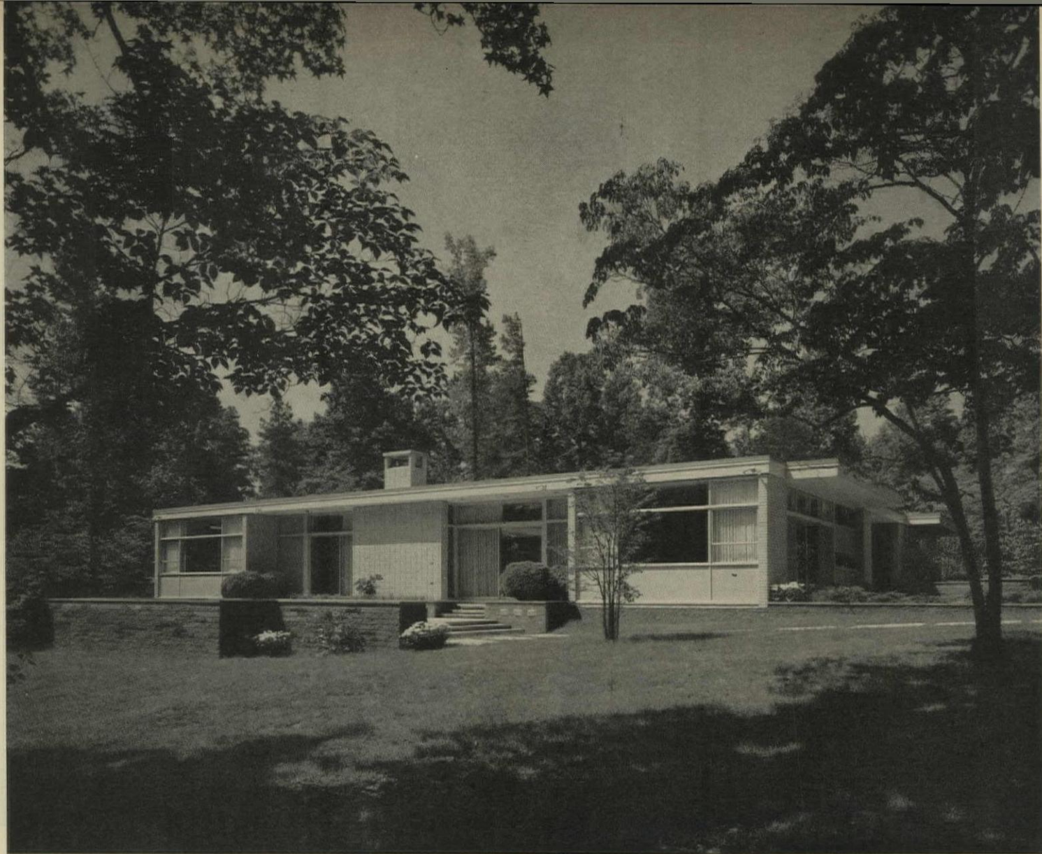
Living terrace gains privacy (and a better view) by perching on a filled embankment which rises as much as 7' above grade.
