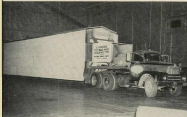
TRUCK delivers 10' x 44' house package to climatic test hangar at Eglin Air Force Base.
