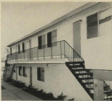
GARDEN APARTMENT was built by Guaranteed Homes, Costa Mesa, Calif. on by-passed urban site. More than half of Guaranteed's business is in rental units.
