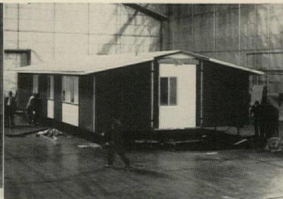
FINISHED HOUSE is 26' wide, rests on four wood beams supported by adjustable steel legs.
