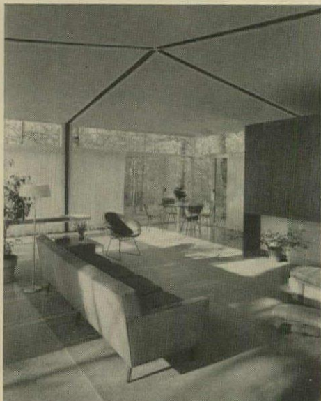
In living room, fluorescent lighting trough and skylight are formed by divided roof girders. Daylight is filtered through plastic and gray glass.
