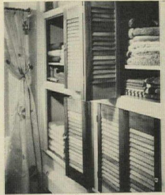
SHUTTERED STORAGE UNIT is just deep enough for folded towels and adds warm look of wood on the wall away from water.
