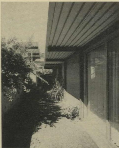
Sheltered court is formed between house and uphill retaining wall. View is from bedroom patio toward outdoor dining area at far end.
