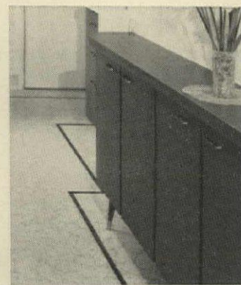
WALL CABINETS , mounted on legs, provide shallow storage in a kitchen too narrow for full base cabinets on both walls.
