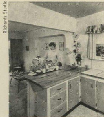
DIVIDER-SNACK BAR in new wall between kitchen and dining room has counter top made of prefinished hardwood strip flooring.
