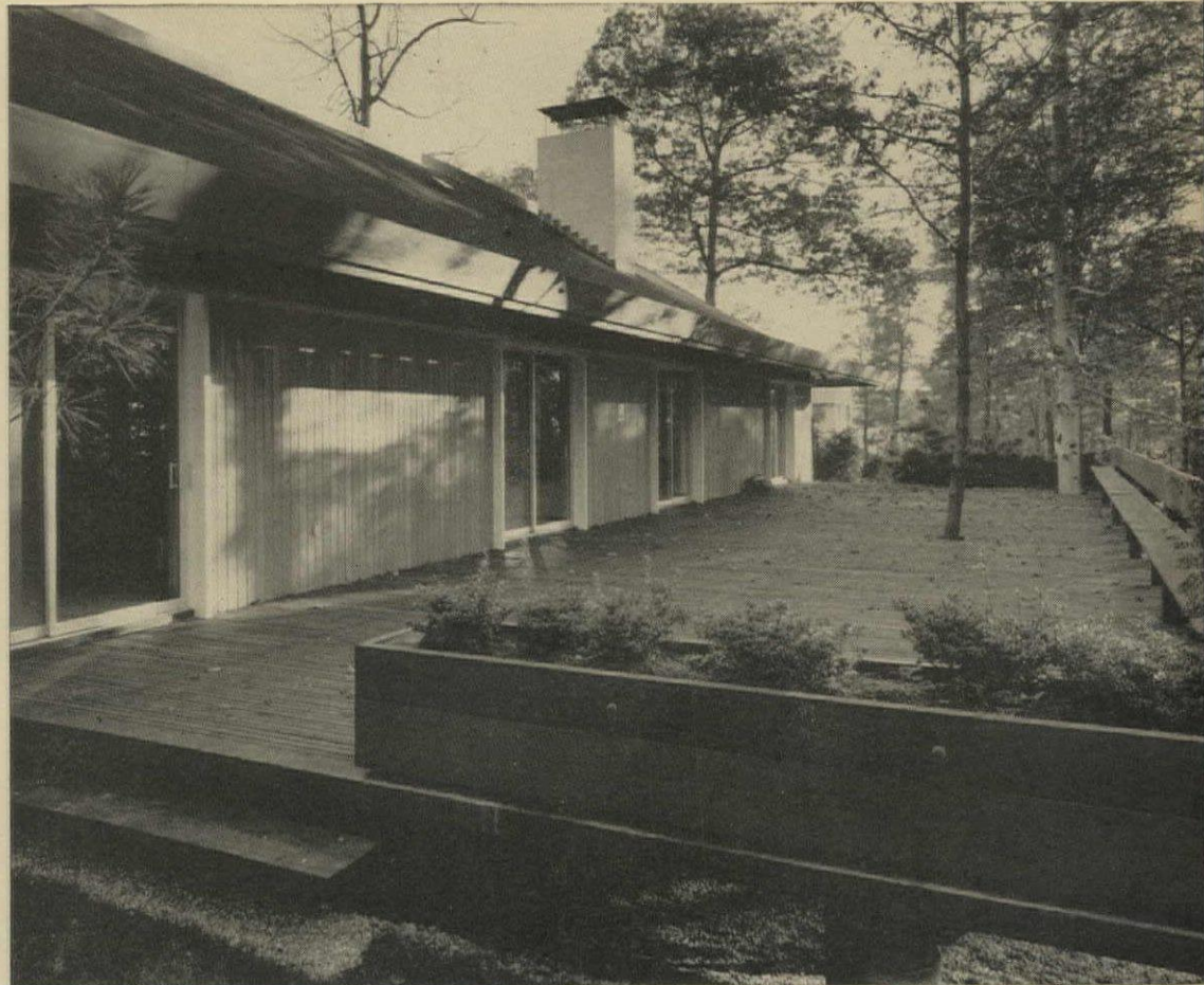
Rear deck, built up from grade, is well protected from view in all directions. A wood banquette extends full width.
