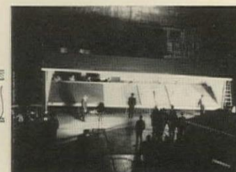
5. To raise sidewall, crew steps inside house and manually lifts wall to vertical position. Lag bolts make all connections fast.
