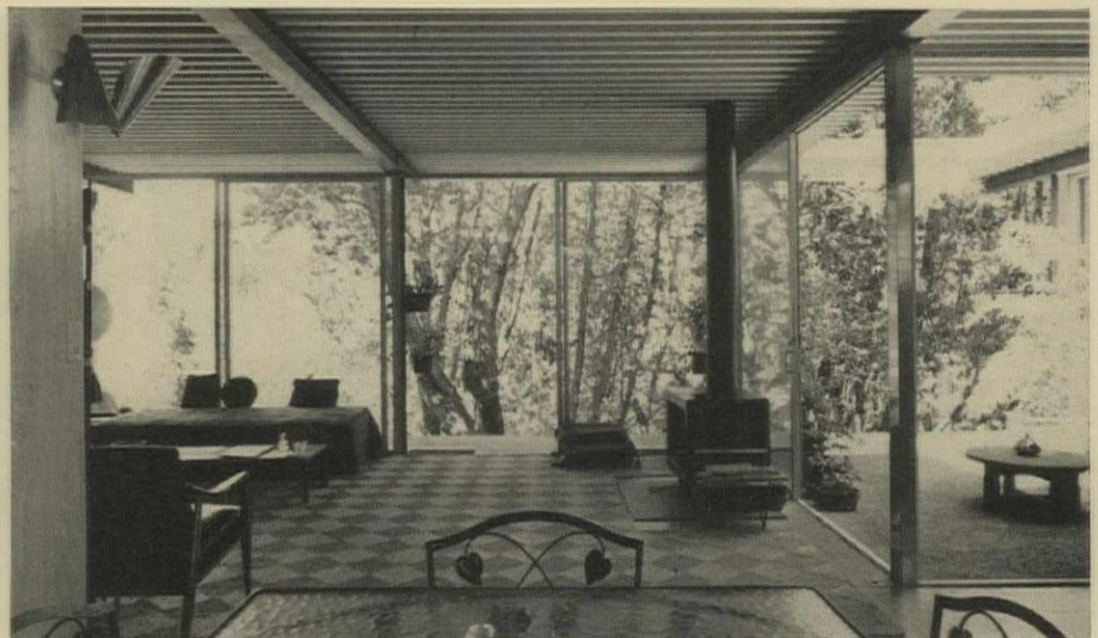
Structural system—steel posts on a 10' module—eliminated bearing walls. So walls are mostly big sheets of sliding glass doors. Opaque walls are
