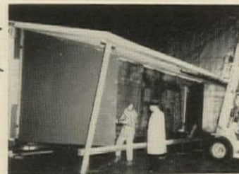
3. Side walls are folded out from under roof. Joint between roof and sidewall is then weather-sealed with urethane foam gasket.
