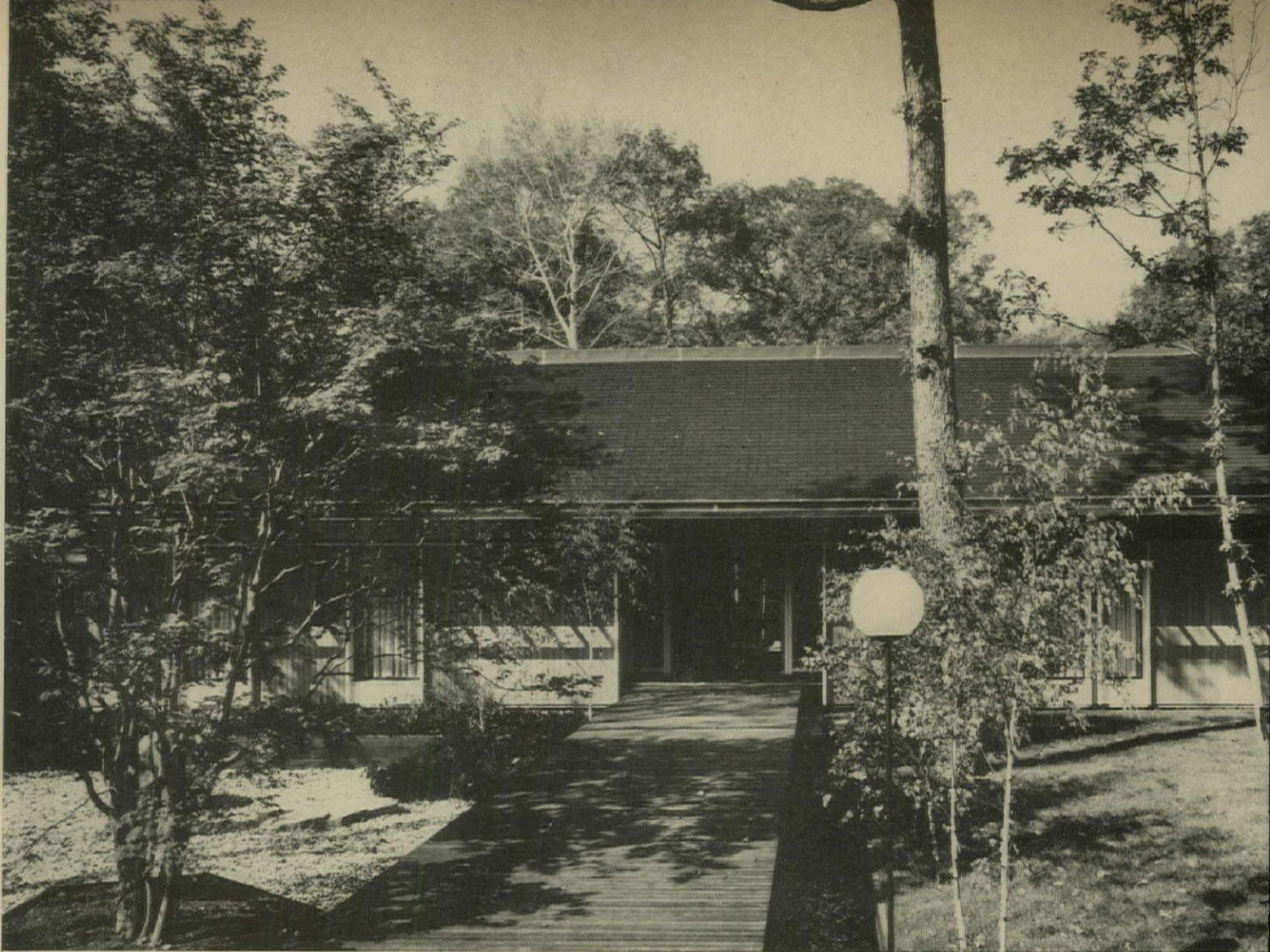
Pitched roof and wood exterior were used to harmonize with the existing neighborhood of development houses. Landscaping is formal.
