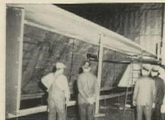
4. Floor panel is gently lowered by roller for forklift. In the field a gin-pole and chain hoist will lower floor to outside floor beam.
