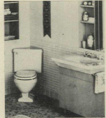
CORNER TOILET with triangular tank can solve space problems in either too-small bathrooms or in powder rooms.
