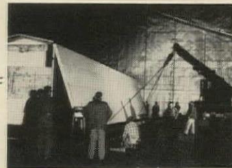
2. Crane lifts one side of roof first. House was erected in test hangar where it would be subjected to 65 F. below zero.
