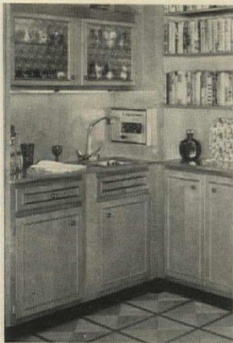
BAR SINK can be assembled from standard kitchen components. But costs can skyrocket if a new plumbing stack is needed.
