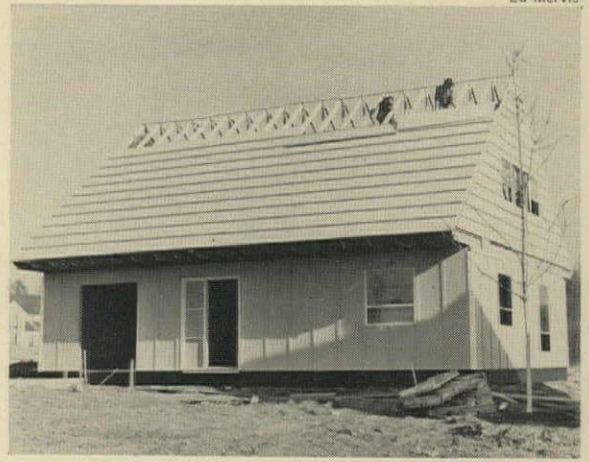
RESEARCH HOUSE has prefinished board-and-batten sheathing-siding, new Bermuda roof system of prefinished plywood sections.
