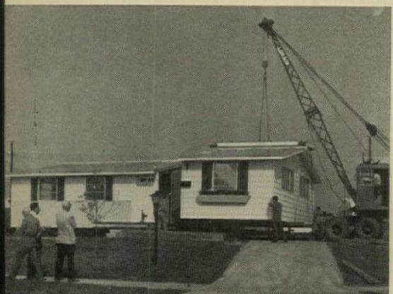
. . . Last section swings in at 10:30 A.M. Asbestos-cement skirt is attached, utilities hooked up. House is finished at 2 P.M.
