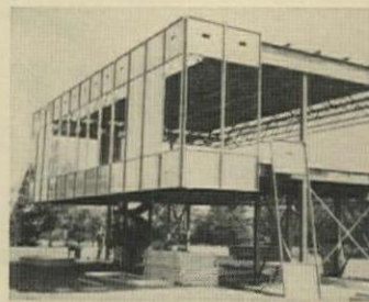
NEXT DAY: All curtain wall panels are locked into place.
