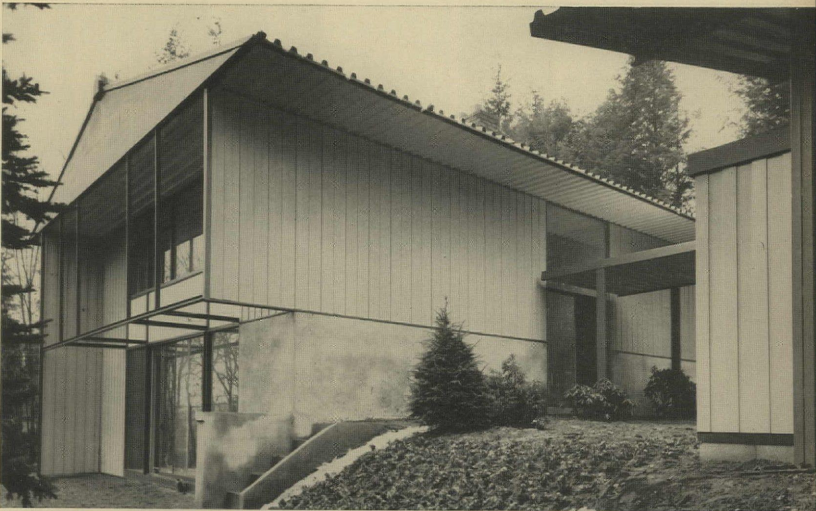
PROTOTYPE STEEL HOUSE is a modified Techbuilt. It is 28' (instead of the normal 24') wide because of greater spans possible with steel.
