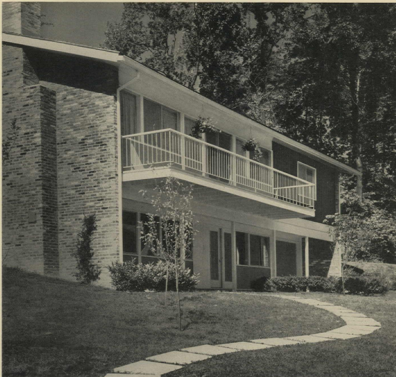
The Overlook, one of six models, has four bedrooms, three full baths and recreation room. Outside, a balcony, covered porch and patio make the most of the wooded, rugged terrain. All homes at Carderock Springs were designed by Keyes, Lethbridge & Condon, A.I.A.
