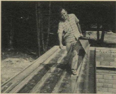
FLOOR PANELS are 16" wide, 3" deep, have interlocking edges, are made of 20-gauge galvanized steel. Channels serve as heating ducts.
