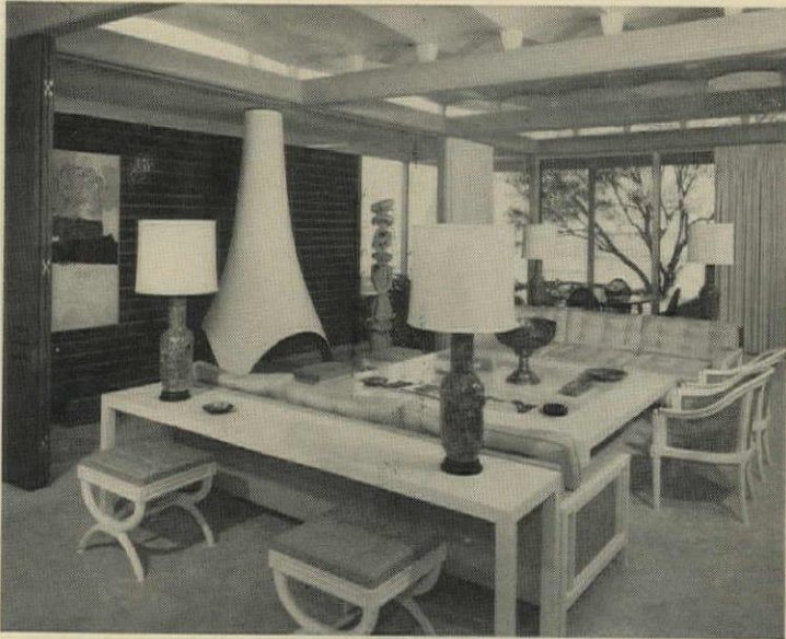
LIVING ROOM (D) has ceiling formed by exposed underside of concrete vault roof. Steel girders, topped by blocking, carry vaults which have clear span of 10'. Ceiling height is 10' except over fireplace at left.
