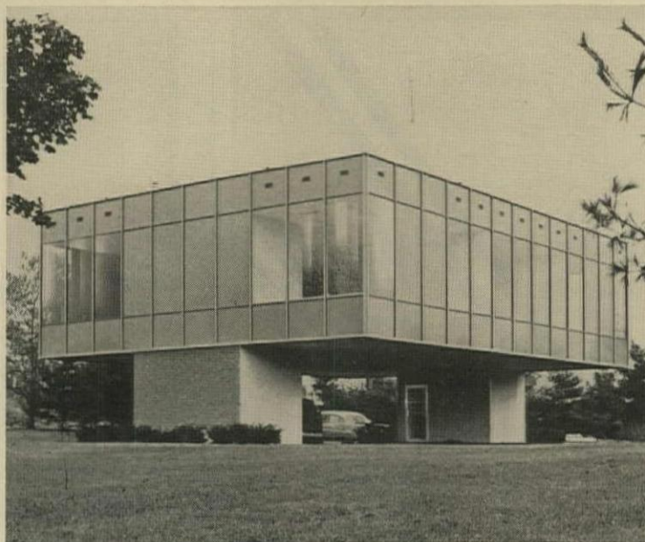
PROTOTYPE MODEL of steel prefab is a 52' x 40' off-the-ground building on two bases. Stairwell is in one base, mechanical equipment in other.
