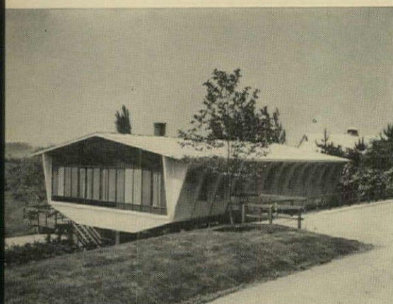
FORERUNNER HOUSE had wood space frames extending beyond side walls.
