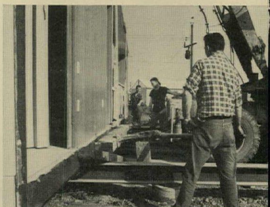
. . . 20-ton crane starts placing first of three sections on foundation at 8 A.M. Jacks push sections together on beams . . .
