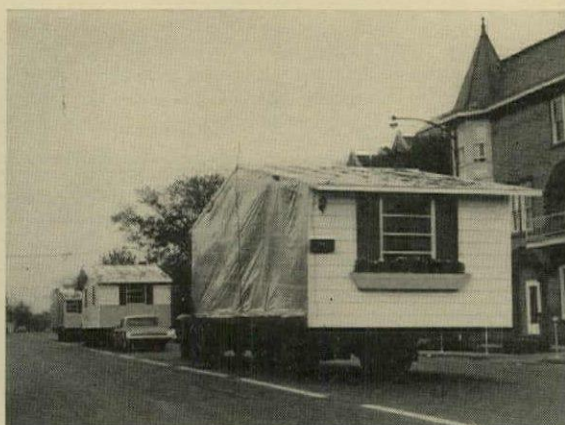
House sections leave factory at 6:30 A.M. and are trucked to site where I-beam foundation and front steps await them . . .
