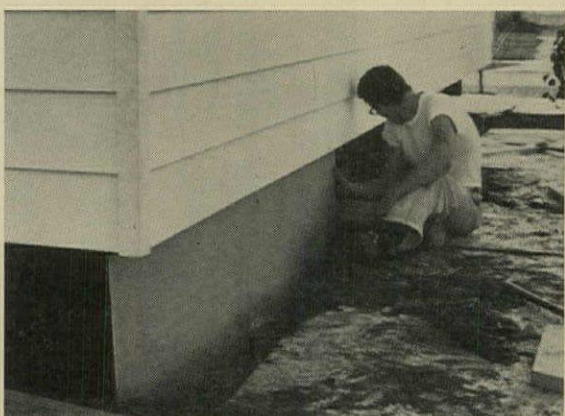
. . . Last section swings in at 10:30 A.M. Asbestos-cement skirt is attached, utilities hooked up. House is finished at 2 P.M.
