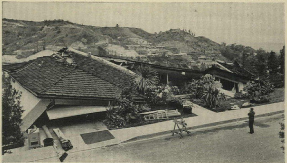
SLIDING HOMES in Los Angeles' steep Brentwood section are bringing renewed cries for stricter subdivision and building rules for homes built on cut and fill. City council probes are
