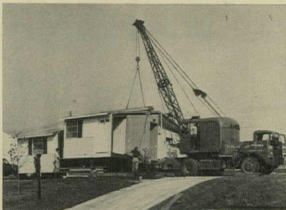
. . . 20-ton crane starts placing first of three sections on foundation at 8 A.M. Jacks push sections together on beams . . .
