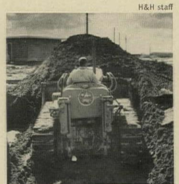
BIG BULLDOZERS carve out basement excavations. Power shovel is not needed since soil is sandy.
