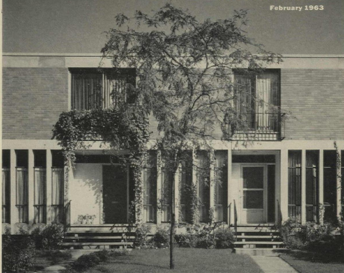
Townhouses in Hyde Park-Kenwood urban renewal area, Chicago. Architects: Harry Weese & Associates. Builders: Webb & Knapp
