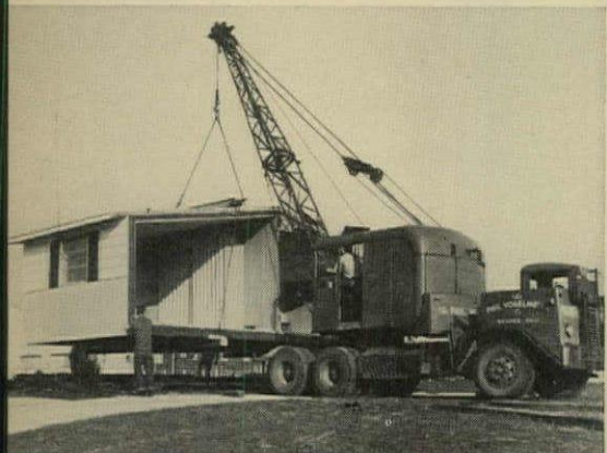
. . . 20-ton crane starts placing first of three sections on foundation at 8 A.M. Jacks push sections together on beams . . .
