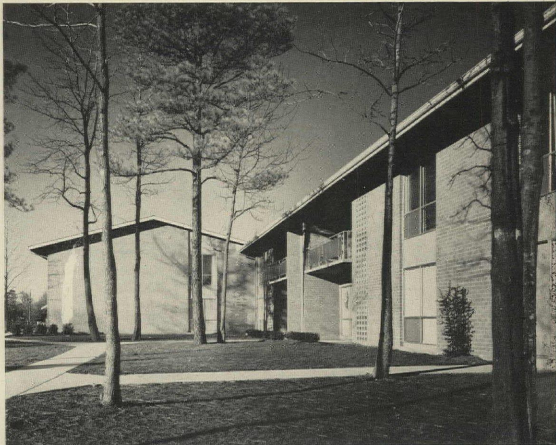
SETBACKS avoid monotonous building placement, create pleasant courts. Deep overhangs shade balconies, minimize sun load and air conditioning cost.
