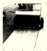
**One-ply roofing,** called "Last-O-Roof," is made of polyisobutylene welded to an elastomerbonded asbestos support. It is applied with cold adhesive, can stand up to any climate. Johns-Manville, New York City. For details, check No. 185 on p 219
