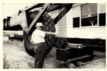
**3. LIFTING BEAM** at rear of housemover raises house, which still rests on steel channels, off I-beam dollies. Space between end-to-end dollies gives beam clearance. Housemover can lift load 4' off ground.
