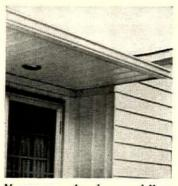
**V-groove aluminum siding** can also be used as a soffit system, as shown above, is supplied in plain and ventilated panels. It is available in white and four pastel colors. Mastic Corp., South Bend, Ind.
