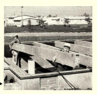
FOR BOTH SYSTEMS, supports may be solid or built-up beams or, as on this Insta-Floor job, plywood box beams for long span, light weight, low cost.
