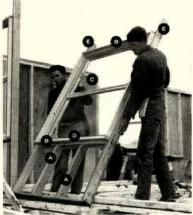
THIS IS THE STRUTWALL! A complete, factory-assembled package adaptable to any construction need. Jack studs (A), top and bottom nailers (B), glazing (C), hardware (D), and side struts (E) are factory installed . . . permits faster job enclosures. Removable grilles, paint priming, plywood box headers and sheathing to fit your needs are factory options.
