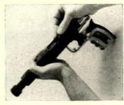
**Piston-type gun** drives fastenings into work at low velocity. Blank cartridge drives the piston which in turn sets the fastener. Unit weighs 4½ lbs. Winchester-Western Div., Olin Mathieson Chemical Corp., New York City. For details, check No. 170 on p 219
