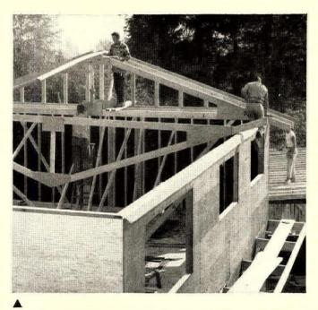
**Bell & Valdez,** large Pacific Northwest builders, used king post trusses in 100 houses during a trial run, then converted all their models to this type. Low cost was the chief reason. Trusses were fabricated by Totem Lumber in Seattle. Totem makes the double-gusseted truss 30 at a time in a special manufacturing process and figures costs at about \$1 less than for a comparable truss with metal connectors.
