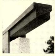
**TOP PLATE**—continuous, rabbeted, and glued snugly between skins ties panels together structurally.
