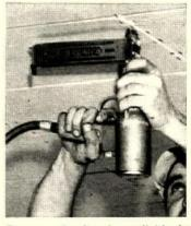
**Power stapler** is available in models that handle staples from 3/8" to 2", and T-nails from 1/4" to 21/2". It operates on air pressures as high as 90 psi or as low as 40 psi. Bostitch-Calwire, East Greenwich, R. I. For details, check No. 174 on p 219
