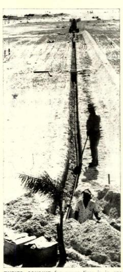
**BURIED CONDUIT** for power lines is in one trench; phone and coaxial cables are separate.
