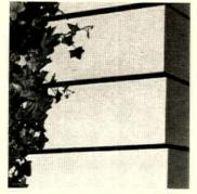
**Prefinished redwood siding** has factory-applied prime coat that gives about half of FHArequired paint thickness. Paint used is an alkyd resin-type primer. Union Lumber Co., San Francisco.
