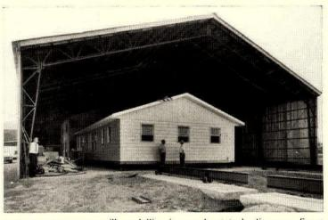
**2. FINISHED HOUSE**, still on dollies, is moved out to loading area. Space between end-to-end dollies will be directly above trench, in foreground, where lifting beam (below, left) will be placed. Factory holds four houses.
