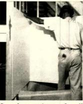
**One-piece waterproof wall** for tub-and-shower enclosure has Micarta surface, foam core, and Micarta backing. It can be installed over studs by one man in an hour. Micarta Div., Westinghouse, Hampton, S. C. For details, check No. 152 on p 219
