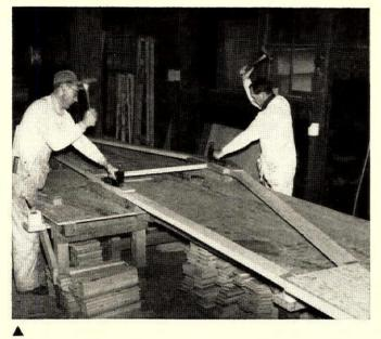
**King post trusses** may have nail-glued or stapleglued plywood gusset plates (as above); or gussets may be pressure-glued; or simply nailed. They're economical because they require only half as many connections as other truss designs. Many component fabricators and lumber dealers supply king post trusses as part of a complete prefabricated house package. Some builders who have used them report savings up to \$300 a house due to use of the prefabbed components.
