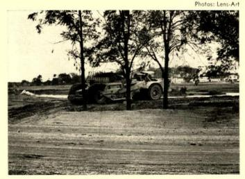
**HUGE SCRAPER**, carrying fill to a low spot, carefully avoids trees that will later be welled. Water in the background forms an artificial lake created to overcome the problem of low, wet ground and to add an important attraction for houses in the \$30,000 range.
