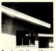
**Board-and-batten siding** is made of %" overlaid exterior plywood with two prime paint coats. Battens are available in 8', 9' and 10' lengths to match plywood sheets. Evans Products Co., Portland, Ore.
