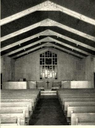
This North Carolina chapel demonstrates the adaptability of the rigid frame. It differs from the usual design in its straight sides-DFPA's construction recommendations for builders include details of this variation. The chapel cost \$6.96 per sq. ft., including masonry, foundation, Texture One-Eleven siding-sheathing and roof of plywood stressed skin panels.
