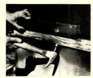
Starter strip with beveled top edge is nailed at bottom of wall.
