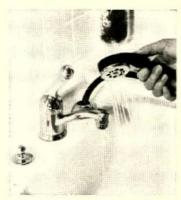
**Spray unit** mounted on flexible pull-out hose permits shampooing in the bathroom sink. Both the spray head and the faucet are operated by the central singlelever control. Delta Faucet Corp., Greensburg, Ind.
