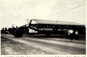
**4. LIMITED ROUTE** of housemover is across highway where phone and power lines have been raised (traffic is stopped for three minutes). Mover makes up to 20 mph, but cannot travel roads because of its width.
