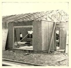
**HEADER** over picture window is section cut from regular panel with power saw. But most windows are cut out of walls after panels are erected.
