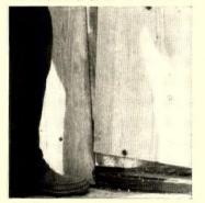
**JOINTS** are formed by slipping grooves of one panel over tongue of next one and over sill.
