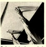
**Embossed lay-in panels** fit into a simple metal grid system. Flame-resistant panels come in  $2' \times 4'$  and  $2' \times 2'$  sizes. Luminous and acoustical panels are also available. Celotex Corp., Chicago.
