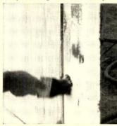
**TONGUE** of t&g panel gets coat of phenol resorcinol glue in field before adjoining panel is erected.
