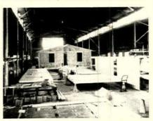
Stationary assembly on work tables is system used at United Factory Bilt, Shreveport, La.
