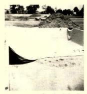
VINYL LINER has beaded edge, snaps into extrusion on wall top.
