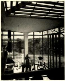
post encased in plaster, center skylight roof.
