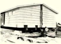
Jacks lower a Del Nero house onto its foundation after sections were rolled into place.
