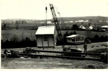
**SPACE FRAME HOUSE** by Building Components Research, Newark, Ohio is made of transverse sections that rest on steel rails (see H&H, Sept).
