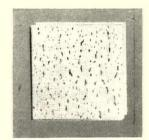
**4.** Hallway ceiling is tiled with a fissured fiber tile. Added cost: \$21.
