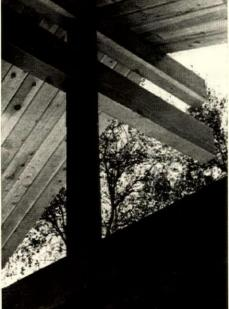
DETAIL shows framing at point where pitch roof over living area intersects flat walkway roof. Top 4x8 is roof ridge; bottom 4x8 was added for additional design interest.
