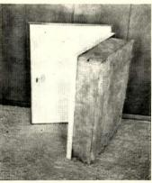
**c.** Two bathroom medicine cabinets (which are recessed in wall) have insulation glued to backs and sides to dampen sound transmission. Added cost: \$2 each.
