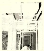
e. Ductwork is made of fiberglass which reduces sound transmission noises from heating/cooling unit and from room to room. (This was already a standard item.)
