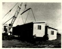
Crane with a cable sling places an American Way house section onto its foundation.
