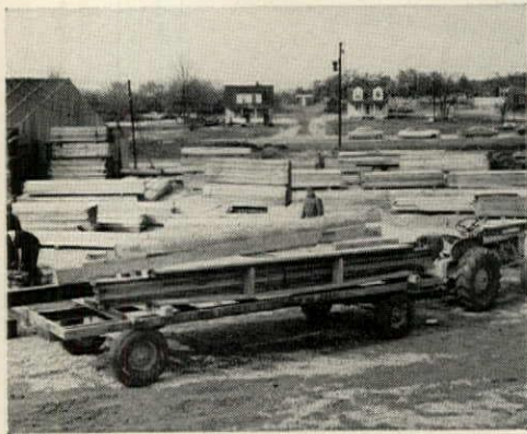
JOIST PACKAGE is first trailer load to arrive from shop, is steel strapped for easy handling.
