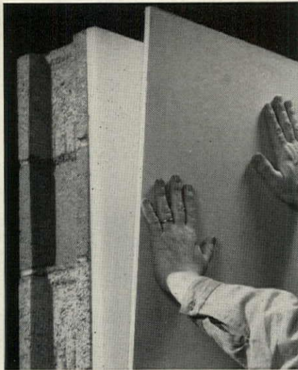
5. Press wallboard into place.
