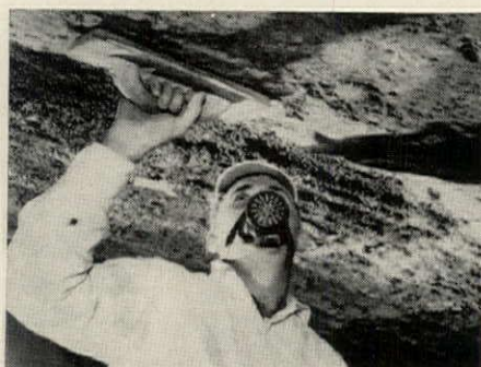
ASBESTOS INSULATION is sprayed 1" thick on 2½" concrete shell. Troweling smooths finish.
