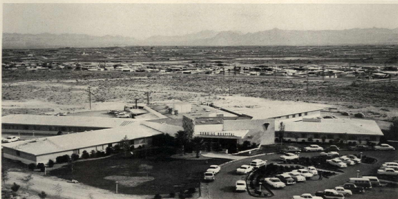
130-BED HOSPITAL was built as an investment by Merv Adelson and Irwin Molasky of Las Vegas, who used their own homebuilding crews on the job. It cost $2 million (including land and $600,000 in
