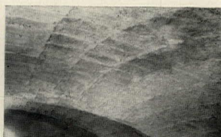
INFLATED FABRIC , held down by cables, serves as form for concrete sprayed from below.
