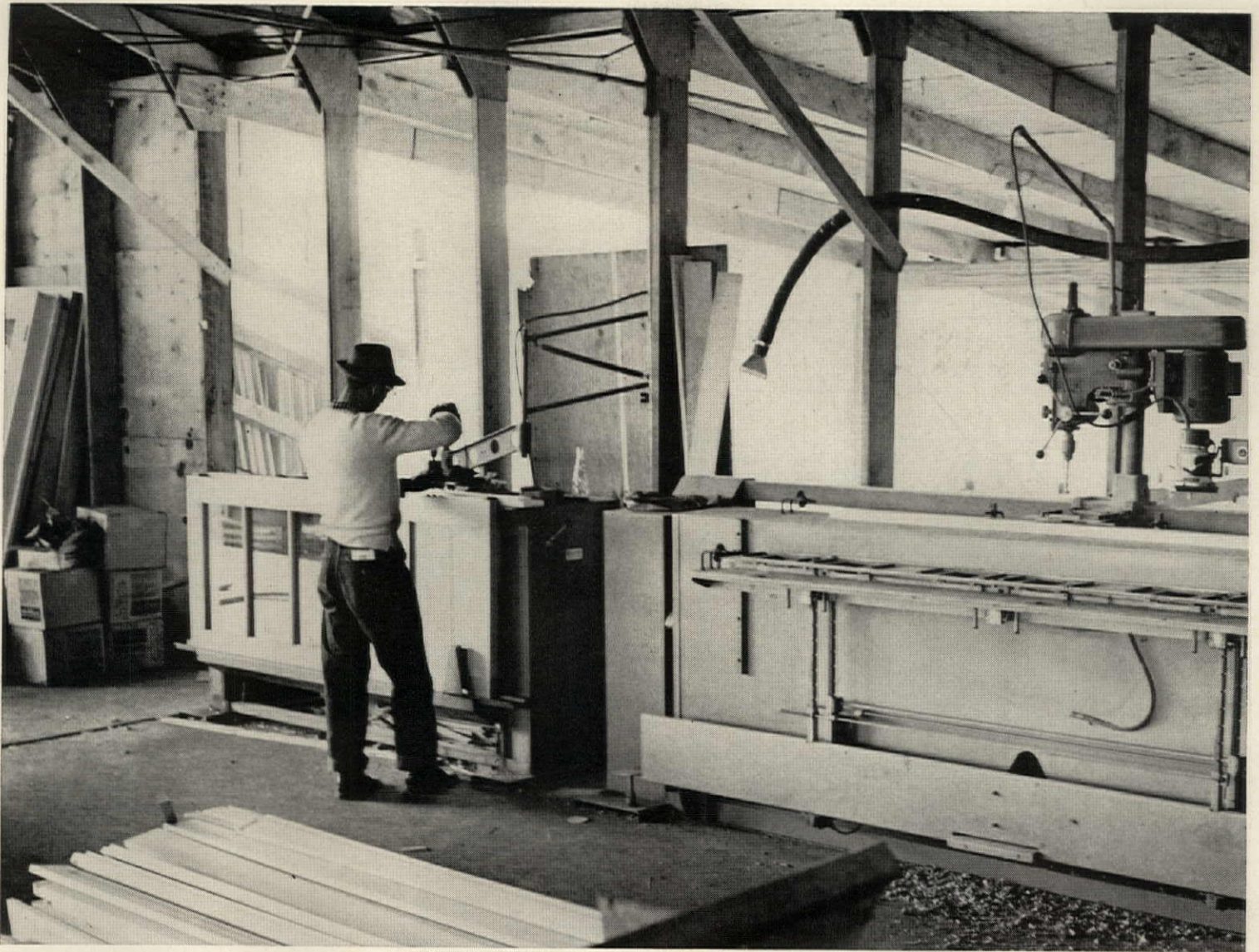
DOORS AND FRAMES are made up into prehung units in roofed-over shop area. Door and window frame parts are milled to size on saws and jointer (foreground), then prime-painted (photo below). All millwork for one house is delivered to site on one trailer, after shell is erected.
