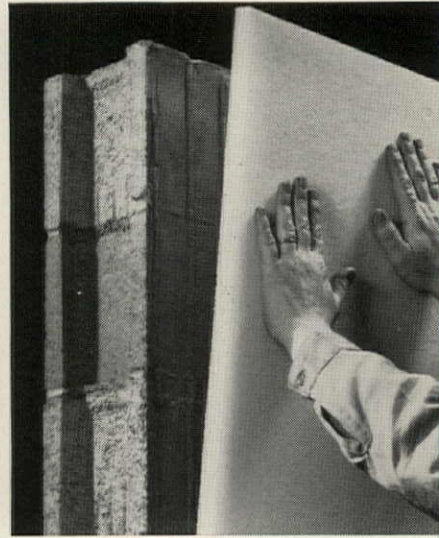
3. Press Styrofoam® into place.
