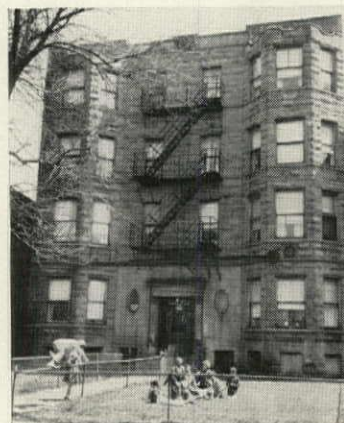
FLATS AT 6527 S. KIMBARK Inspectors found 171 violations
