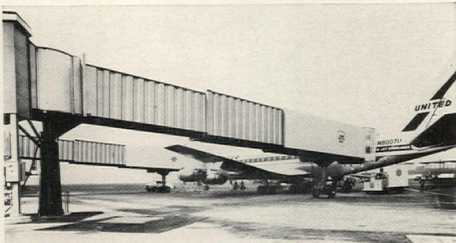
LOADING RAMP, 115' long is made of three telescoping box beams with 14-gauge webs
