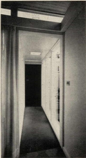
BRIDGE connecting modules is glass-walled, has electric radiant heating.
