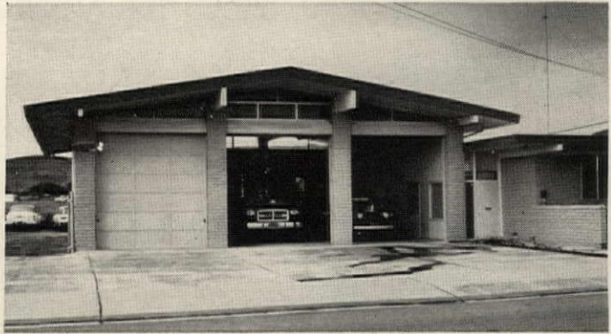
FIRE STATION in San Ramon, Calif. was built by Volk-McLain, a homebuilding company which has built schools and a shopping center.
