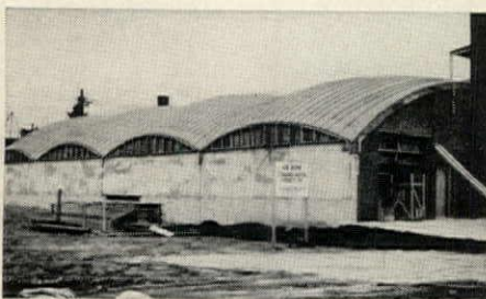
INFLATED FABRIC , held down by cables, serves as form for concrete sprayed from below.
