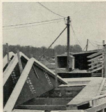
GABLE OVERHANGS are pre-assembled and attached to sheathed gable ends. These assemblies are delivered to site on trailer with wall panels.
