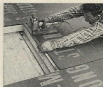
PRECUT SHEATHING is nailed to the framing on the jig table.
