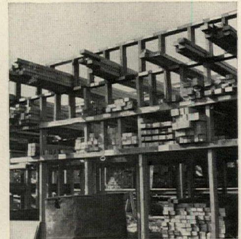
STORAGE BINS are open on both faces. Precut lumber is fed in one side (previous photo), withdrawn from the other side (see opposite).
