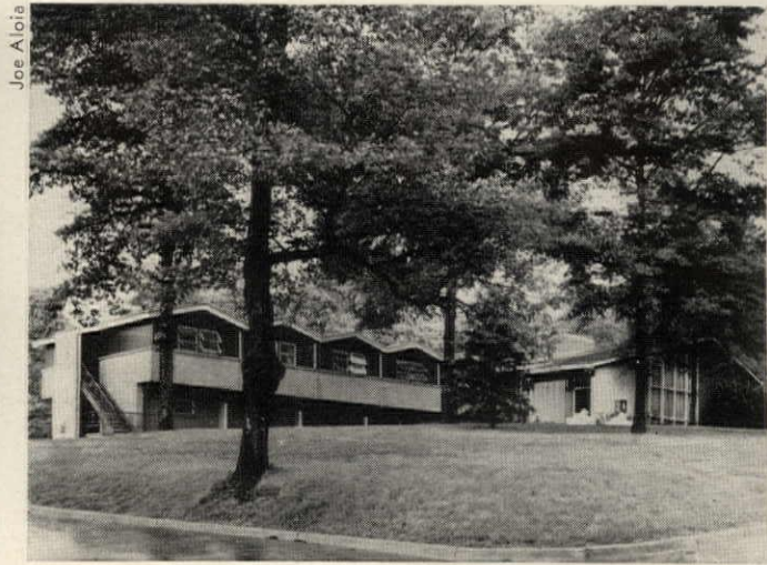
FRATERNITY HOUSE was built for 34 Birmingham Southern College students for $55,000 by Homebuilder Crowder. Architect: Philip Kessler.
