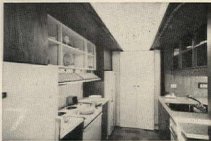
KITCHEN is fully equipped. Appliances "plug in" to rough wiring and plumbing in floor.
