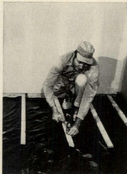
STEP 2. Vapor barrier of .004" polyethylene film is laid over strips and a second set of 1 x 2s is nailed over the first set.
