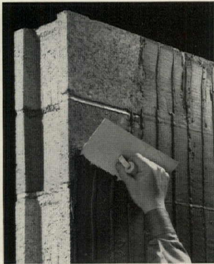
2. Apply Styrotac™ bonding cement.
