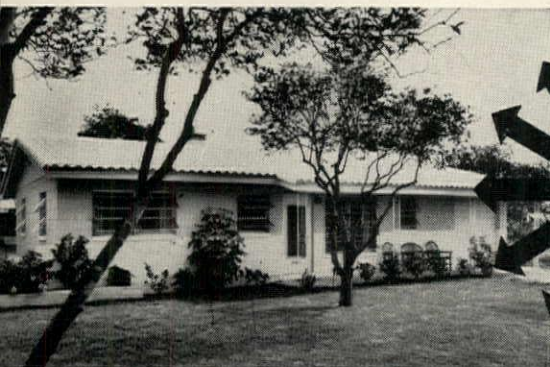
TYPICAL CHEEZEM HOUSE is concrete block with cement-tile roof. This two bedroom model—Cheezem’s second-best seller—has 1,008 sq ft plus garage, sells for $11,900.
