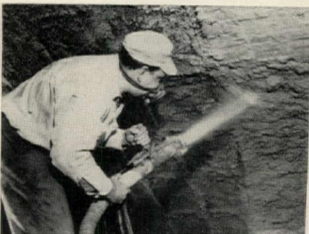
ASBESTOS INSULATION is sprayed 1" thick on 2½" concrete shell. Troweling smooths finish.
