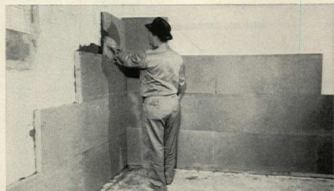
INSULATING BLOCKS of rigid urethane have low thermal conductivity, do not absorb water, and are easily cut with hand tools.
