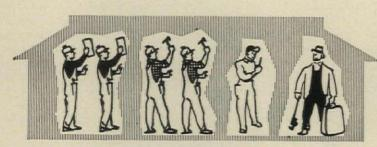
**10th day:** Two dry-wall men, two carpenters, heating contractor and plumber work inside without confusion. Dry-wall crew sands joints, Carpenters hang prefinished kitchen cabinets and install heat vents. Heating contractor installs furnace. Plumber installs fixtures.
