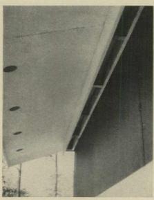
PREBUILT SOFFIT (Upson) is screened and primed. Also prebuilt: brick veneer mold.
