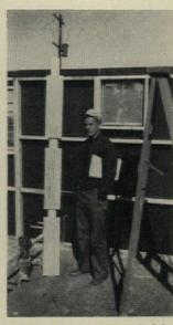
**PREBUILT T-POST** speeds joining of partitions to wall panels.
