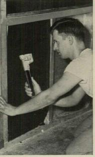
DUO-FAST Gun Tackers and Hammer Tackers make fast work of installing ceiling tile, insulation, building papers, plastic enclosures, metal lath and similar jobs.
