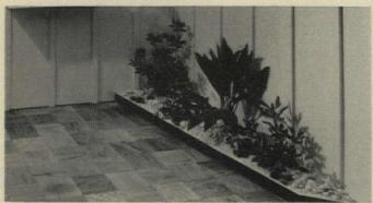
BOARD & BATTEN SIDING, shown in a display, is made by nailing or glueing Hypalon covered battens to plywood siding-sheathing sheets.
