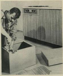
Wood-front steel cabinets combine durability of metal with appeal of wood. Steel door frames have channeled edges which will accept maker's line of paneled wood fronts—or any sheet material. Panels can be changed if owner wants to restyle kitchen.
