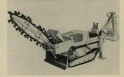
Trencher-dozer-backhoe is designed to handle practically any digging, grading, or filling assignment. It cuts trenches as deep as 78" and from 3" to 18" wide, at speeds up to 840'/hr. Backhoe has buckets from 12" to 36" wide and digs as deep as 8'4". And dozer blade can finish the job by backfilling and leveling ground to final grade. T-76 measures only 37" wide (without attachments).
