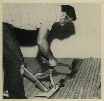
**Portable nailer** cuts nailing time for hardwood flooring as much as 65%. And a conversion kit (photo right) adapts the tool for face nailing. Porta-Nailer has a non-marking fiber base for nailing pre-fininshed flooring without scratching, and
