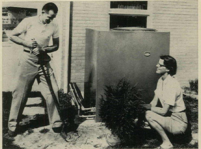
GAS COOLING UNIT made by Bryant uses absorption principle. Vertical exhaust lets owner landscape around it.
