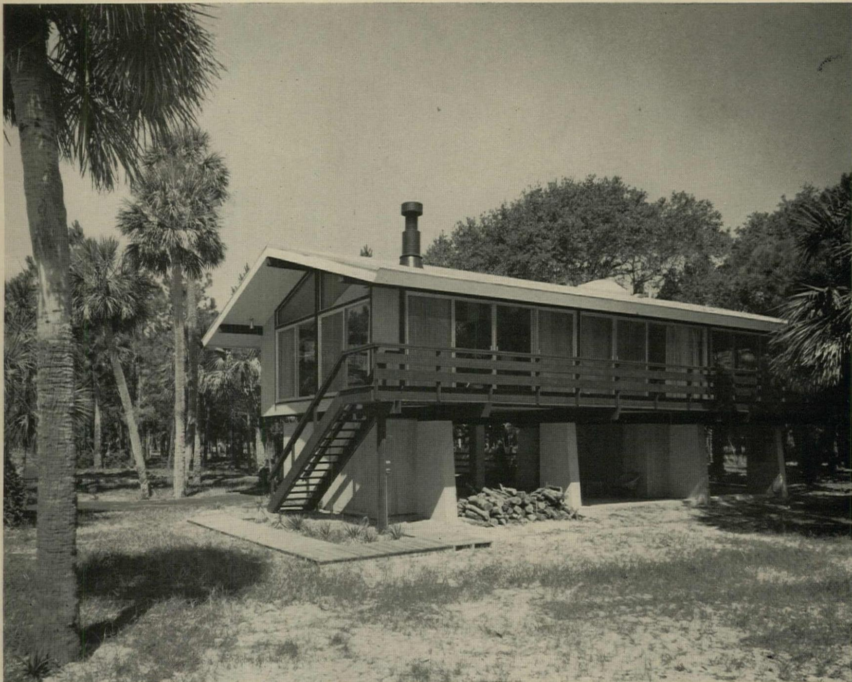
RAISED HOUSE has walls made of sliding glass doors to open house to view and to breeze. Long balcony serves as corridor in this simple plan.
