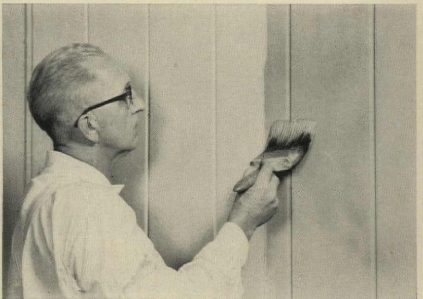
SAVES $65 PER HOME. Medema estimates "savings of $65 per house because factory-primed Insulite Siding saves us one complete coat of paint. What's more, we find it helps make the finish coat blister-free. We have never had a paint complaint on Insulite."
