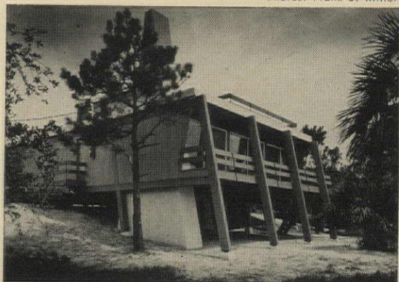
SLANT-FRONT HOUSE shows freedom of design typical of Sea Pines. Slanted posts are main vertical supports.
