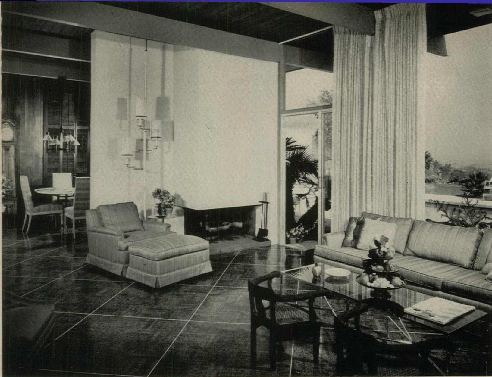
FIREPLACE WALL (a) separates living and dining rooms. Transom over glass doors extends to ceiling (2" solid t&g sheathing on 4x12 beams).
