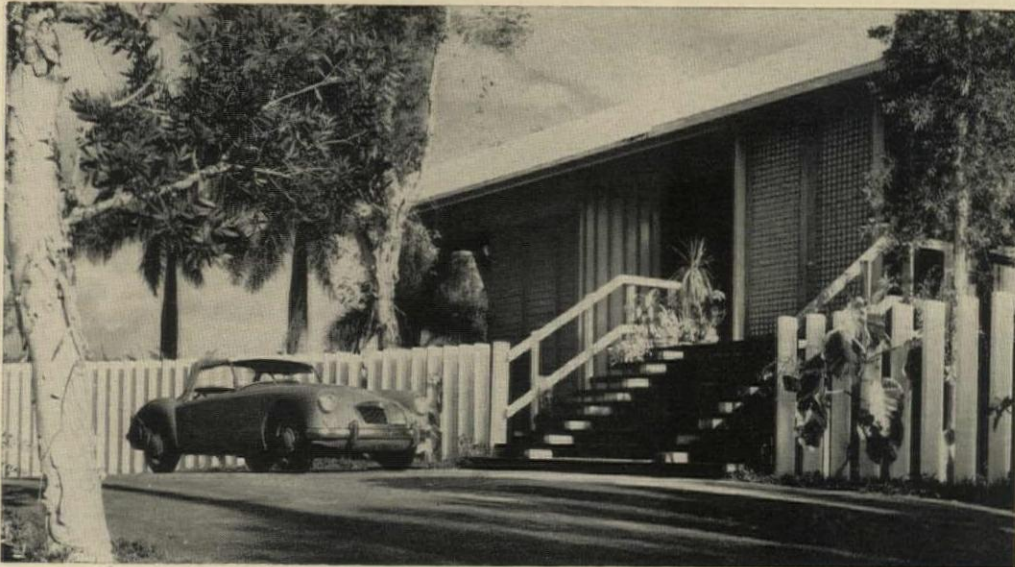
14. These precast concrete posts form a new kind of fence
