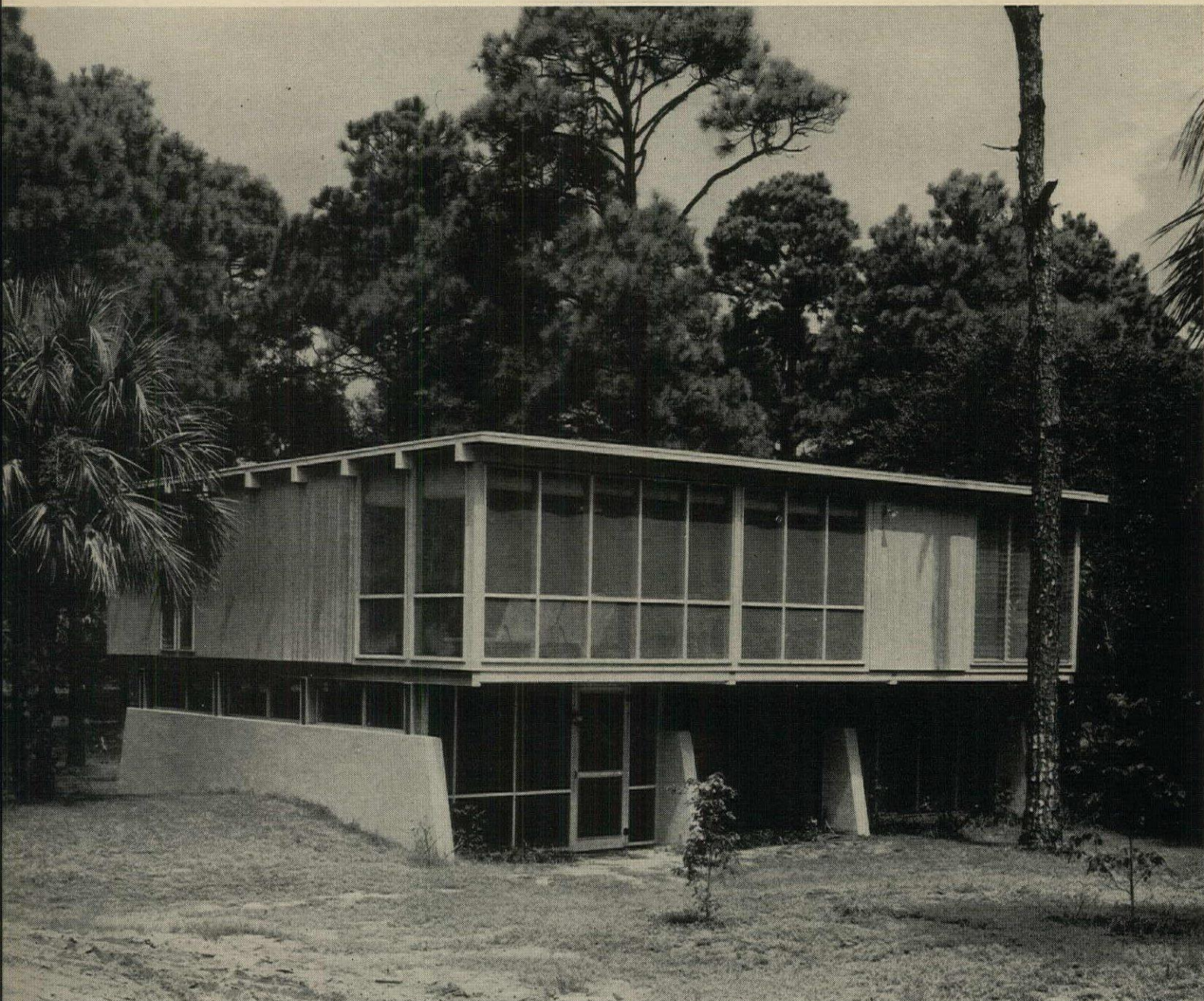
OCEAN SIDE of house has large screened porch for most of its length. Lower level is also screened, has bath for "desanding" bathers.
