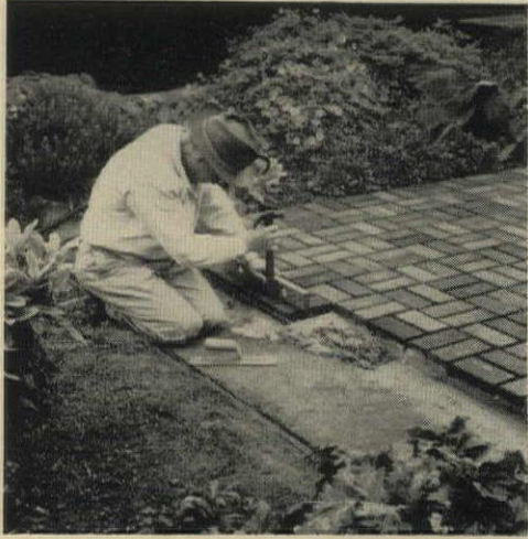
37. Brick is traditional outdoor flooring
