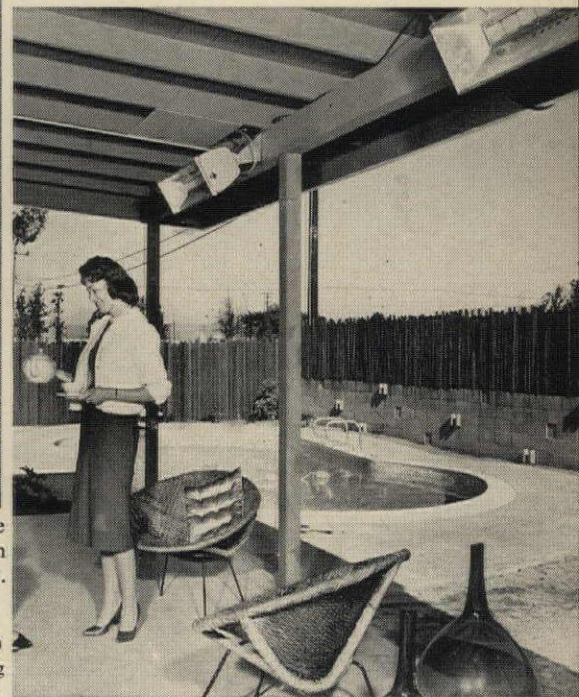
SWIMMING POOL HEATERS supply a growing market for gas. Burkay model has self-generating controls, needs no external wiring.
