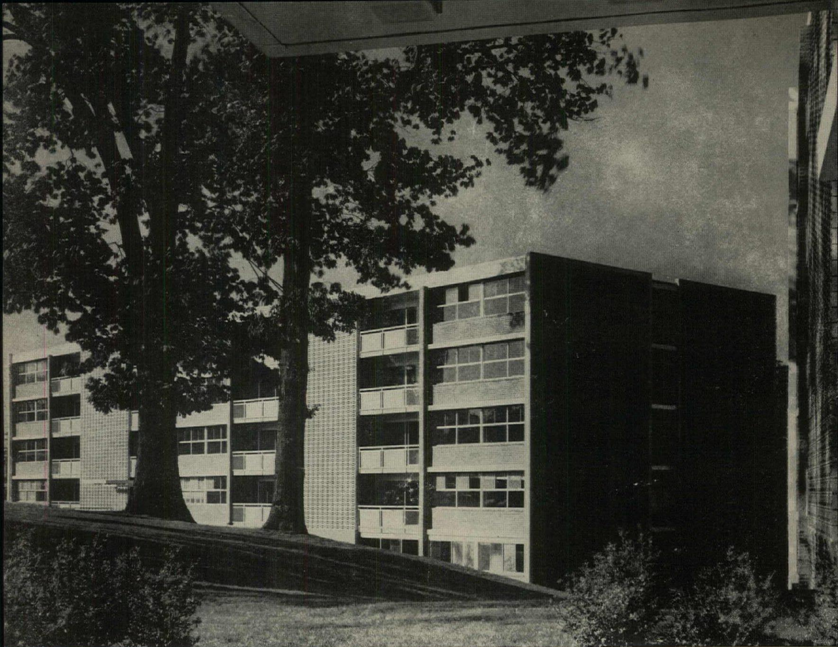
UPHILL, ENTRY SIDE of each building is four stories tall. Big trees were saved throughout the park-like site.
