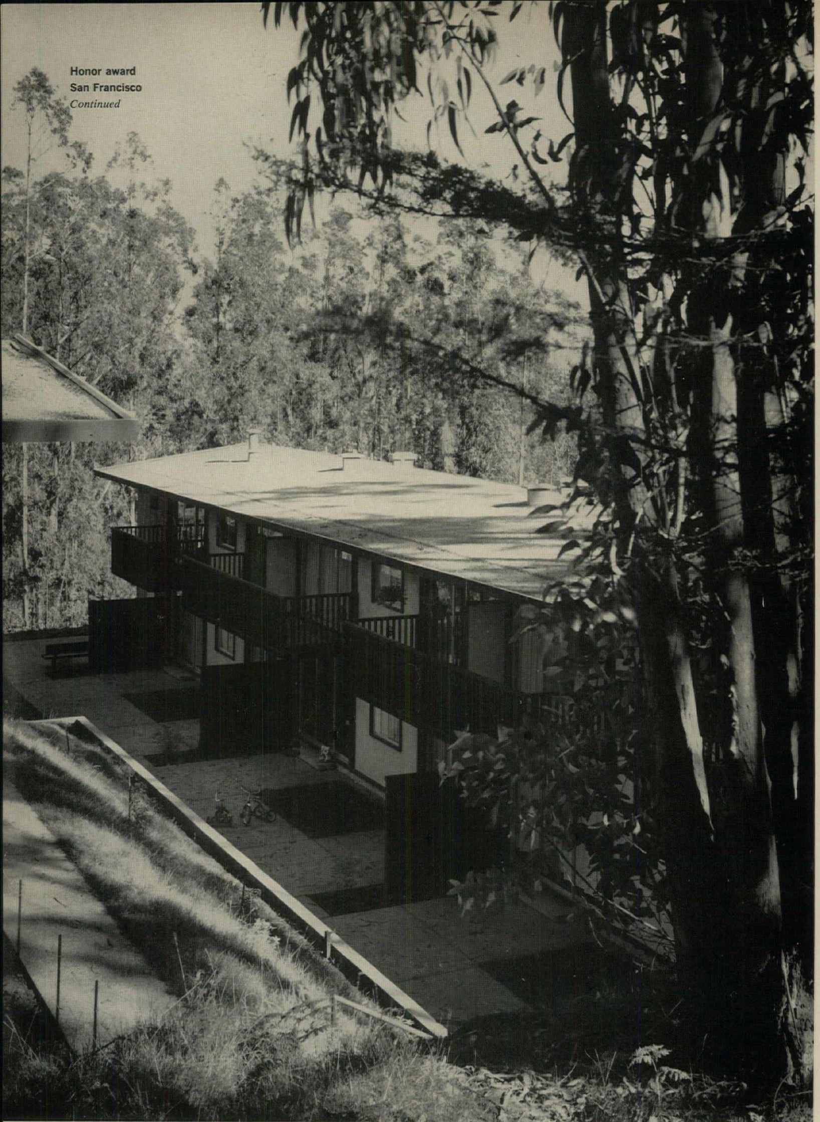
OUTDOOR LIVING SPACE , on terrace or balcony, opens directly to rear living rooms in each apartment through wide sliding glass door.
