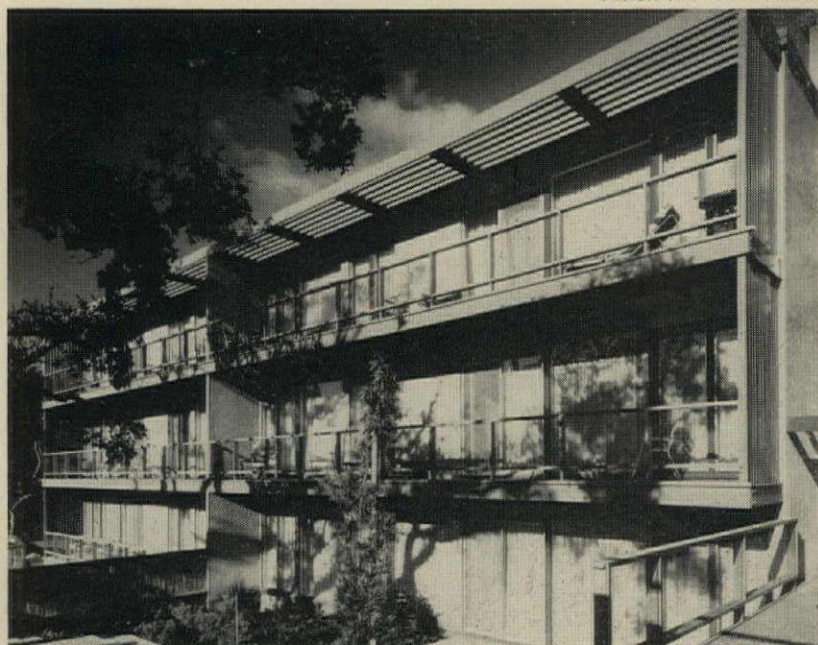
APARTMENT-LENGTH BALCONIES OR PATIOS —up to 40' long and with dividers between apartments—give each tenant a private outdoor living area.
