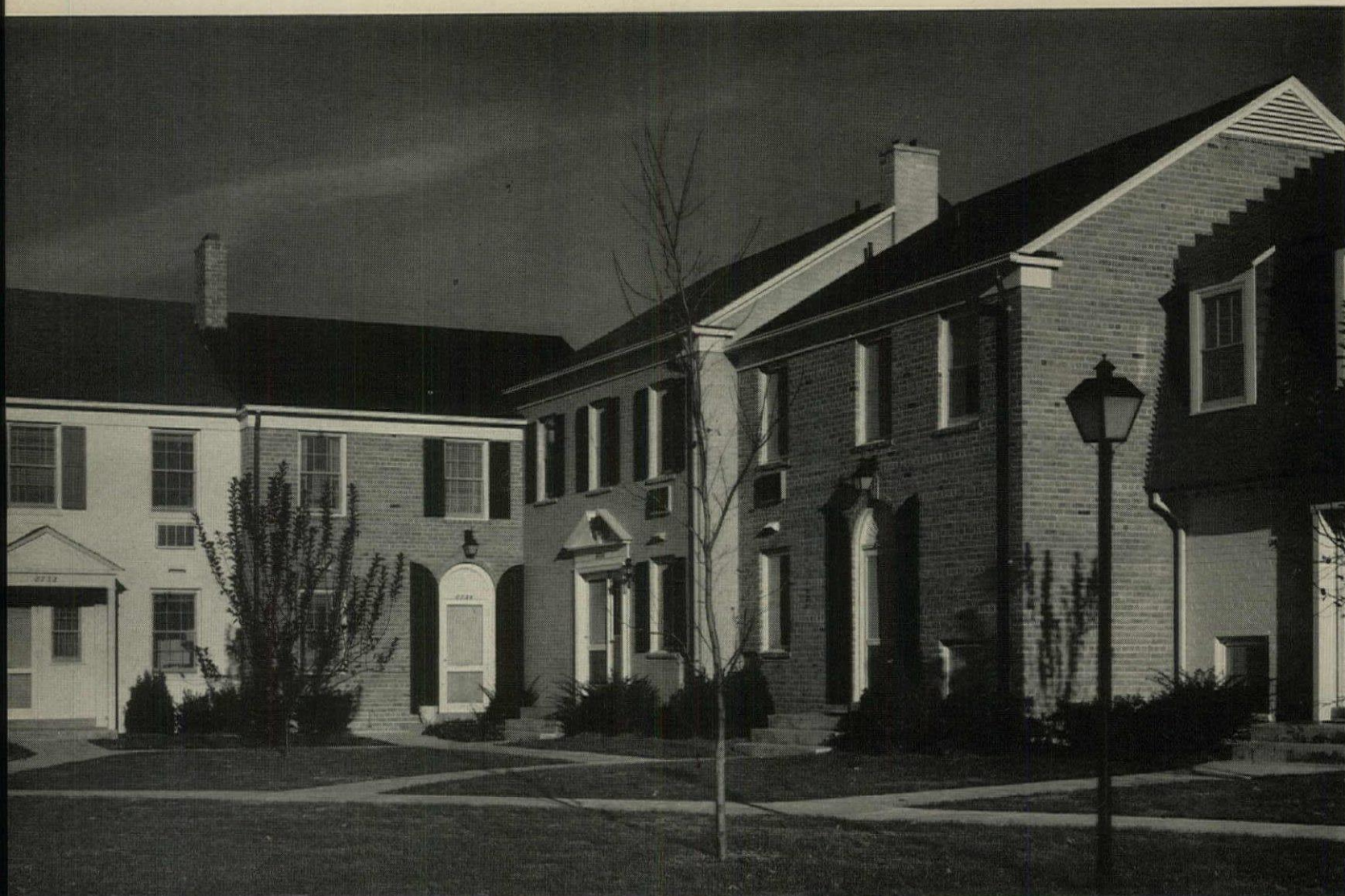
INDIVIDUAL FACADES of similar townhouses have different textures and colors of brick and different window and entrance treatments.
