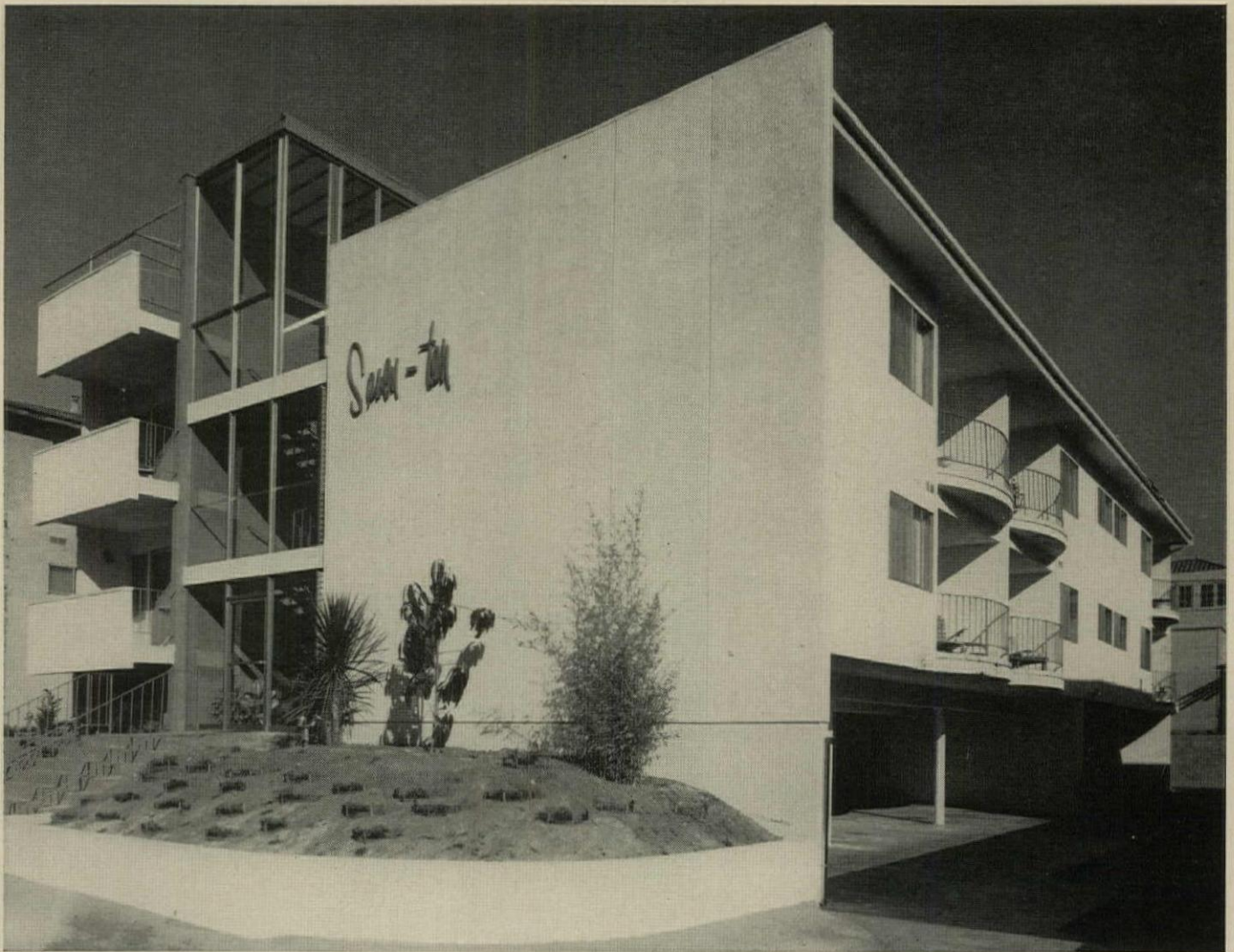
BLANK FRONT WALL gets design interest from three-story-high glass-walled stairwell. Balconies, right, open apartments to view.
