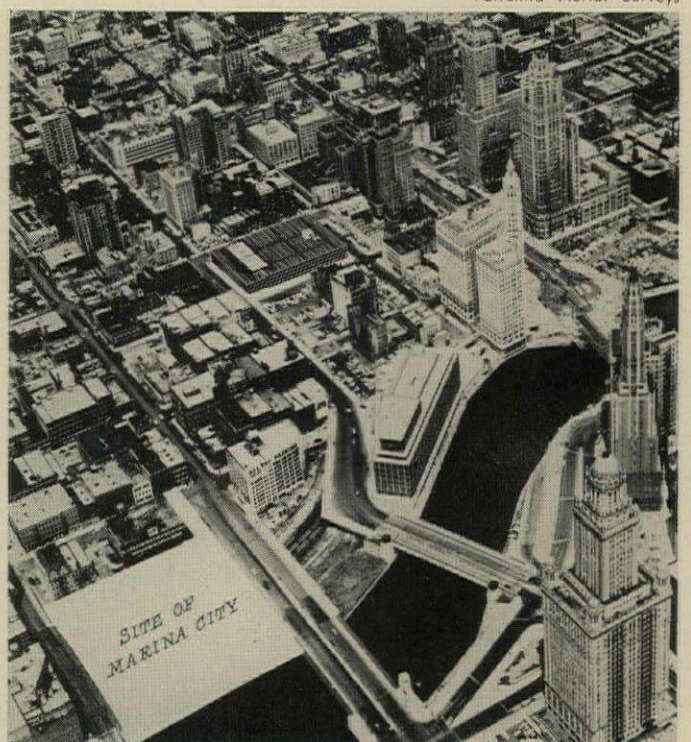
SITE OF MARINA CITY , on Chicago River near Lake Michigan and on edge of main business district, is Block 1 on original plat of Chicago.
