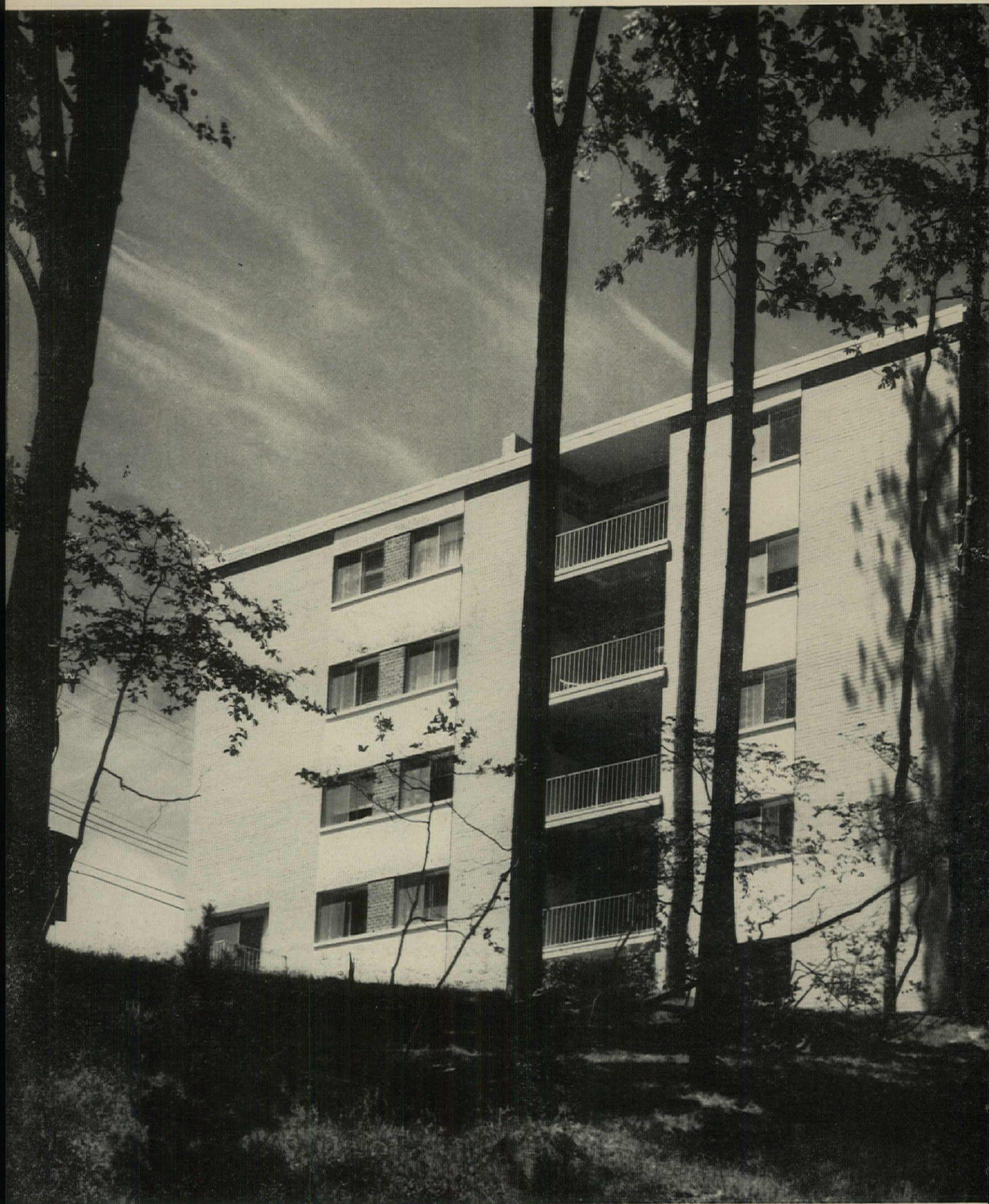
FIVE-STORY APARTMENT in Silver Spring, Md. offers high density with maximum open space. Architects: Collins & Kronstadt.
