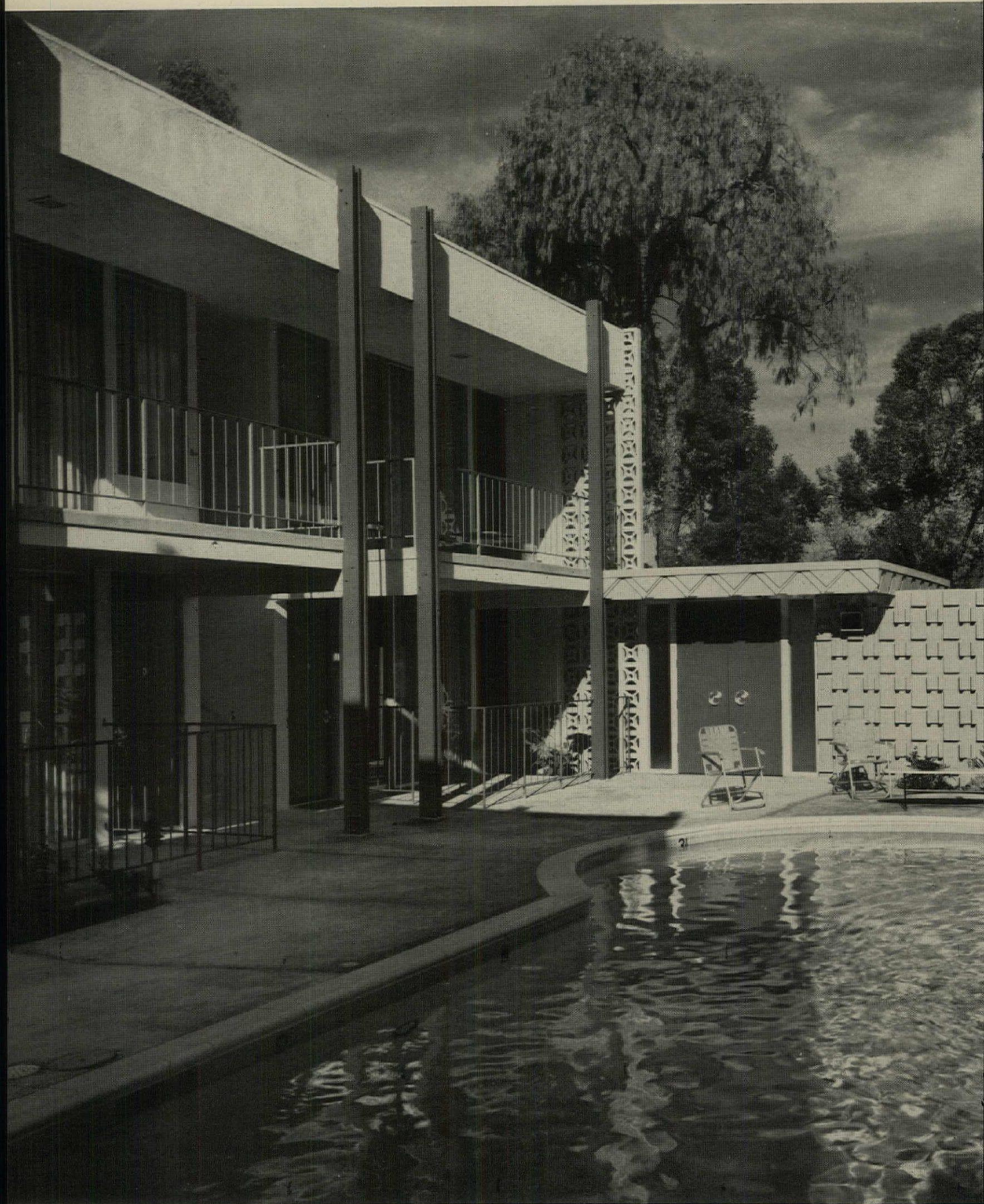
NINE-UNIT APARTMENT WITH POOL was built by Flair Corp in Woodland Hills, Calif. Architect: John B. Ferguson & Assoc. For details, see p 166 .
