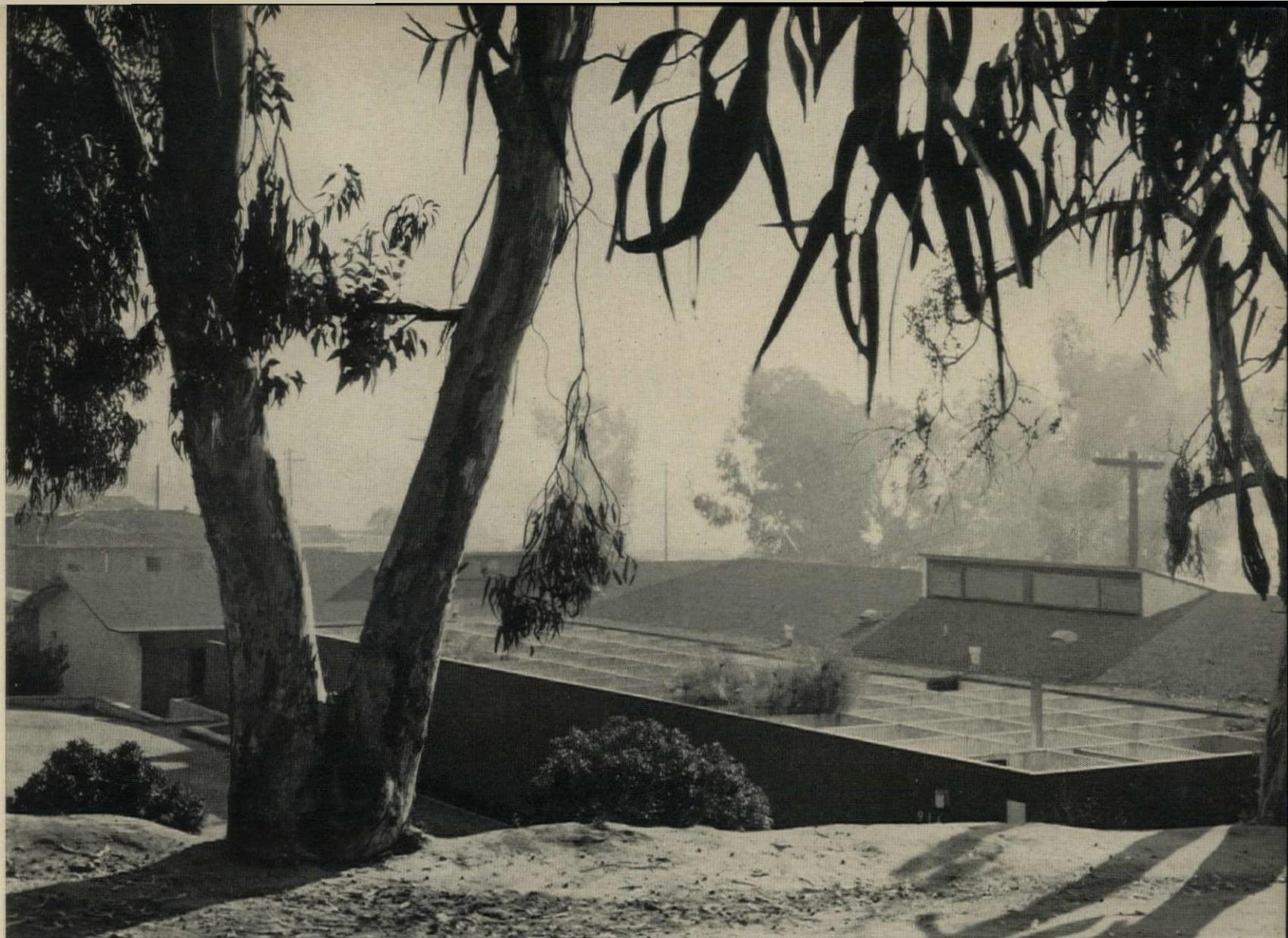
BELOW-THE-STREET DUPLEXES , their outdoor living areas screened by fences and overhead grilles, offer complete privacy for tenants.
