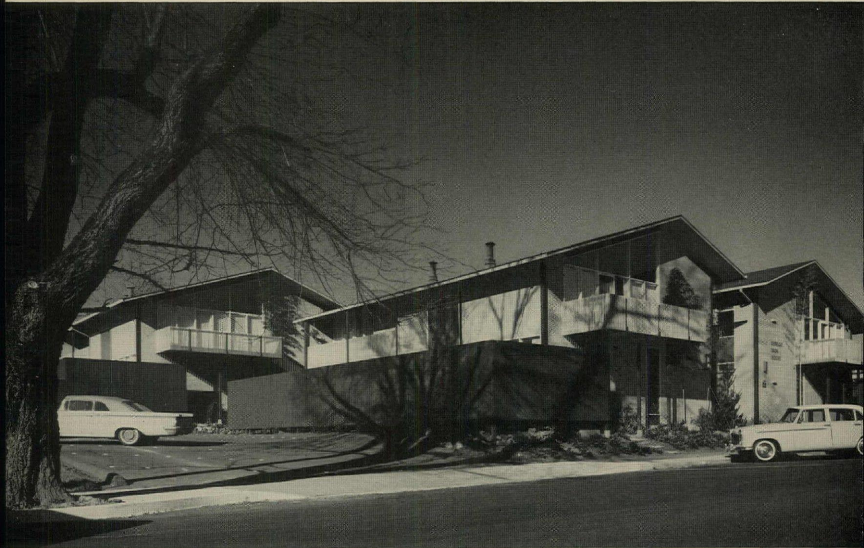
TIGHTLY GROUPED FOUR-UNIT BUILDINGS provide outdoor living in fenced terraces or balconies for 22 families on ½-acre site.
