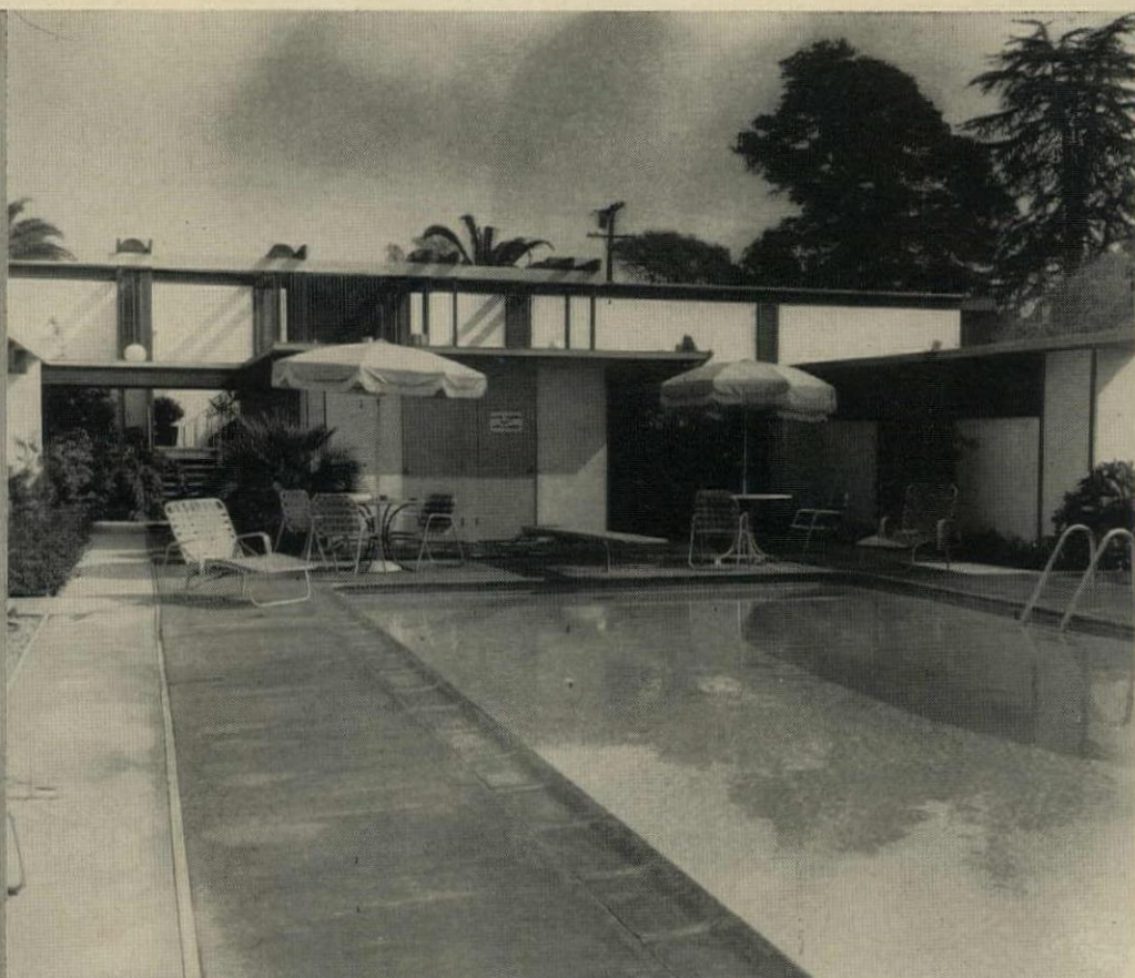
CENTRAL POOL AND TERRACE is only a step from all 20 apartments. Rooms facing this court have high windows for privacy.
