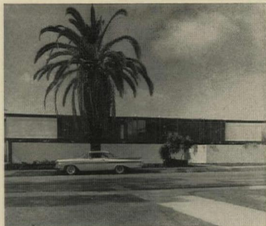
CONTEMPORARY FACADE is closed to street. Wood-frame building has stucco walls with redwood trim.
