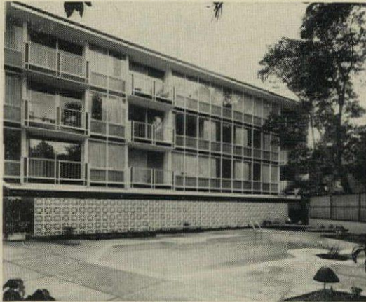
PIERCED BLOCK SCREEN shields cars parked under the building from view from the outdoor recreation area.
