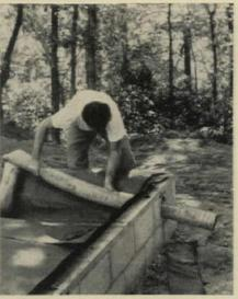
**2.** Forms are laid on vapor barrier, inflated to 14 psi. To turn corners, forms can be bent to a radius five times their diameter.
