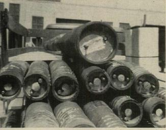
**ALUMINUM ENDS** of inflatable forms have tire-type valves. Forms can be used in any weather and stored in the open.
