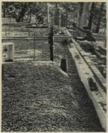
**1.** Gravel base is formed, right, to bring bottom of duct to exterior grade, rather than 2" above it (this is new FHA-MPS ruling).
