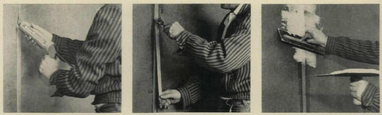
EPOXY FILLER is applied with caulking gun. KRAFT PAPER is pressed in with knife.
