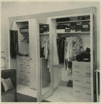
**OVER CLOSET DOORS.** fluorescent wall bracket serves to light the interior and to give general room illumination. Part of light is deflected upwards to the ceiling.
