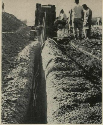
**TRENCHING** can usually be done cheaper by builder than utility builders' costs run as low as  $10\phi$  a foot if job is lumped in with other earthmoving work. Job shown is Centex Construction at Elk Grove, Ill.
