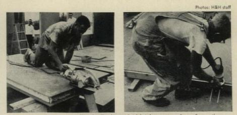
PANELS CAN BE SITE-CUT. Wood spline in panel (right) is temporary brace for routing.
