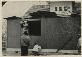
**ROOF IS SHEATHED** and picture-window frames set in place. Total time for the whole job, including trim and roofing: 71/2 hours. /END
