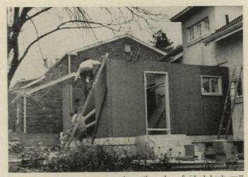
**KING-POST TRUSSES** are passed up through unfinished back wall. Two men, unfamiliar with panels, built the whole 16'x21' addition.
