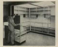
PANELS slip into grooves formed in frames.
