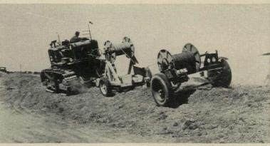
**CABLE-LAYING TRAILERS** are towed behind plow (left) which is pulled through earth by tractor. Cable is fed through the shoe of the plow to the correct depth, which is established by plow adjustments.
