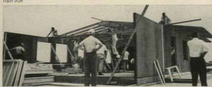
**ROOF TRUSSES** are put up on panel walls. End panels were left out until all trusses were up. Despite newness of the system, building crew closed in the house in one day.
