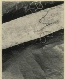
**3.** Loose wire coil is placed around inflated form. Coils at 5' intervals raise form 2" so concrete will flow under it.
