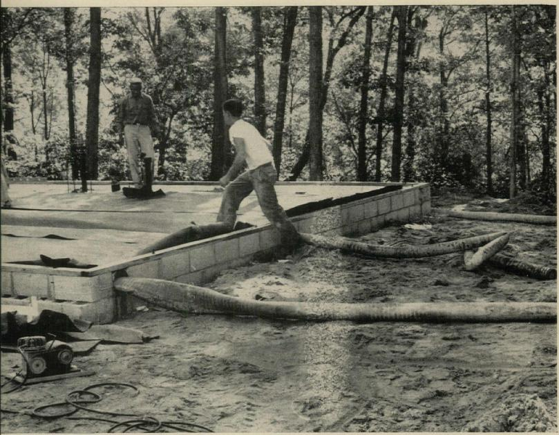
RUBBER TUBES form ducts in slab. They are inflated before slab is poured, deflated and withdrawn after concrete sets.
