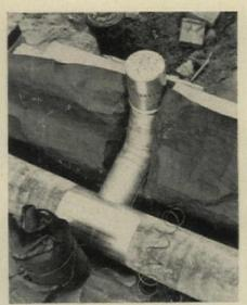
**5.** Wall register is strapped on like floor register. When form is deflated, it is easily drawn out through galvanized sleeve.
