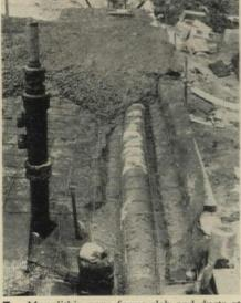
7. Monolithic pour forms slab and ducts at same time. Resulting jointless duct cannot be blocked with concrete or rubble.
