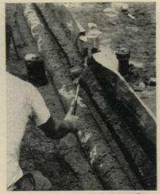
**8.** Flexible form, hit with hammer, vibrates concrete and insures smooth ducts. Most other duct systems need special vibrators.
