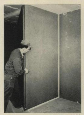
**UNFINISHED PANEL** is set against exterior wall. Skin has no nail dimples, so only joints need finishing.
