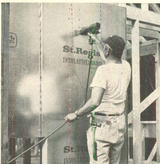
This product offers an option on method of applying either with nailing in the conventional manner or through the use of a stapling device.
