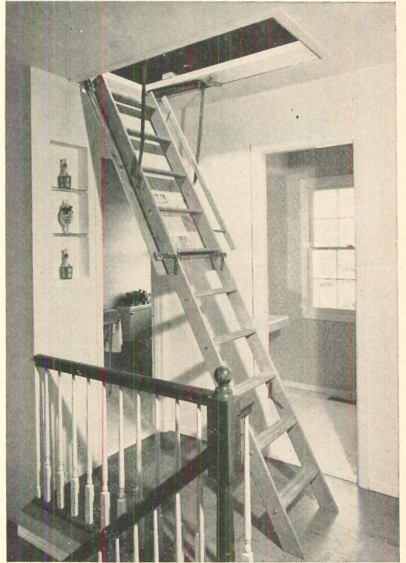
PULL-DOWN STAIRS lead to 500 sq ft attic in "Manor House"—useful for storage in basementless model.
