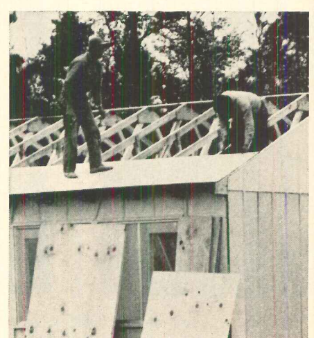
WALK ACROSS sheathed roof - From left gable end to right gable end 59.20 .30
