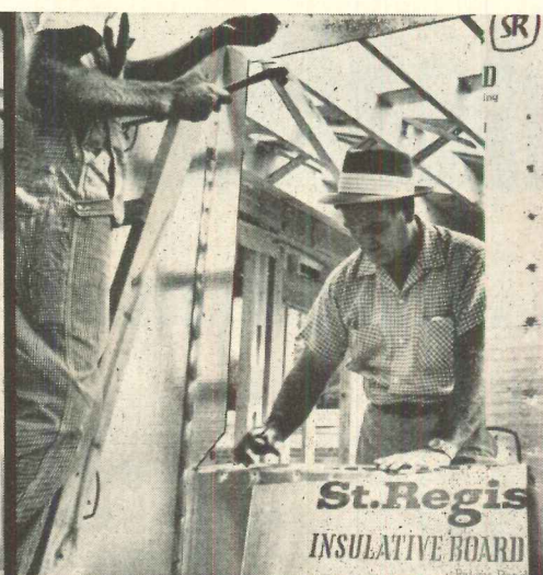
Door and window openings can be cut out after applying to studs. Cut can be made several inches from the framing, bending resulting flange back to provide additional flashing between framing and sash.
