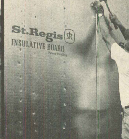
Marked for convenient positioning over studs. Specially tapered and reinforced edges permit lap. Means less nails, half the time to apply compared to other sheathing which must be pre-cut and butted.
