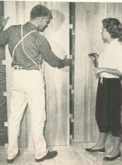
WALL PANELS in 32"x84" or 96" pieces have self-furring, self-aligning back strips.
