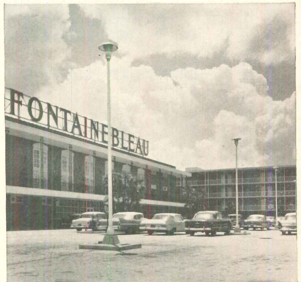
PTL's light the approach and grounds of the Fontainebleau Motel, New Orleans. The scientifically designed optical system directs the light down, rather than onto the windows of the building.
