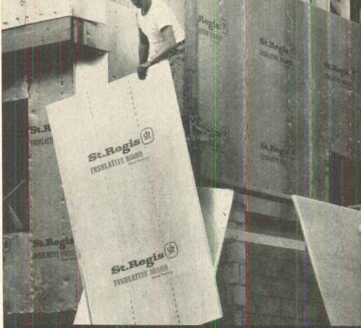
Light in weight — approx. 6½ lbs. per 4' x 8' sheet. Top this "one-handed" situation with heavier types of sheathing board. One man can easily carry a half dozen panels or more. Speeds work, reduces fatigue.
