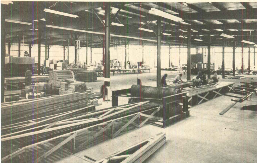
80,000-SQ-FT PLANT , not yet fully equipped, is now producing 75 houses a month with 80-man force. Output is expected to double in '61.
