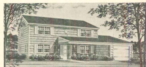
New two-story (plan at left) has 1,854 sq ft—100 sq ft more than previous version (plan at top). In new model, stairs and powder room were relocated to provide true center hall, family room was enlarged by extending part of kitchen into laundry area behind garage. Four-bedroom house has trim garrison front (second-story windows align with first-floor door and windows), sells for $17,500 with air conditioning and 8,400 sq ft lot. Three-bedroom version (right) has 1,772 sq ft and same first-floor plan, sells for $16,990.
