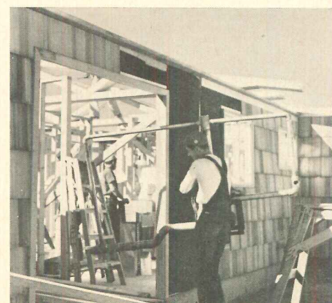
PLUMBING TREE is carried into house. Since photo was taken, tree is supplied built into panel.
