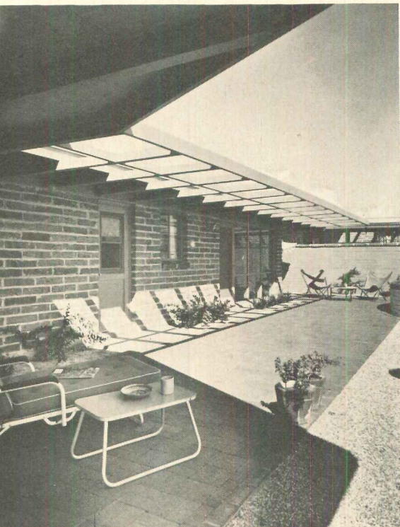
PATIO LIVING is featured in nearly all Lusk houses. Ramadas and wide overhangs shade rear windows and part of patio.
