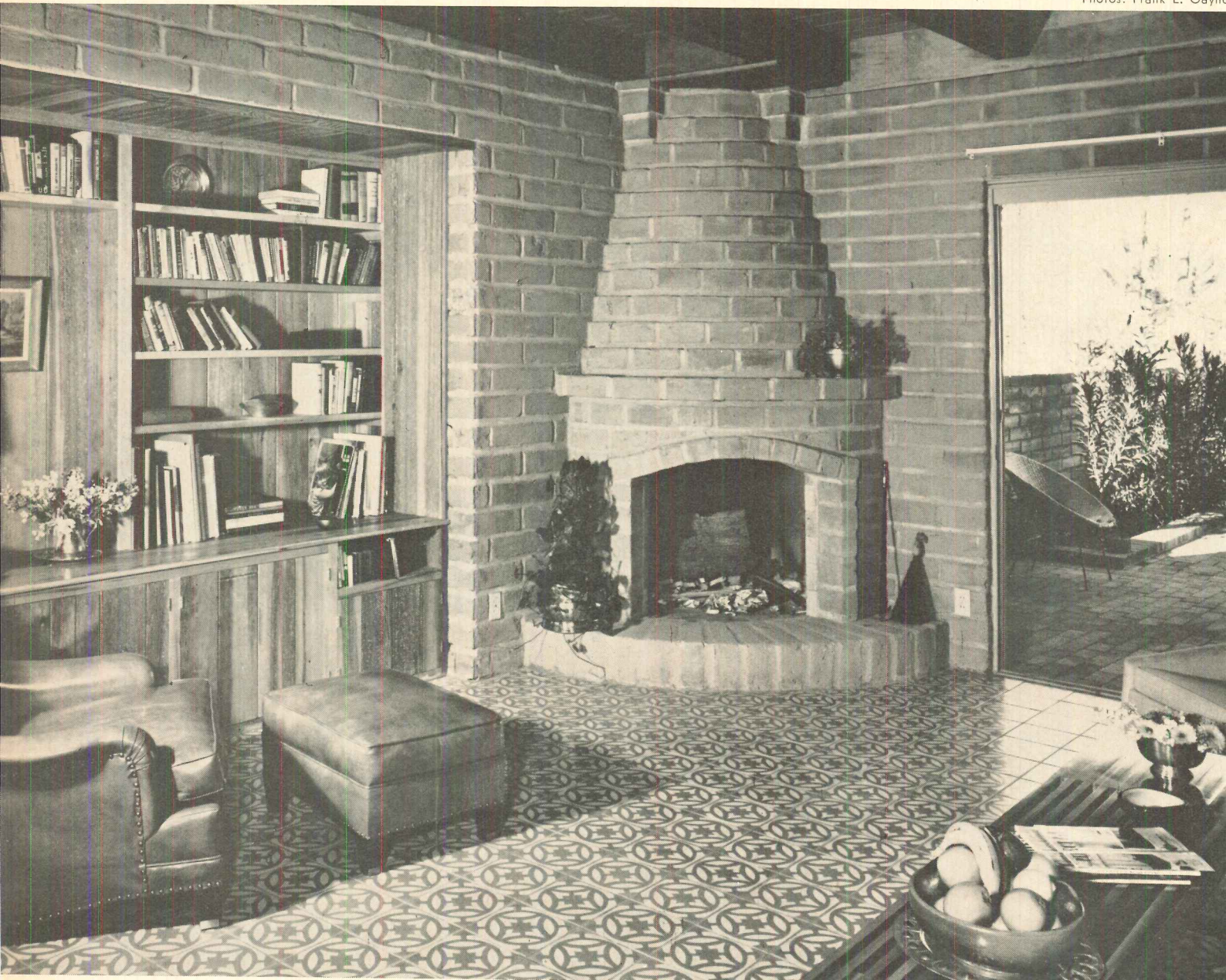
TERRITORIAL DESIGN is achieved with hand-made Mexican tile floor, adobe brick, and beehive-shaped fireplace in family room
