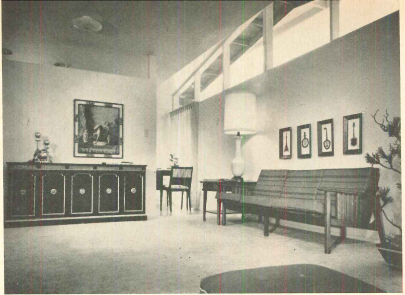
CLERESTORY across front living-room wall is obtained by leaving ceiling open to pitched roof for first 2' before first truss position.
