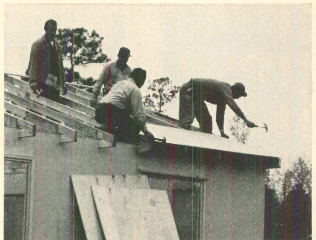
Hold (aligns + nails to trusses) 48.90 .40
