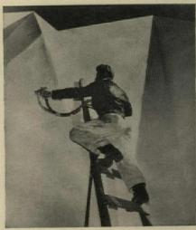
VINYL ROOFING is sprayed on in three coats that form membrane 40 mils thick.
