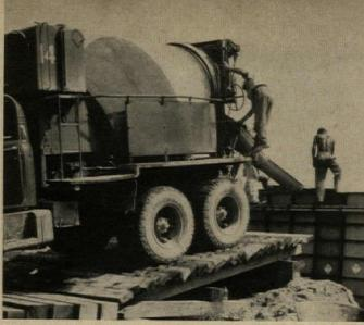
TRUCK BACKS UP TIMBER RAMP to pour into top of forms. A 40'x24' house takes 20 yd of concrete. All walls poured in two hours.
