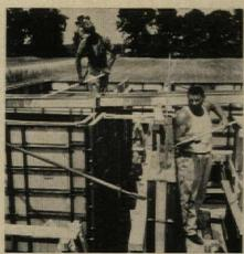
CONCRETE IS SCREEDED as soon as form is full. Note conduit at top of form.
