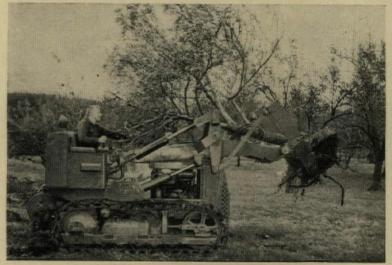
SMALL TREE DIGGER on tractor can move 4" tree in 30 seconds.
