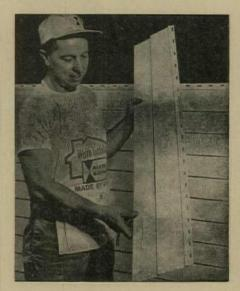
Narrow clapboards are now reproduced in Alcoa's aluminum siding. New material has two 4" boards in each 8" wide panel. Like Alcoa's 8" horizontal and 12" vertical siding, double four is made of Alumalure-coated alclad, in white, grey, green, yellow, charcoal grey, maroon.
