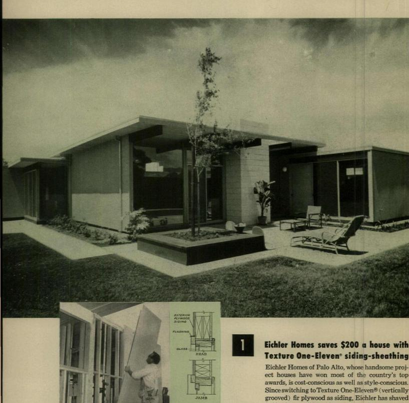
Typically, T 1-11 is nailed to studs 16" o.c. Edges are shiplapped. Standard millwork is available to fit. Insulation can be applied between studs if needed. For more information on fir plywood siding-sheathing, write Douglas Fir Plywood Association, Tacoma 2, Washington.
