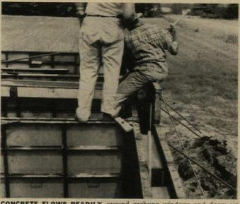
CONCRETE FLOWS READILY around prehung windows and doors set in forms (foreground). Diagonal rods are temporary form braces.
