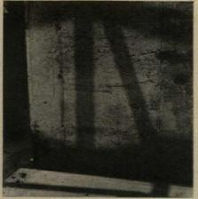
**CONCRETE SURFACE** has rough texture that provides a "tooth" for plastering.
