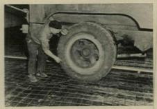
**BEFORE POUR**, vapor barrier and wire mesh will support weight of transit-mix truck.
