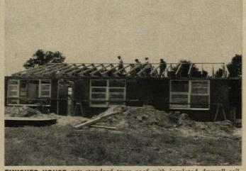
FINISHED HOUSE gets standard truss roof with insulated drywall ceiling. This house is the first of an 82-house development. Price: \$14,500.
