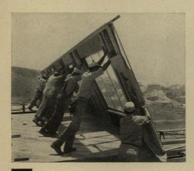
Tilt-up fir plywood walls mean savings of \$525 per house for Smith & Kline Construction Co., Castro Valley, Calif. They fabricate entire 40-ft. second-story walls, then tilt them up into place. This eliminates the time and cost of erecting scaffolding, and plywood's structural strength makes bracing and blocking unnecessary.
