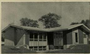
REAR ELEVATION shows how the hillside site was used to turn basement into a daylighted living, work, and play area.
