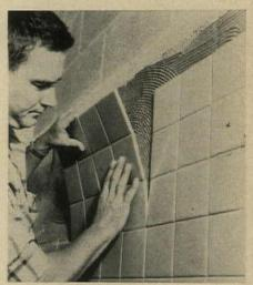
**Stylonet 12-set** is a 3x4-tile sheet of 4½" ceramic wall tile mounted on a paper-mesh backing that allows 70% contact between tile and wall. Sheets will not buckle, handle easily. Mesh is quickly cut with a trowel, is pliable enough to adapt to wall surface.
