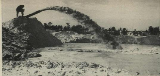
DREDGE TAILPIPE spews fill into dike-enclosed settling area. When fill is high enough, pipe is moved.
