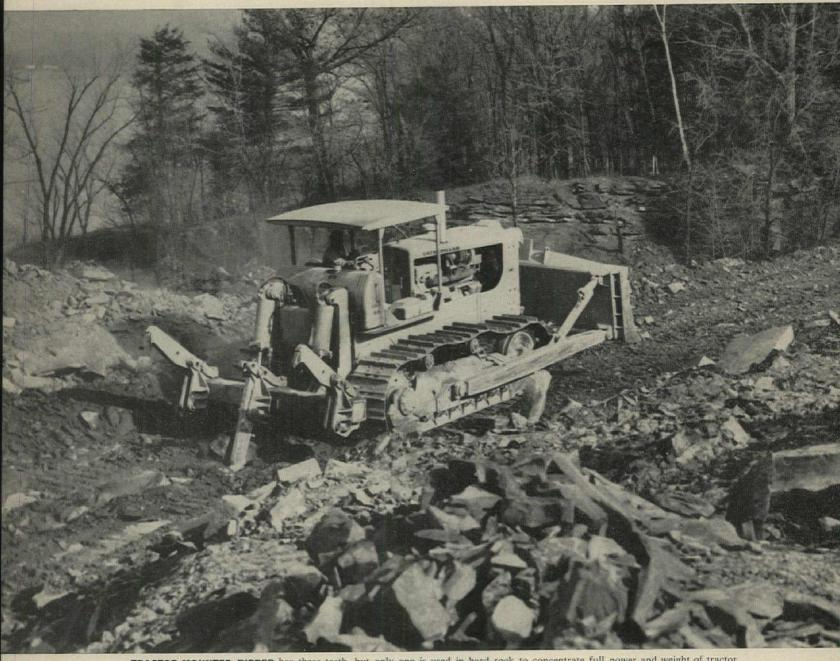
TRACTOR-MOUNTED RIPPER has three teeth, but only one is used in hard rock to concentrate full power and weight of tractor.
