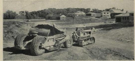
FOUR-WHEEL SCRAPER hauls topsoil to new lots. Scrapers strip and stockpile topsoil before building starts
