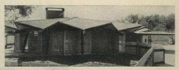
FINISHED HOUSE has nonloadbearing exterior walls that can be set at any position because buttresses (photo at left) carry all loads.
