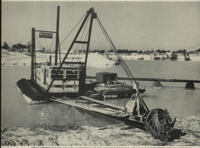
SMALL DREDGE dislodges and sucks up underwater soil with cutter head, foreground, and pumps it through tailpipe, right, to reclaimed site.
