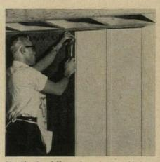
Vertical siding has been added to Alcoa's new line, is designed to match the 8" clapboard introduced earlier. Vertical corrugations 12" oc give board & batten effect. Siding is made of Alclad sheet Alumalure coated in dark and light green, maroon, white, and grey.
