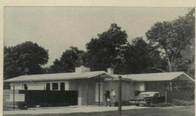
**COMPONENT-BUILT HOUSE** has vertical aluminum siding, interlocking aluminum shingles. Front roof is 42' wide; 57' rear roof extends to cover carport.
