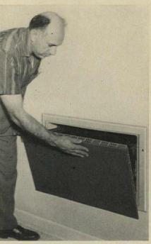
**3.** Next, attach the interior baffle. It's adaptable to any room decor. Paint, paper or panel it. Or hang a picture over it. All that's left is to plug in the Built-In *Thinline* and let it run.
