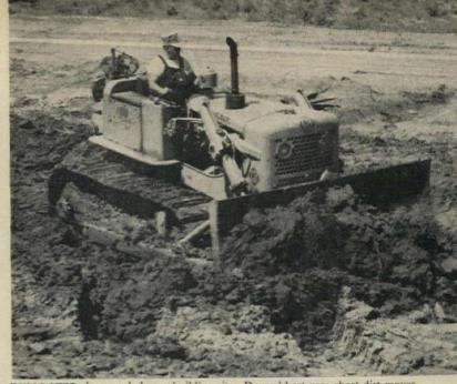
BULLDOZER clears and shapes building site. Dozers' best use: short dirt moves
