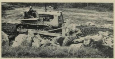
DOZER clears ripped rock. Ripper dislodged boulders or broke them in big chunks.
