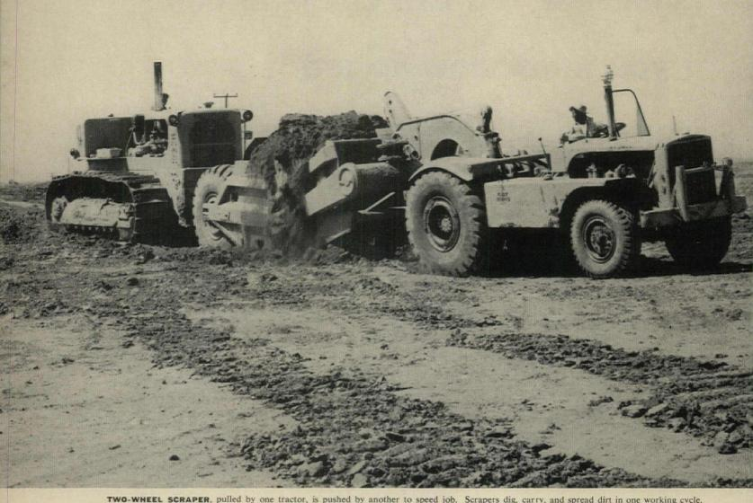
TWO-WHEEL SCRAPER, pulled by one tractor, is pushed by another to speed job. Scrapers dig, carry, and spread dirt in one working cycle.
