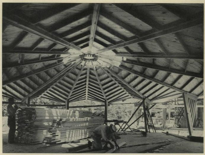
CIRCULAR ROOF is made up of 12 triangular folded plates fastened to ring which frames skylight. Twelve buttresses (photo, bottom left), set 12 joists (3x6s). Plates and joists converge at center steel compression
