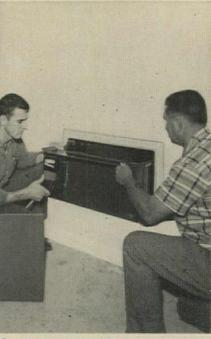
**2.** After the all-aluminum case is permanently sealed into wall with mortar, the drawer-type chassis slides easily into place. No nuts, bolts or screws needed. Outside louver installs from room side.
