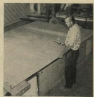
vapor barrier in sidewalls in a quarter hour. This was a onehour chore with hammer and nails. At an average of 10 panels per house, builder puts an additional \$16.88 in the profit column on each house.
