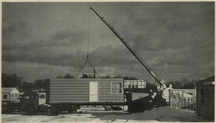
TELESCOPING BOOM, 85' long, is mounted on 42' trailer loaded with all materials for a house. Wall panels form trailer sides.
