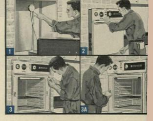
Install any model in minutes! Drop-Leaf Door or Frer Door models, all are designed for fast installation in sta ard 24" width cabinets or wall sections. With carpentry a rough wiring completed, simply: (1) Connect junction I and BX cable supplied. (2) Slide in unit (leveling screincluded, if needed). (3) Mount with concealed screws. (3 French Door models, tighten only two clamps (no screw
