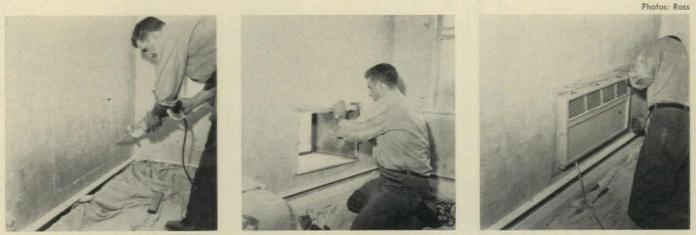
Add air conditioning. One easy way to do this is with room air conditioners. The photos above show three steps in the simple process. Left: the interior drywall is cut out and a matching cut (not shown) is made on the exterior. Center: the new opening is framed with a steel casing. Right: the air conditioner is set in place and the surrounding joint sealed with a molding, inside and out. If the house has warm-air heat, cooling may be added at the furnace.
