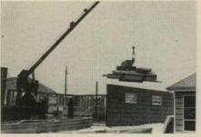
**U-SHAPED LIFT** designed by Schleicher hoists materials over erected wall panels.
