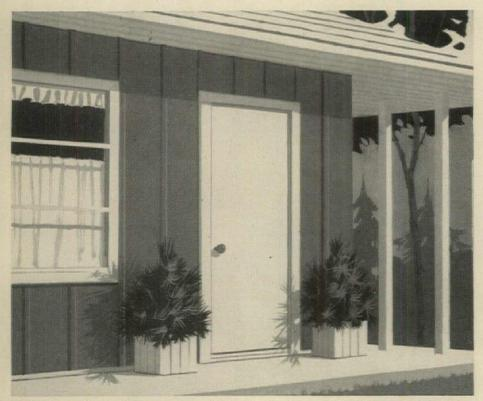
**Striking vertical effects** can be obtained with Duraply Flat Panels in traditional board and batten treatment. Or, you can eliminate battens for quick, easy applications by using the interesting grooved patterns of Weldwood Duraply Ivy League, Duratex<sup>®</sup>, or Duraply V-8 siding. All types of Duraply siding are available mill-primed.
