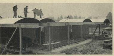
**Vaulted roofs** like the one on the Redi-Gas building in Parkland, Wash. are being adopted by more and more builders for home construction. Components were fourfoot-wide arched stressed skin panels of Exterior fir plywood with paper honeycomb core. Lightweight, easily handled, each spans 16 feet. Component construction helped keep total cost of the building to \$8.10 psf.
