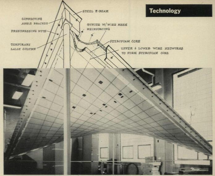
SADDLE-SHAPED ROOF PANEL is formed by wire network that, when tightened, forces foamed-plastic core boards into double curvature.
