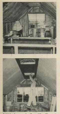
Add bedrooms in the attic. The attic shown here was turned into a bedroom and a den-sewing room, with plenty of storage between them. The attic was unfinished, but already insulated. The roof ridge was adopted as a lighting trough; plastic sheets cover the light bulbs and cut the glare. New wider window replaced the existing one. Battens to cover joints of painted plywood sheets give finished room a panelized look. Architect: Walter Widmeyer.
