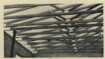
GANG-NAIL<sup>®</sup> GUSSETS MAKE HINES TRUSSES EXTRA RIGID Hines Trusses are built with patented Gang-Nail metal gussets and superior grades of kiln-dried Douglas Fir and Western Hemlock for the highest quality. Use Hines Trusses to speed building, save labor costs, reduce lumber waste, and eliminate interior bearing walls.
