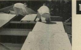
Roof panels, too, cut labor because they covered 32 sq. ft. at a time, providing ceiling, roof decking in one component. Man-hours required for roof: 15. Total cost of the house was \$13,000, or \$12.50 psf. Contractor was G. A. N. Company; architect, Charles Metcalf.
