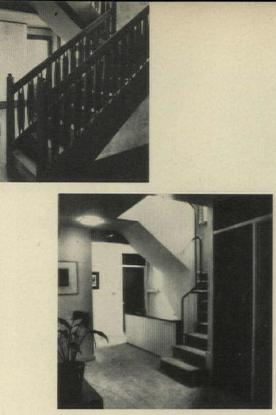
Add an entrance closet. The large staircase in this Massachusetts house was closed in so a goodsized hall closet could be built in next to it and near to the entrance. Closing in the stair made a new handrail a necessity so it was made as simple as possible, in keeping with the rest of the modernization. Architect: Frederick Bruck.
