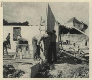
**EXTERIOR WALL COMPONENTS**, shown here during assembly include a blank wall panel, exterior door panel, two small window panels and two windowwall units. All window panels arrive on site ready glazed.
