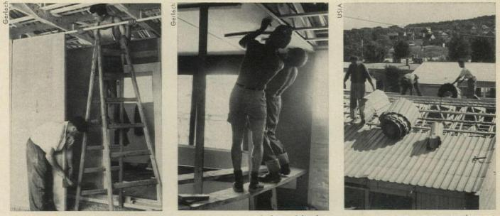
**PARTITION COMPONENTS**, in six varieties, fit into splines between floor slabs and roof trusses. Wiring is distributed through attic.
