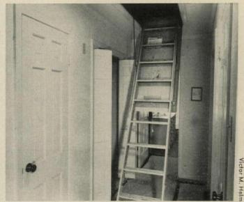
**PULL-DOWN STAIRWAY** gives access to 500 sq ft of dead storage area. Stair is pulled down into corridor flanked by four big closets. House was built by Mascari & Sumner for Houston Parade.
