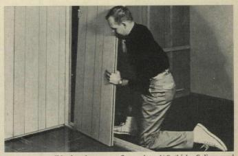
**PARTITIONS** slide in place over floor plate  $\frac{1}{2}$ " thick. Splines and plates tie panels into a wall more rigid than conventional partition.
