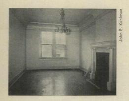
Add a large dining room. To turn this highceilinged second living room into a dining room, the mantel was stripped away. An opening was cut through the fireplace to make a passthrough to the kitchen. (The flue and its brick casing were left and covered.) Also added: dropped ceiling, new paneling over old walls. Modernizer: Walter Ford.
