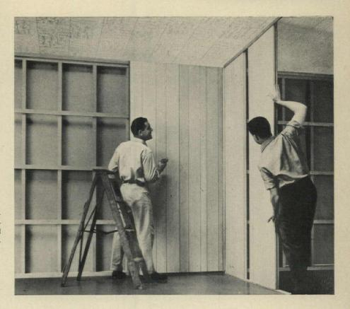
**FINISHED PANELS** are used to face structural walls or as integral, non-bearing partitions. Cherry graining gives the look of wood without the need for any job-site finishing.
