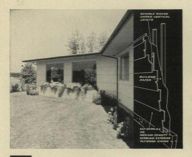
**Lapped plywood siding** makes a rigid wall without sheathing. On this Olympia, Wash. home, 16"-wide courses were nailed to studs, with wedges at joints. Plywood may be regular or, as used here by designer-builder Charles Sten, overlaid for a premium paint job. It may be ripped, or purchased precut (beveled or plain) in several widths.
