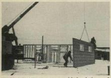
WALL-LENGTH PANELS, with insulation and siding, are lifted from trailer to slab.
