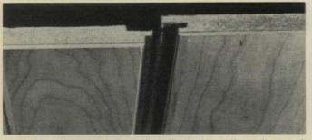
**EASY WALL PANELS** have an insulating-board tacking strip at each interlocking joint. V-grooves conceal joint where panels match.
