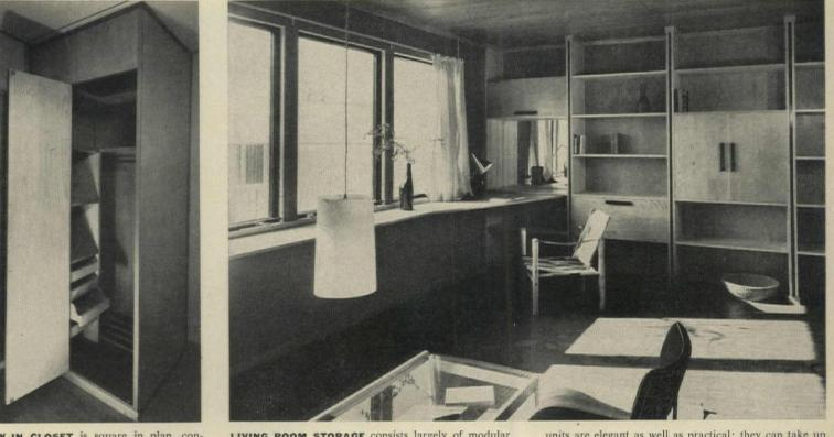
WALK-IN CLOSET is square in plan, contains sliding trays, shelves, hanging space. LIVING ROOM STORAGE consists largely of modular shelf units. Vertical reveals between prefabricated
