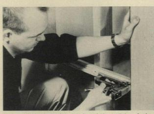
**PANEL UNITS** go up fast, can be quickly stapled to furring strips nailed to the studs. Fiberboard backing adds to wall's insulation.
