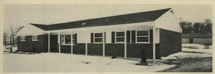
EXPERIMENTAL MODEL, build in 1959, has shallow bedroom windows, seven porch posts, half-height standard brick wall along the front.
