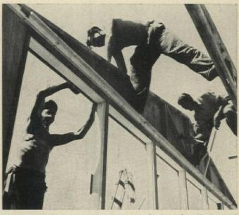
**ROOF TRUSSES** being erected here come in three sizes (7, 8, and 9 meter spans). In the pilot models, trusses were topped either with panels, or with "Fural" aluminum roofing on purlins (see below).
