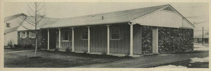
FOR-SALE MODEL has deeper bedroom windows, full-height board-and-batten front siding, used brick at end of house, six porch posts.
