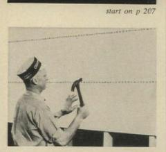
"Frame locators" eliminate guesswork in nailing Celotex's Celo-Rok or Fi-Rok gypsum wallboard. Each sheet is printed with small letters spaced 1" apart in lines 16" oc. When drywall is nailed vertically, the lines locate studs; horizontally, letters are the key. Lettering fades when exposed to natural light.
