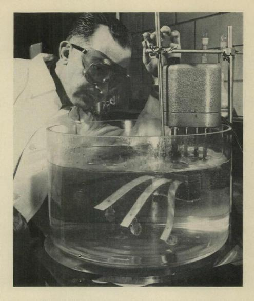
Tests like this show new vinyl can work for hot-water piping
