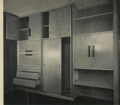
TYPICAL STORAGE WALL UNITS, all one-meter wide, were designed for use in many areas. Coat closet shown at center has sliding doors with recessed pulls.
