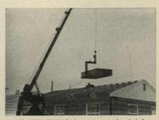
ROOF SHEATHING, last cargo unloaded from trailer, is swung onto trusses. /END
