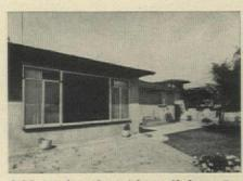
**Add enclosed outdoor living.** In this case, a plastic roof was added, to cover the outdoor living area. New roof line extended the length of the house to remove the old roof line's jagged look and shade the large windows. Brick planter also extends the length of the house to soften the appearance of the stucco finish. New outdoor living room has sliding glass doors and (not in photo), barbecue fireplace.
