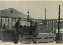
PALLETIZED LOAD of sheet materials is deposited exactly where needed inside walls.
