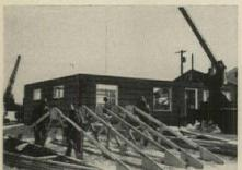
SIX TRUSSES ARE SPACED along angle-bar attachment notched at 2' intervals.
