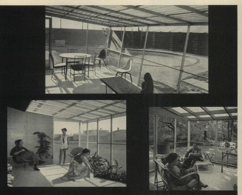
Fiberglas Translucent Paneling is resistant to weather and damage, comes in a new range of decorator colors, and is easy to handle because it saws and nails like wood. For all sizes, types and styles of homes, choose from prefabricated or custom-designed aluminum or wood-framed units. For versatile new patio plans by architect Herman York, write to Owens-Corning Fiberglas Corporation, Dept. 67-G, National Bank Building, Toledo 1, Ohio.
