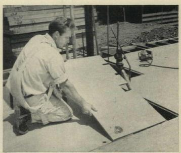
8 Fir plywood subfloors have cut floor installation costs in half for Andy Oddstad, big-volume builder in northern California. Using 5%-inch Ply-Scord®, one man can install the average floor in one day. It used to take two men the same time to do the job. Waste is negligible and DFPA-inspected PlyScord makes a solid base for finish flooring.
