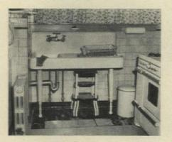
Add new equipment. This old kitchen was modernized by replacing the old equipment with new. The vintage 1925 sink was replaced by a built-in sink and cabinet, complete with garbage disposer. The new sink has a single-lever faucet. The new equipment also includes a built-in dishwasher, undercounter cabinets, and low storage between the counter and the window sill.
