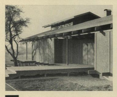
**Panel-and-batten** wall on Eugene, Ore. home was simply built with standard  $\frac{3}{8}$ " Exterior fir plywood nailed to studs with battens at joints, and stained. With weathering, plywood checks and acquires a pleasantly textured surface. One-step wall method meant low cost: \$8.75 psf. For the smoothest siding, use overlaid fir plywood, painted.
