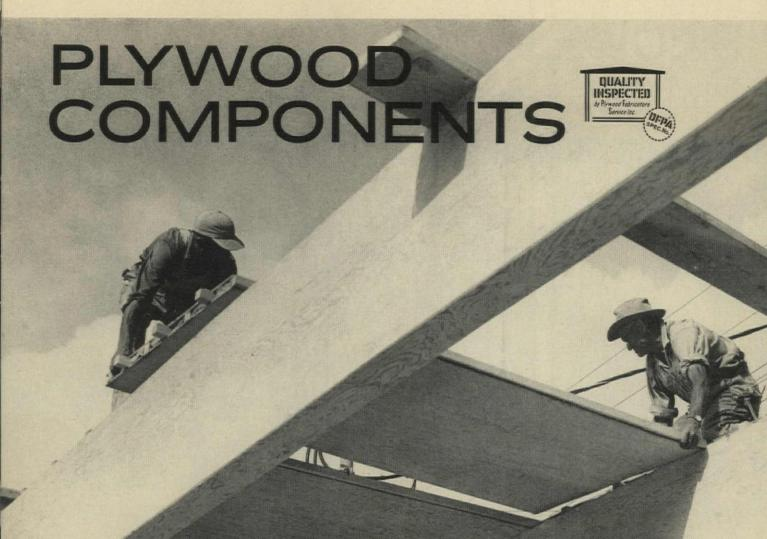
In building at Rochelle, Illinois, Hines Box Beams span 35'. Stressed Skin Panels form roof deck. Architect: Gene C. Jackson.
