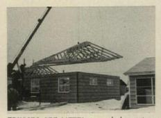
**TRUSSES ARE LIFTED** on angle bar, set on wall panels, and nailed in place.
