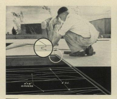
New tongue-and-groove  $2 \cdot 4 \cdot 1^{\circ}$  plywood cut labor 37% for Tacoma, Washington builder R. H. Wegner. The  $1\frac{1}{8}^{\circ}$  subflooring-underlayment is now available with t&g edges to eliminate blocking. Two men can lay 1,000 square feet in four hours, handling 60% fewer pieces than with conventional joist construction.
