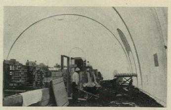
**\$1.25-a-foot space** is provided by Air: Seal airhouses. Vinylcoated nylon envelopes are sealed to ground by metal ballast rings or deep-soil spears. Hot-air blowers inflate and support tent. (Only 0.15" to 0.20" water-gauge pressure is needed normally, only 1" for gale winds.) Various colors are available. Price includes erection in Seattle area.
