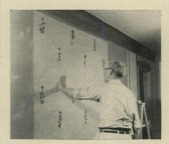
Vinyl wall covering is a sandwich of paper backing, aluminum foil moisture barrier, fabric and embedment decoration, Krene sheet overlay. Royaltex goes up like wallpaper, resists mars like vinyl, will not suffer from moisture staining. Sheets come 23"x95". Plain patterns cost 34¢ to 50¢ a sq ft, botanicals about 65¢. Over 20 patterns are available.
