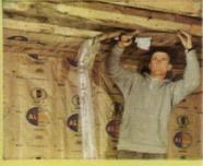
BUILDING OR REMODELING? Reflectal's Alfol Aluminum Foil Insulation is clean to work with, easy to install. Reflects summer heat out, makes homes 15° cooler—reflects winter heat in, cuts fuel bills as much as 35%.
