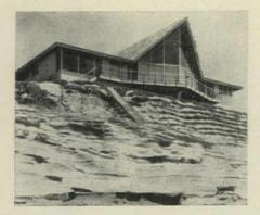
Steel columns and rafters, welded into big A-frames, make a structural cage for the two-story living room of this oceanfront house and support a glass wall that will resist wind and water pressures of 80 psf.
