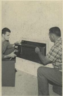
**2.** After the all-aluminum case is permanently sealed into wall with mortar, the drawer-type chassis slides easily into place. No nuts, bolts or screws needed. Outside louver installs from room side.
