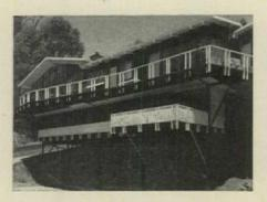
The rigid steel frame above springs from a unique foundation grid to provide solid support and wide spans for two living units—an upper-level house and a lower-level apartment.
