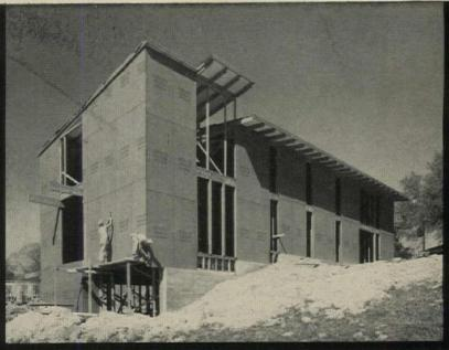
**Rugged Insulite Sheathing** was also used on Hillside Apartments. Easy to nail, easy to saw, the Insulite panels cut application time, saved waste.
