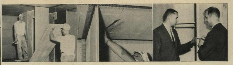
4 1" long length gypsum lath is then erected. Edges interlock for strength. **5** Safe-Edge Cornerite is stapled to the other side of lath at ceiling.
