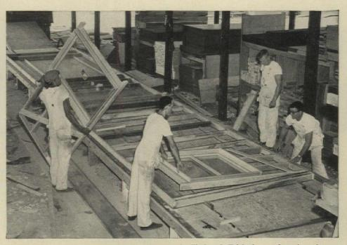
**Installation within minutes! Fits tighter!** At Fischer & Frichtel manufacturing plant, workers cut two load-bearing struts to fit header construction. Then nail Strutwall to adjacent studs to become an integral part of the wall panel. It's that easy!
