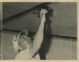
3 Safe-Edge<sup>®</sup> Cornerite is stapled to ceiling to hold top of lath panels.
