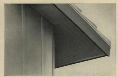
**Simple replacement** of plywood or cement asbestos facing material with aluminum panels results in cleaner appearance, easier application. Factory-finished aluminum eliminates painting expense.
