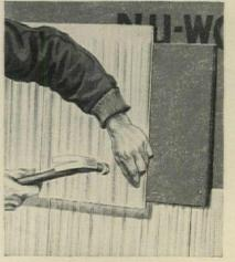
Now with 4' lengths of Nu-Wood shingle backer, three stud spaces can be covered at once to provide desired deep shadow lines of siding or shingles. Easy to apply. Saves money, adds extra insulation. basic to quality
