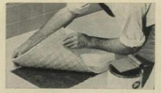
**Mesh-mounted ceramics** are new from American Olean. New backing holds tiles firmly in place, is flexible enough to handle easily yet stiff enough so it doesn't sag. Since mesh is on back, design is always visible and little cleanup is necessary. Strong bond will allow slight masonry movement without loss of grip. Perma-Bak may be used with any setting method, comes in all patterns in 1 9/16"—34" and 2 3/16"—1 1/16" series.
