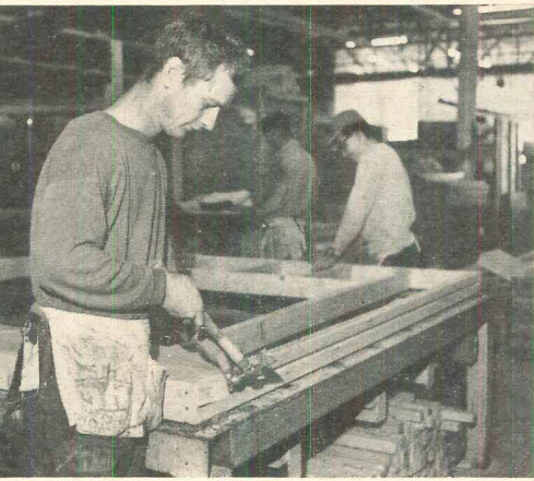
4 When panel frame is complete, it gets an IBM production ticket, which identifies it, shows it is for house No. 168,211. IBM numbers are key to ordering, manufacturing, accounting, and delivery.
