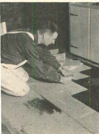
VERSABOND is spread with serrated trowel with continuous glue line.
