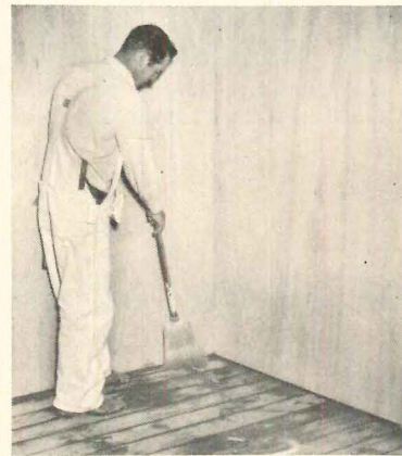
SUBFLOOR should be clean, dry, smooth, and well nailed.
