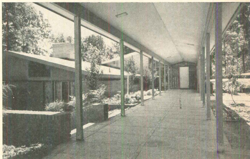
LENGTHY WALK leads from carport to entry. Steps (left) lead to dining terrace. This side of living wing has service rooms.
