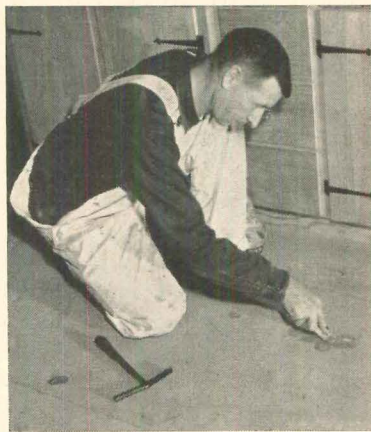
NAIL HEADS are set flush or counter-sunk, dents filled with compound.
