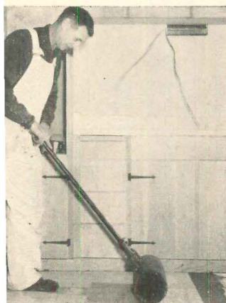
SMOOTHED FLOOR is rolled both directions with a 150-lb roller.
