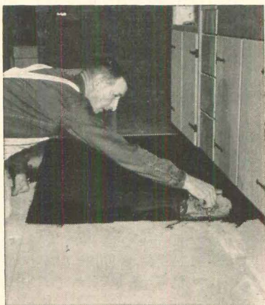
FLOOR TILES are laid with tight joints to meet manufacturer's specs.
