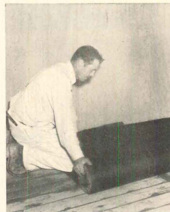
BUILDING PAPER may be used between subfloor and Versabord.
