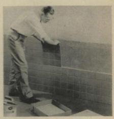
Tile on sheets goes up 12 at a time. New American Olean Master-Set tiles have a paper-thin backing that exposes 75% of the bonding area, yet holds tiles firmly enough to assure straight grout lines. Tile may be set with any accepted method; sheets need no soaking before being applied. Master-Set Tile comes in all standard glazed-tile sizes, in regular and crystalline glazes, and in some scored tile designs.
