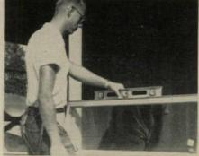
**AWNING IS LEVELED** to make sure the assembly will be true. Picture section will be nailed to the top of awning section.
