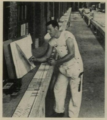
PATTERN STRIPS ARE LAID OUT on long table. Working from blueprint, carpenter tacks down blocks to show where framing members go.
