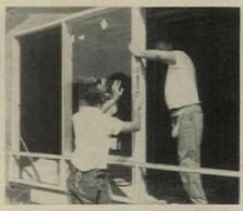
**CENTER PICTURE WINDOW** is installed after the three awning sections. Here it is leveled and plumbed before being nailed.
