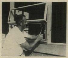
**WINDOW IS NAILED** through prepunched holes in aluminum frame. (See also drawing.) Aluminum strip will cover nail heads.
