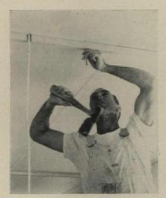
NAILING STRIPS 1" x 1½" on ceiling, floor, and sidewalls locate and hold partition. Wiring leads are dropped through ceiling, sandwiched between wallboard faces.
