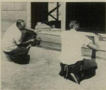
**BOARD IS NAILED** along base line as a straightedge on which the awning section can be rested before it is nailed in place.
