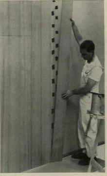
Thin redwood paneling gives a low-cost natural wood wall. La Honda panels are only 3/8" thick, 4", 6", or 8" wide in 8' lengths. Edges are t&g. Panels may be nailed or glued (above) to walls. One side of each panel is smooth milled, the other is resawn to give a choice of textures. Kiln-dried panels come in dust-tight cartons. One carton of 8" panels will cover up to 78 sq ft. Price: about 25¢ a sq ft.
