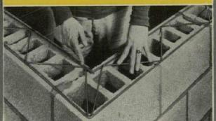
Insist on genuine Dur-O-waL for crack-free masonry walls with a backbone of steel
