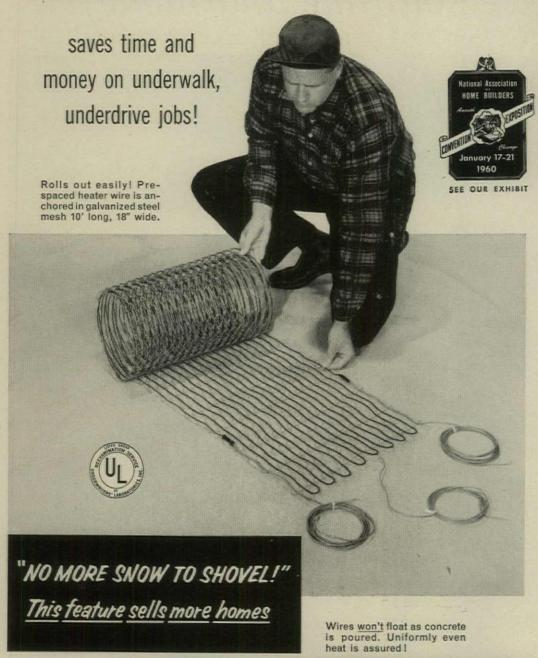
SNO-MELTER, designed for 42 watts per square foot, puts a practical price on snow-free walks, tire tracks for the drive! Heater wire has pre-assembled lead wires and ground, "Roll-out" installation saves time, cuts cost. Write for full facts!
