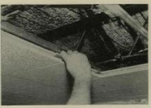
Fireproof acoustics are provided by Armstrong's Acoustical Fire Guard. Hung in mechanical suspension, these 5%" and 34" tile give up to four-hour fire ratings, have noise reduction coefficients of .70. Tiles are factory finished in fissured or random patterns. Light reflectance is over 78%.
