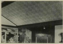
Decorated silent ceiling is new from Kaiser. Material is pinhole perforated Firtex on which a choice of six pastel colors have been printed. Ceilings come in all standard sizes with fir-lock or butt joints for stapling or gluing. Ceiling absorbs up to 70% of noise striking it manufacturer claims.
