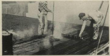
FOR WEATHER PROTECTION. Weatherproof with a Reinforced Monolithic Built-Up Roof of porous Fiberglas Perma Ply\*. Successive applications of hot asphalt penetrate the Fiberglas mat and are bonded together into a one-piece, long-lasting roof.
