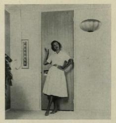
Ceiling-high doors that cut cost of overhead framing are now being made by Simpson Logging. Hollow-core flush doors are made 7'11" long and may be end-trimmed as much as 3" at the top to allow fitting. A 5½" lock rail extends the full width so lock can be set back as far as you wish. Doors are available in ribbon and rotary Lauan, rotary birch, and hard-board.
