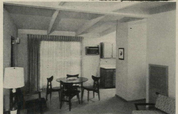
INTERIOR of finished house shows how panelized exposed-beam ceiling looks. When roof is all in place, ceiling and framing is spray-painted. Larsen is using this roof system in his 6,000-house Clair-Mel community in Tampa (H&H, Nov '58, p 60). /END
