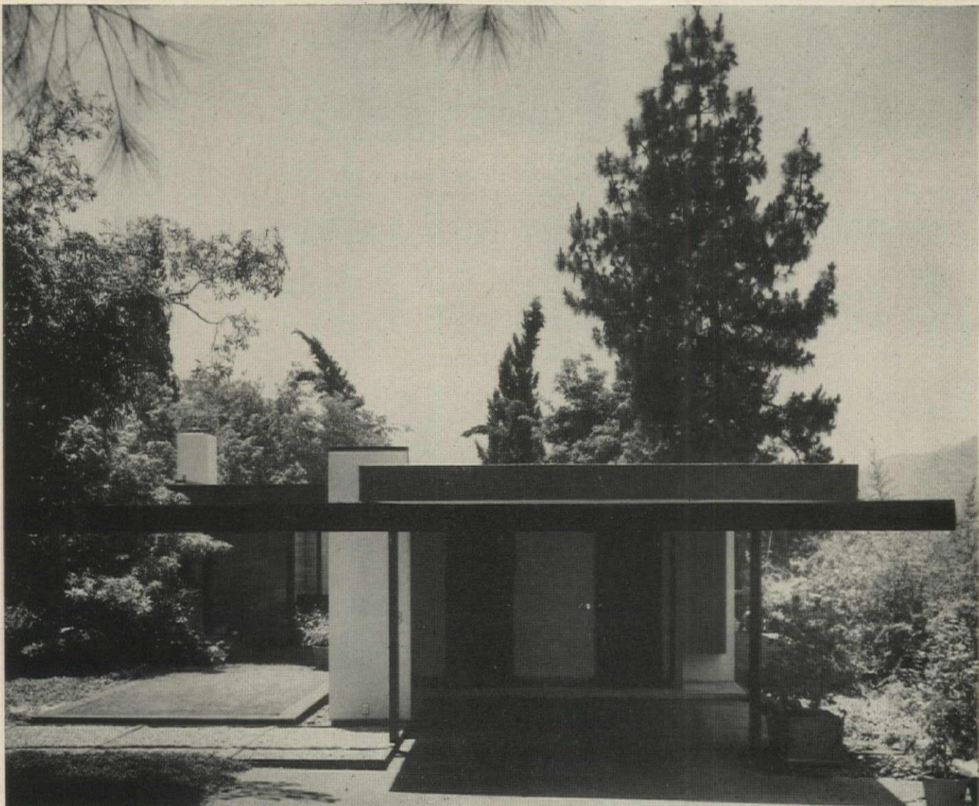
CARPORT ENTRANCE gets interest from wide overhang and long trellis, carefully laid-out grass and gravel rectangles, left.
