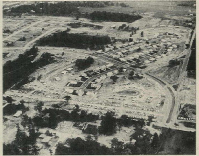
AFTER houses are up, La Bonte stages miniature parade of homes, at which visitors see variety of models by his eight builder clients.
