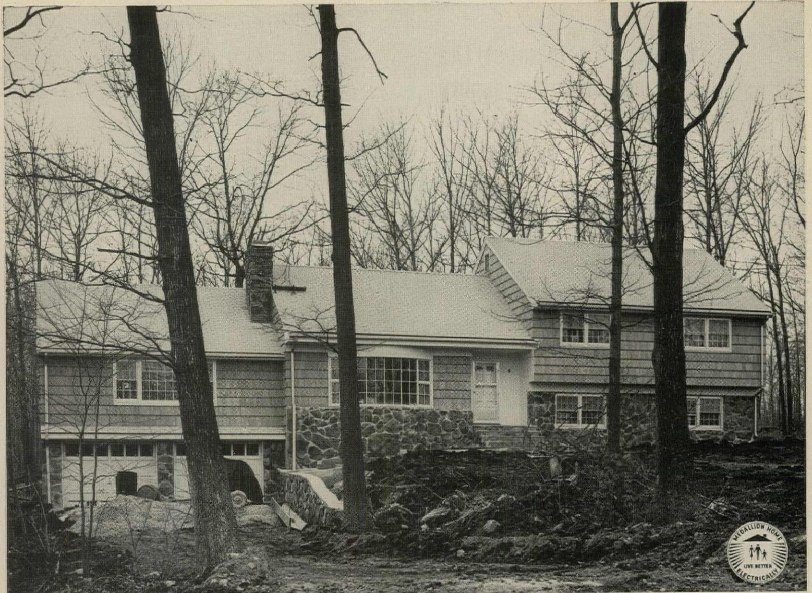
General Electric Remote-Control Wiring controls "Light for Living" in this Gold Medallion Home at Rock Ridge in Fairfield, Conn.
