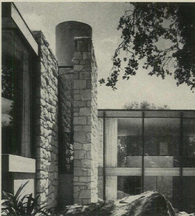
FIREPLACE CHIMNEY is set between two-story planes of masonry. Narrow glass sheet runs full wall height, so fire can be seen outside.
