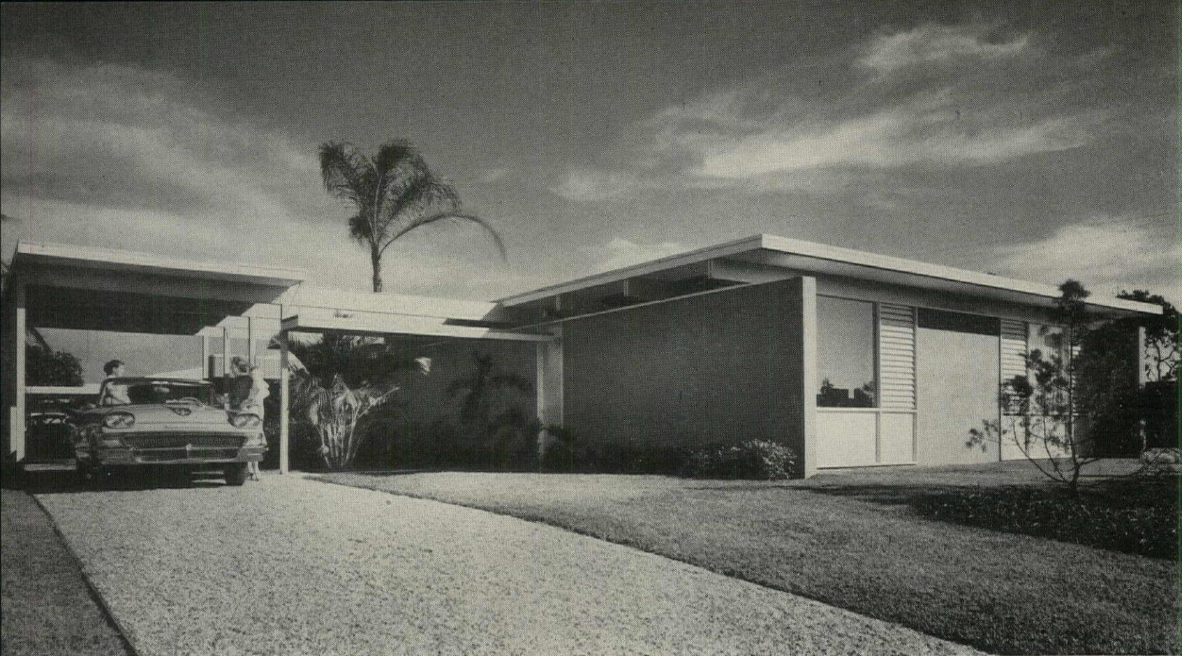
House is sited sideways to street. Front wall, facing carport, is blank except for entry and fixed glass set between the roof beams.
