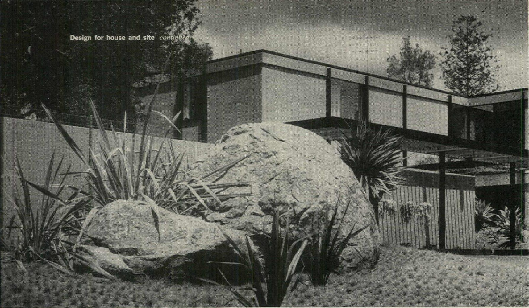
APPROACH TO HOUSE is from motor court through entrance court. Freestanding wall, left, hides lawn. Trellis gives walk a semi-shaded effect.
