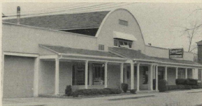
SOUTHPORT LUMBER CO has dressed up the front of the yard over the years, but the original building is still the core of the expanded building. Other units have been added at rear.
