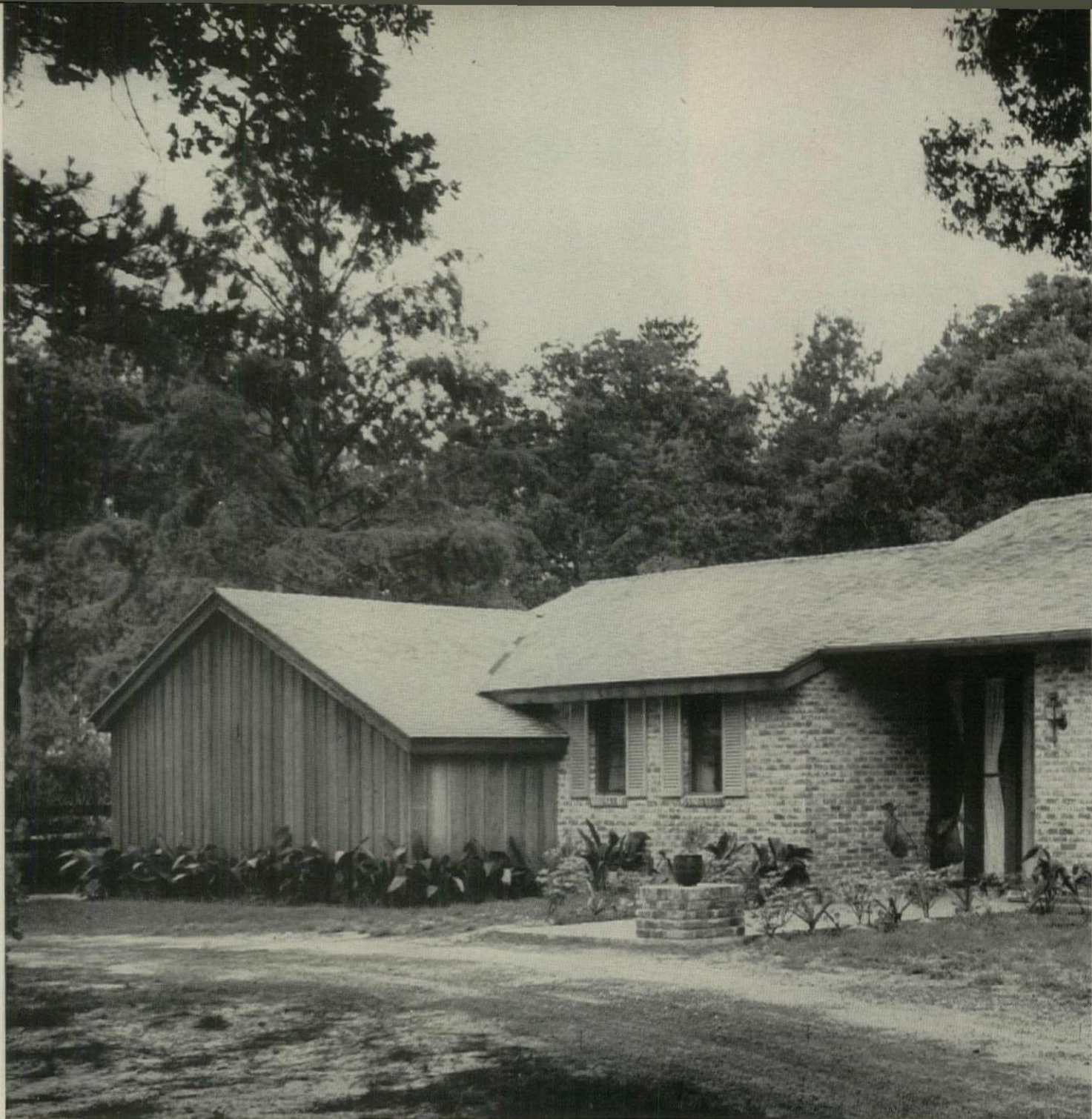
NATURAL MATERIALS OUTSIDE HOUSE —soft-colored brick, cedar shingles, and board-and-batten siding—create patterns and shadows.
