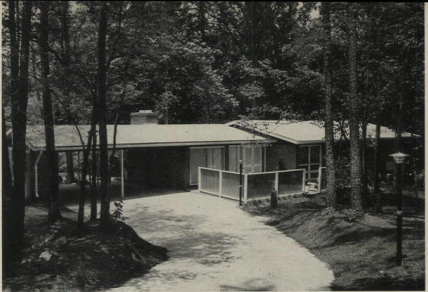
Entrance is set off by fenced terrace. Living room sweeps out to form carport. Family room, bedrooms are at right.
