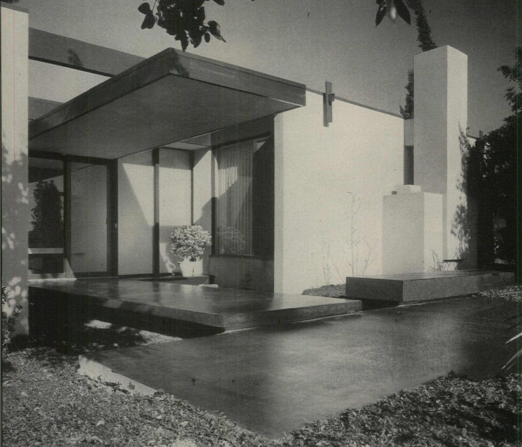
MAIN ENTRANCE gets dramatic emphasis from cantilevered overhang which covers entry court, sweeps out over walk.
